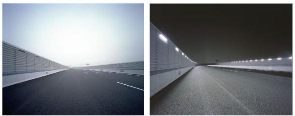
Source: Panasonic Eco-solutions (Project name: Shin Meishin Expressway Asuka IC- Nabeta IC in Japan) **Figure 6.2.9Noise Barrier with Lighting System in the handrail/noise barrier/view barrier**
