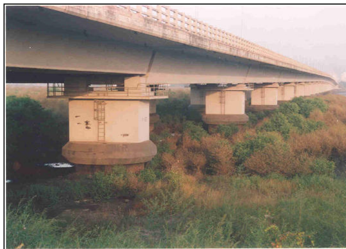
Figure 4.3 Airoli Creek Bridge
