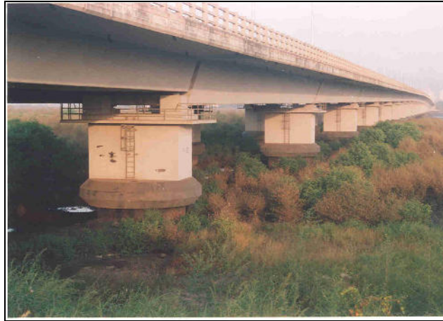
Airoli Creek Bridge
