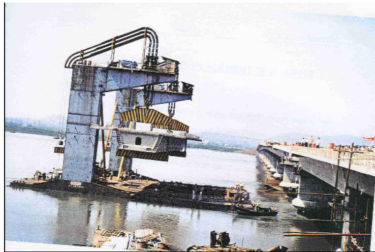
Figure 2.6 Girder Shifting during Launching
