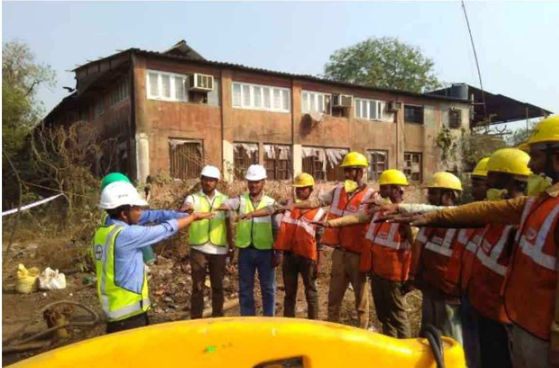
Package-1 Safety Pep Talk for workmen
