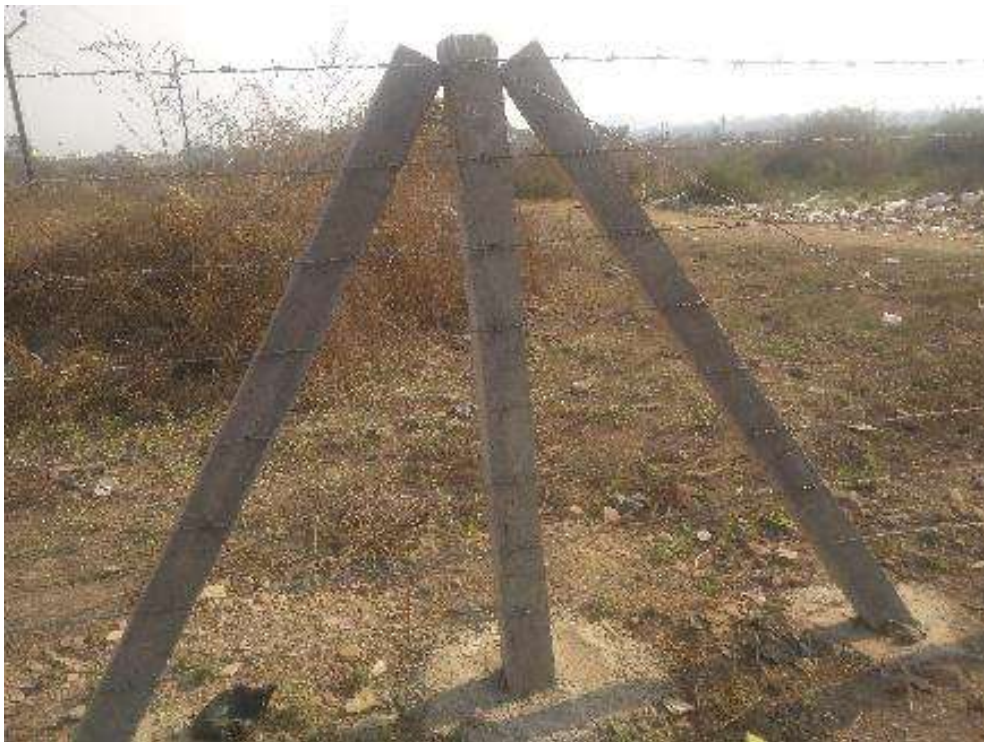
Package -2 Erections of RCC Poles in Mudflat at Interchange ROW.
