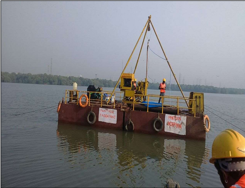
Package-1 GT Investigation in progress in Intertidal Section at MP10-B
