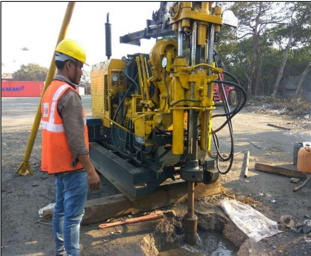
Package-1 GT Investigation in progress in Sewri Interchange at AP42
