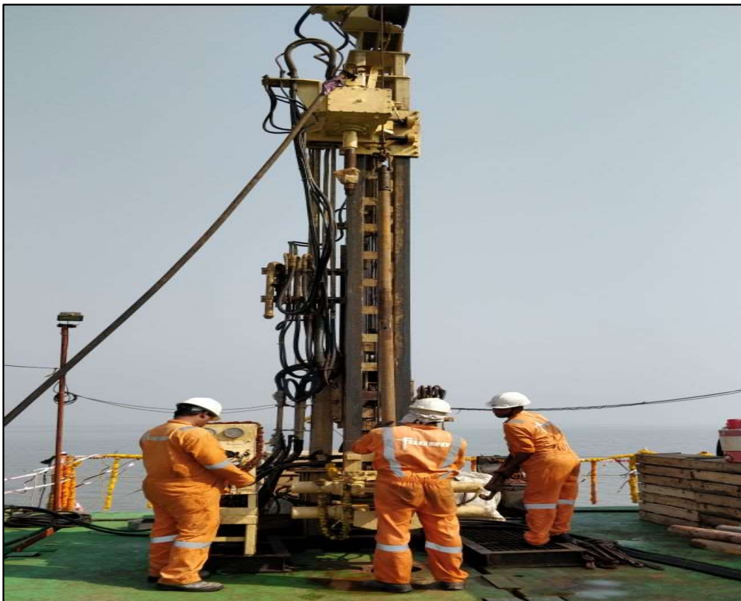
Package-1 GT Investigation in progress at Marine Section
