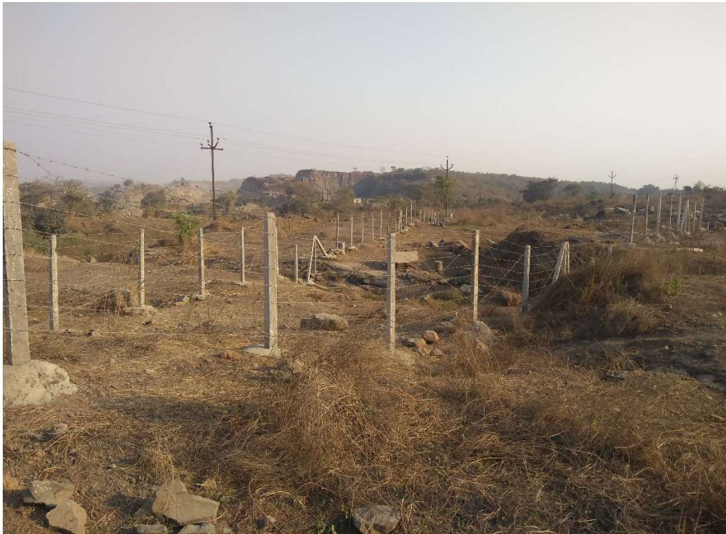
Package-2 casting yard (4.3 Ha)
