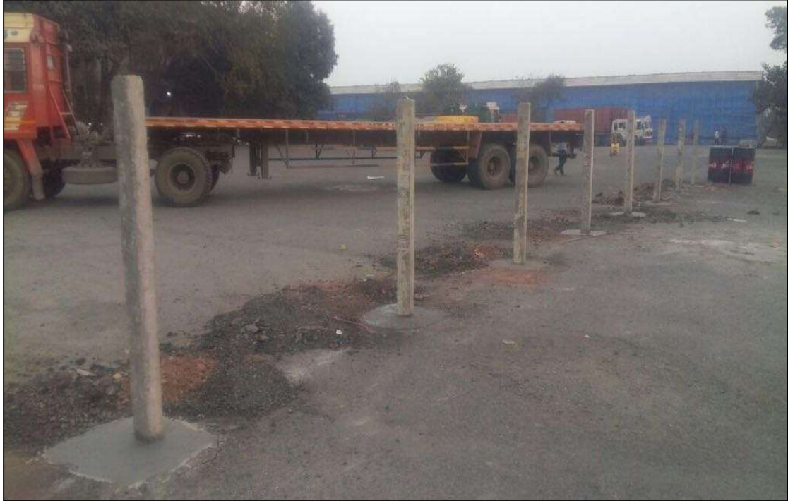
Package-1 Fencing work in progress in STP area at Sewri Interchange
