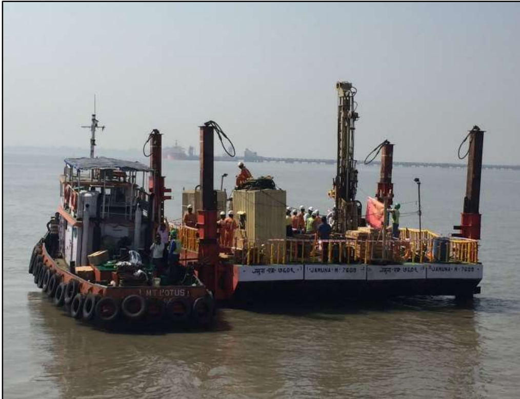
Package-1 Geotechnical investigation Works Start in Marine Area at MP 118-B
