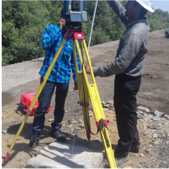
Photo 19: Survey Work (Control Point) On-going
