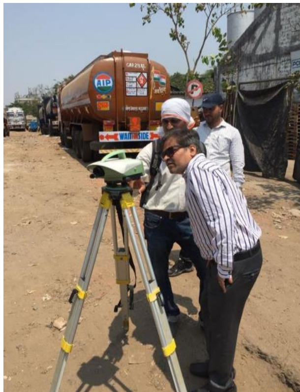
Photo 18: Survey Work (Control Point) On-going
