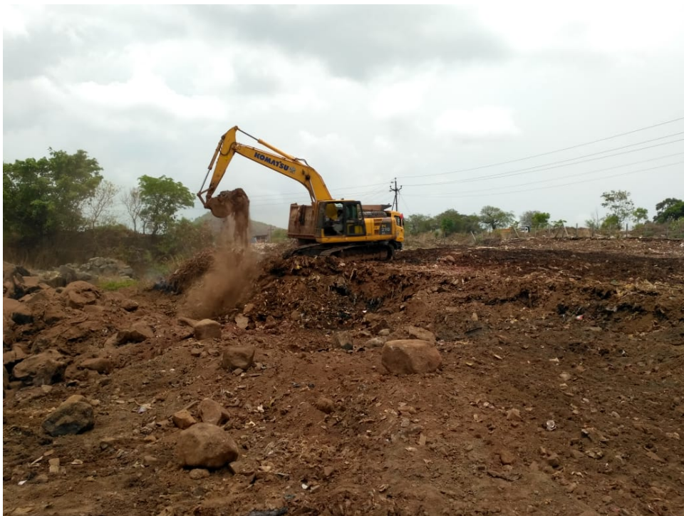
Photo 10: Excavation and ground levelling work for the Labor Camp in Progress
