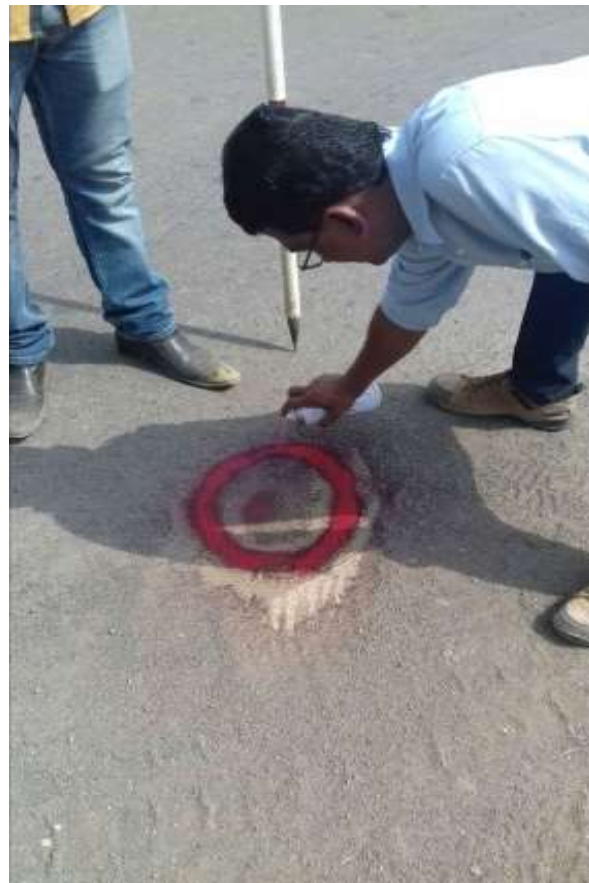
Photo 20: Centre Line Marking at Chainage 18+187
