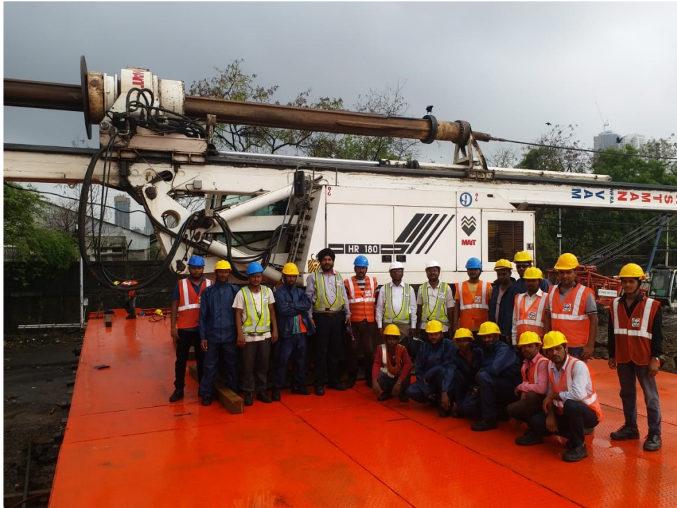
Photo 3: Temporary Access Bridge Piling Gantry Erection Completed at MP 1 Location
