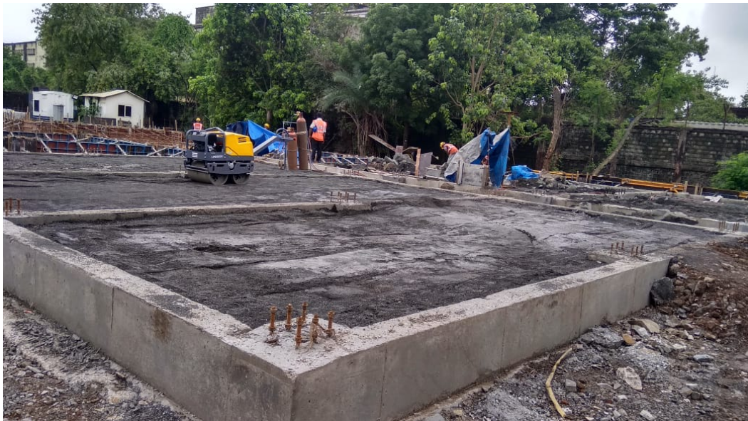
Photo 6: Project Office –Foundation Works at STP Yard completed
