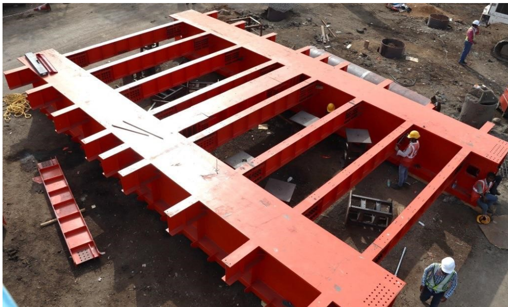
Photo 4: Girder 3-3X Fabrication Work in Progress
