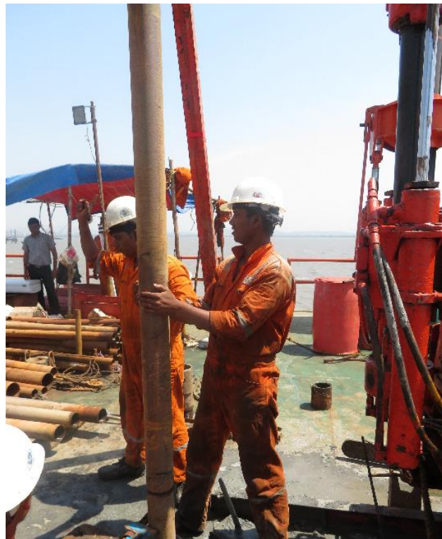
Photo 12: Geotechnical Investigation at P 157R
