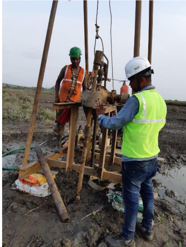
Photo 11: Geotechnical Investigation Works at Interchange
