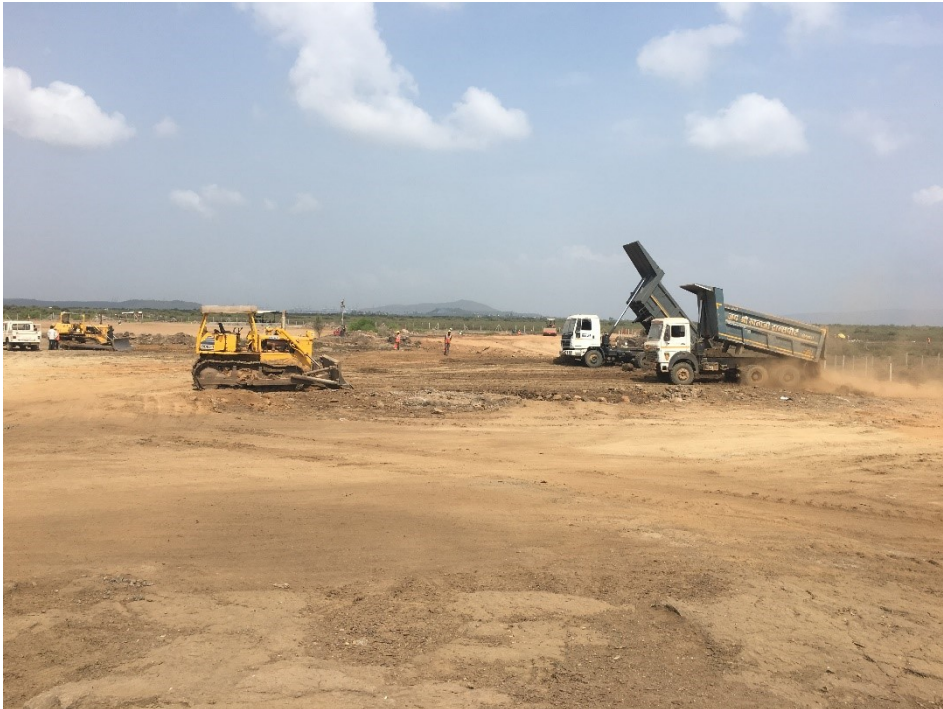
Photo 9: Excavation and ground levelling work in the Casting Yard
