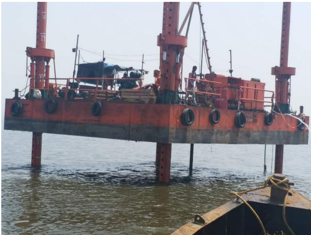
Photo 14: Jack Up at P 163R Location
