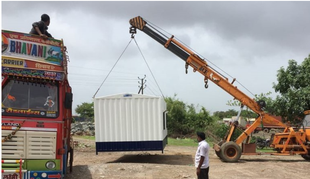
Photo 17: Site office container placing and set up works ongoing
