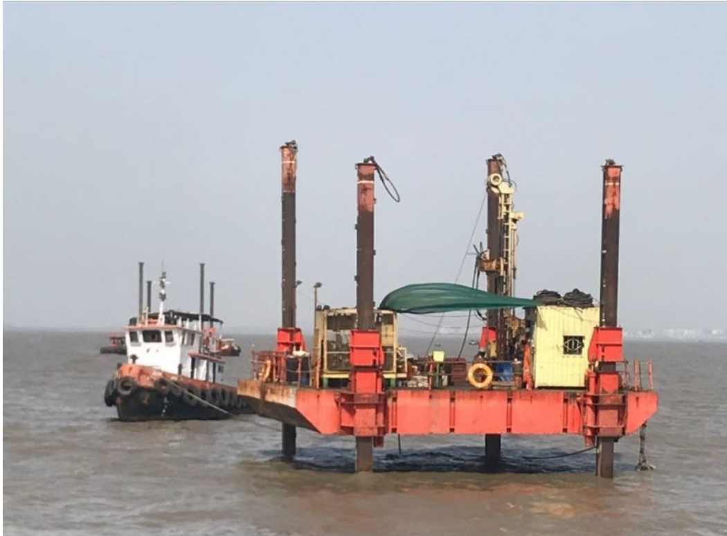
Photo 7: Marine GTI works at MP 146A in progress
