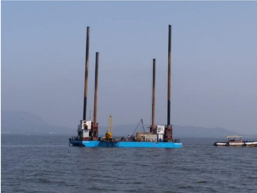
Photo 13: Jack Up at P 152L Location
