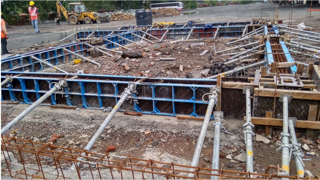
Photo 5: Project Office – Plinth Beam Formworks at STP Yard in progress
