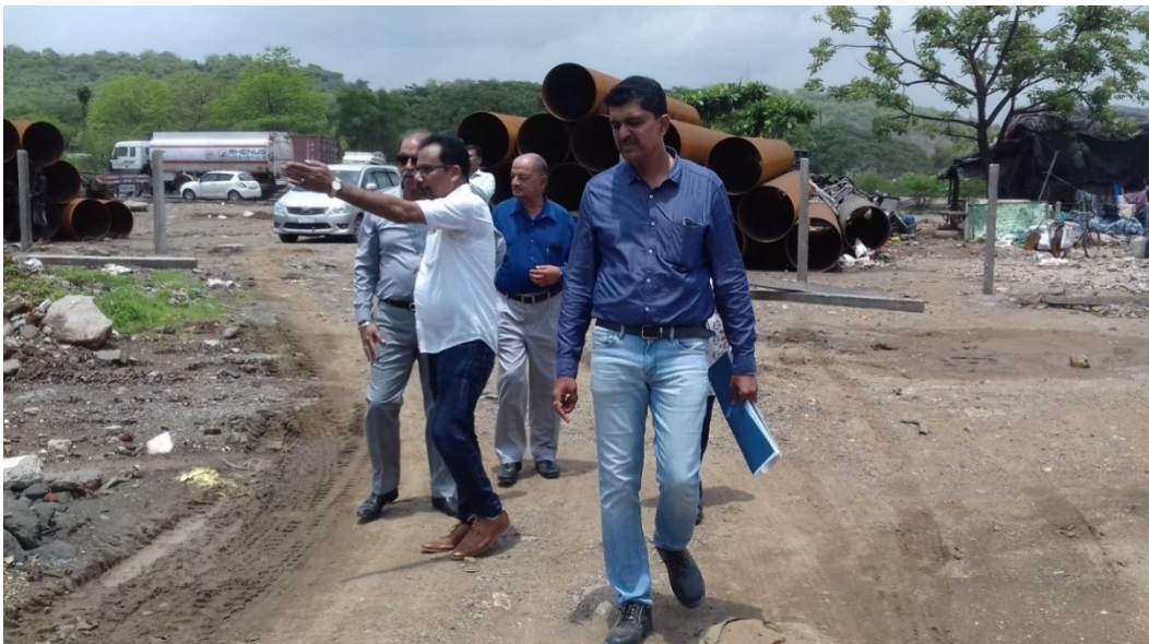
Photo 16: Joint Inspection by the GC and Contractor dated 19.6.2018
