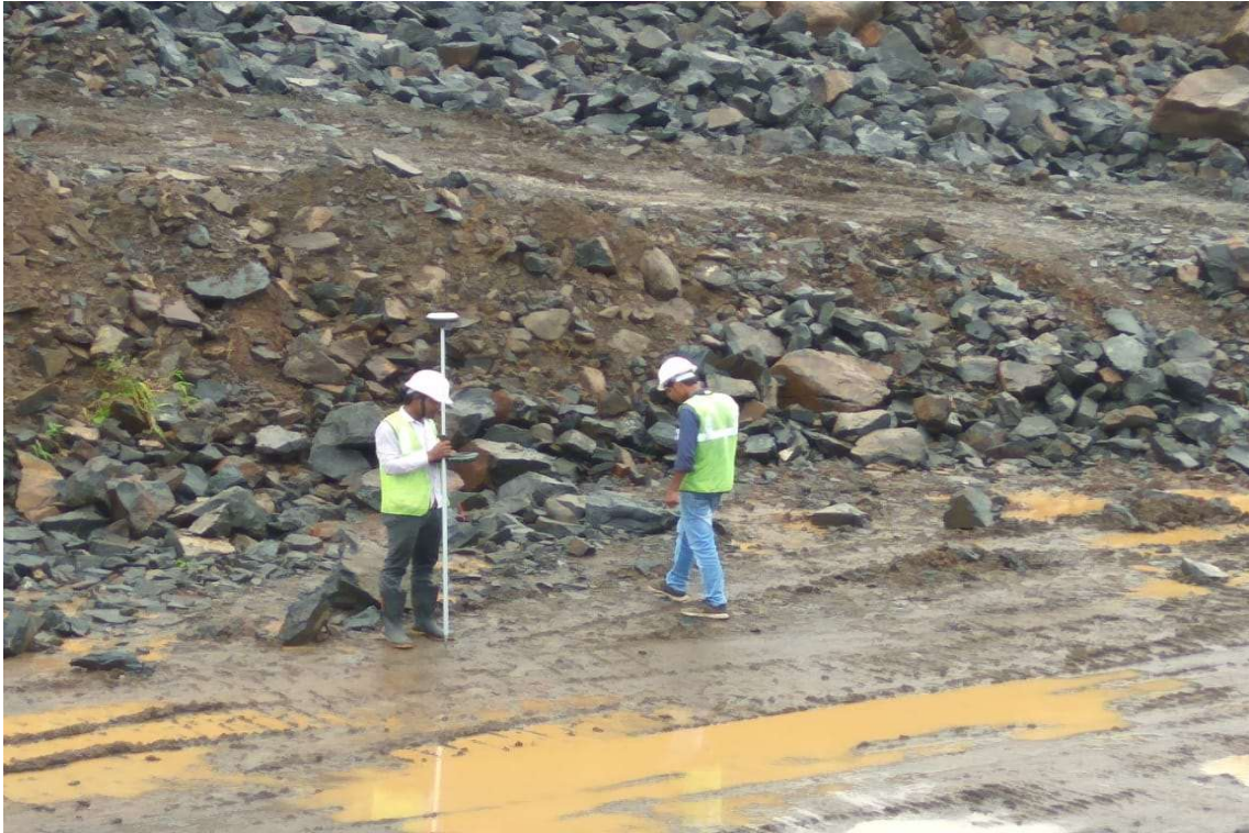
Photo No. 21: Topographical Survey Works at Chainage 19+700 in progress
