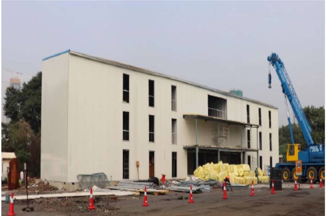
Photo No. 9: Site Office Construction Works in progress
