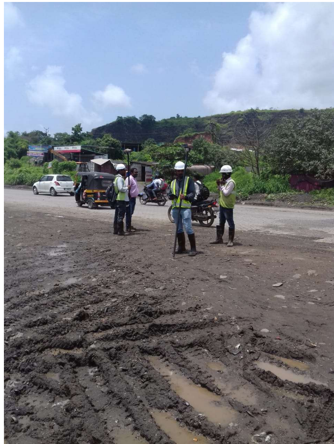
Photo No. 22: Survey Works at Chainage 20+200 in progress
