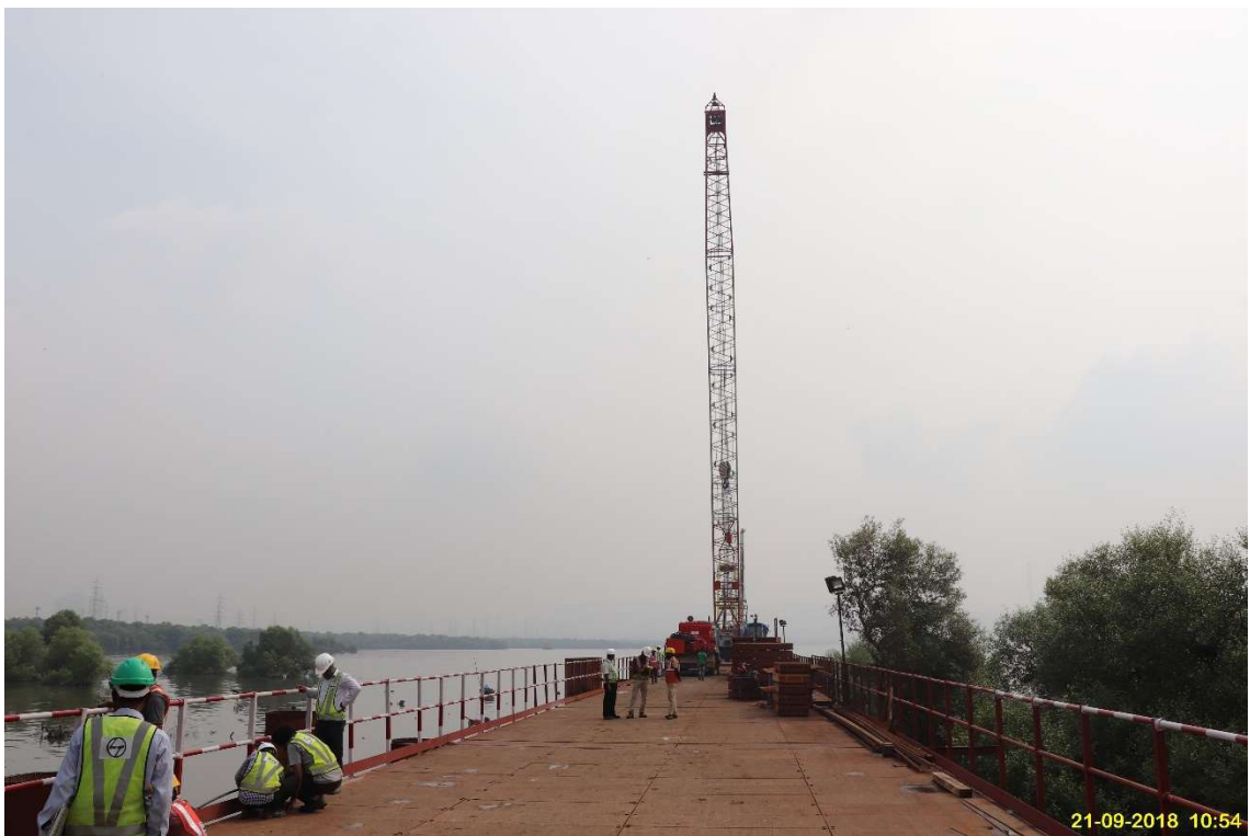
Photo No. 6: Temporary Access Bridge (TAB) Erection Works in progress
