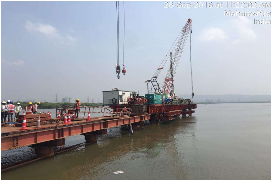
Photo No. 7: Temporary Access Bridge (TAB) Erection Works in progress
