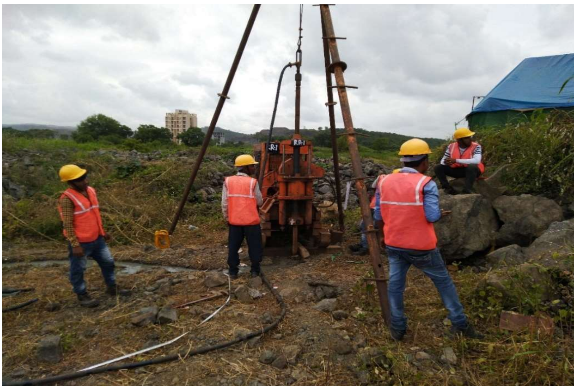
Photo No. 20: GTI work at Chainage 18+487 in progress
