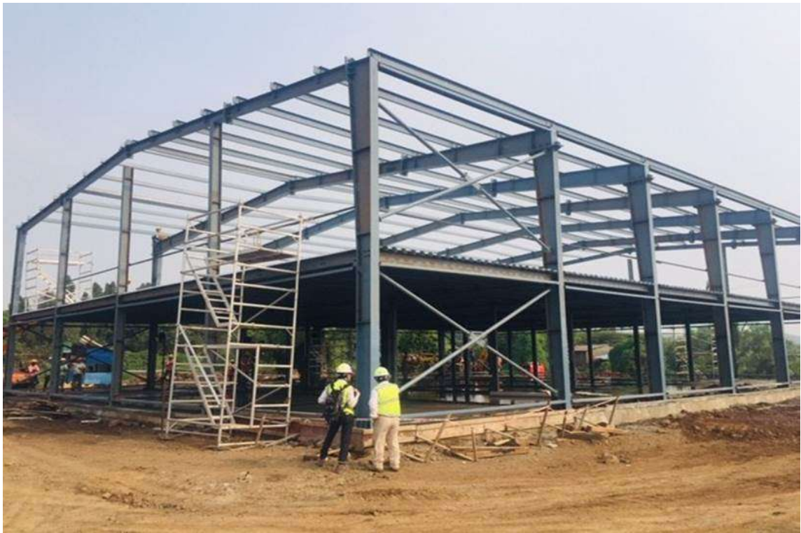
Photo No. 13: Project Site Office Construction Works in progress
