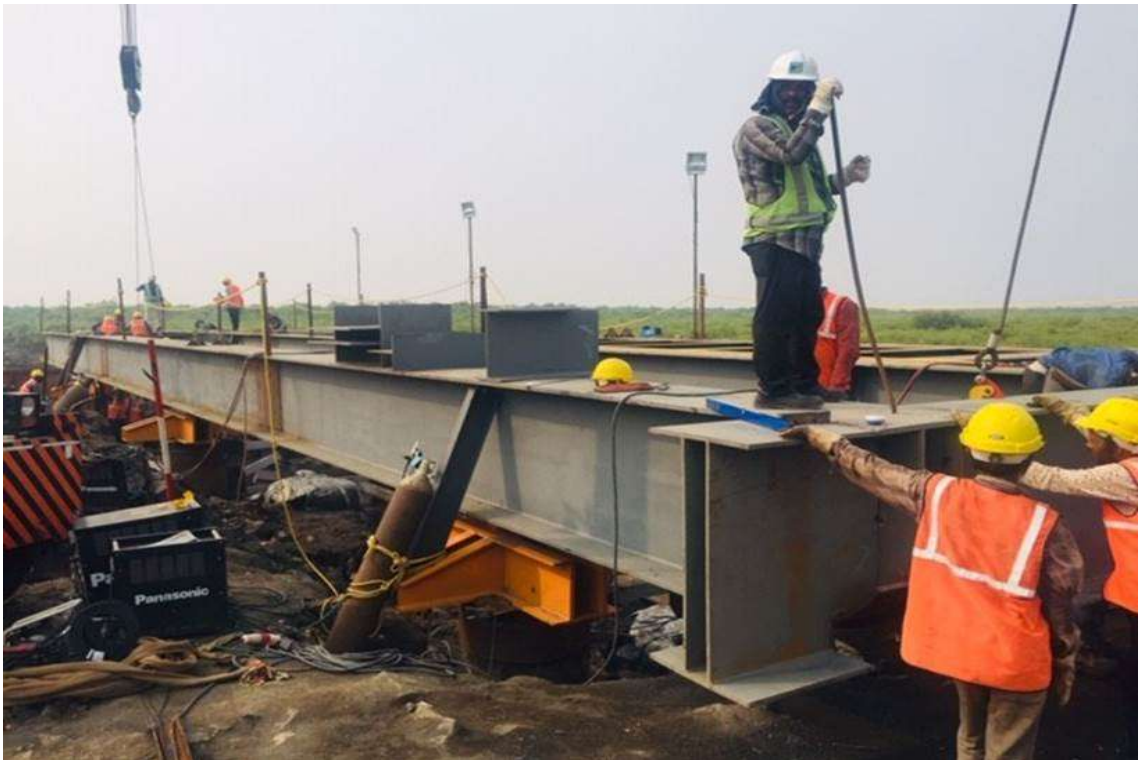
Photo No. 11: Temporary Access Bridge (TAB) Erection works in progress
