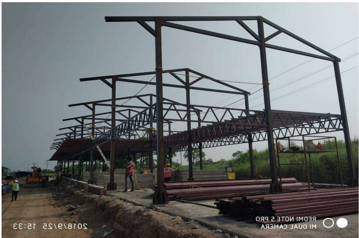
Photo No. 14: Labour Colony Construction Works in progress
