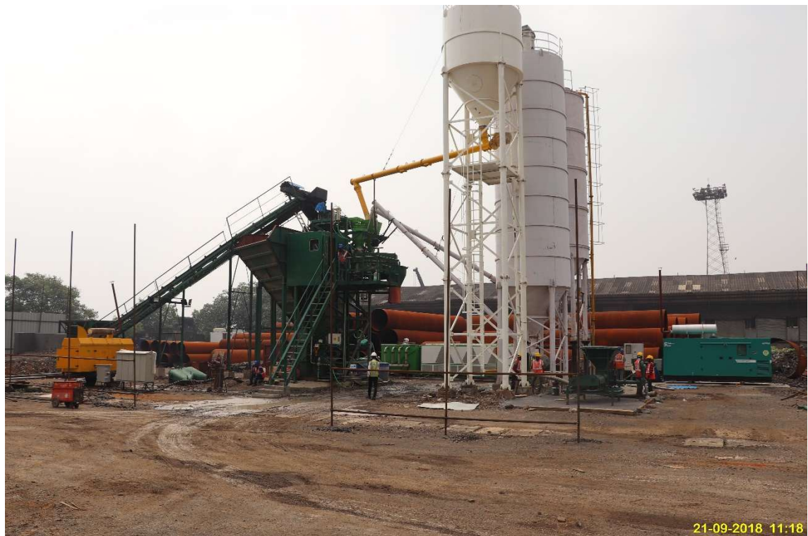
Photo No. 8: Concrete Batching Plant Installation works in progress
