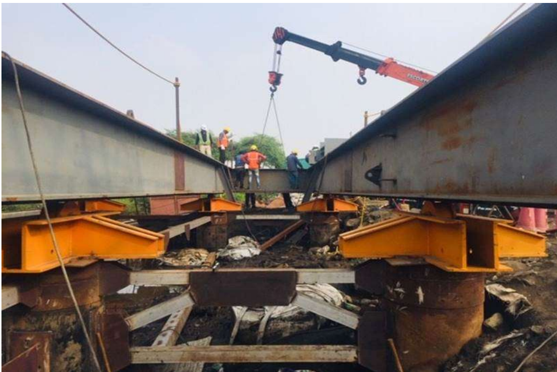
Photo No. 12: Temporary Access Bridge (TAB) Erection works in progress
