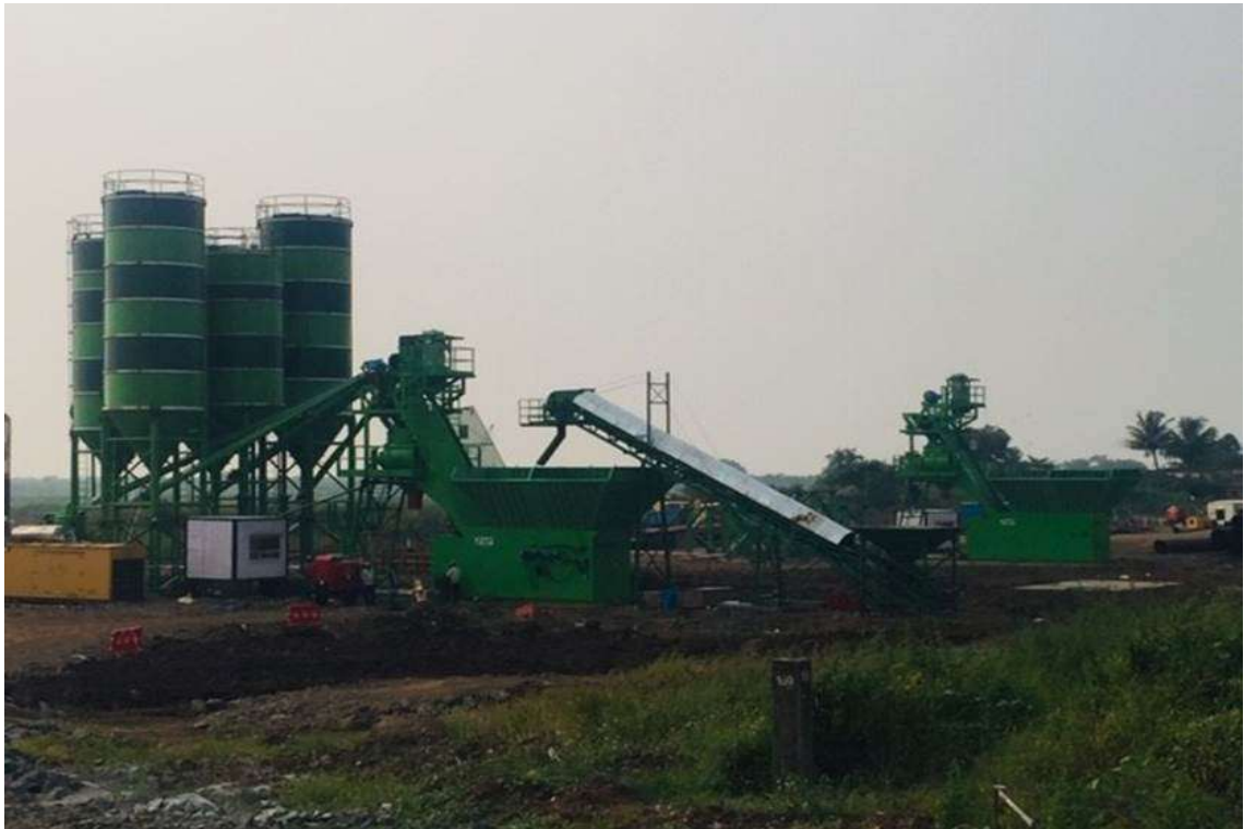
Photo No. 15: Concrete Batching Plant Erection Works in progress
