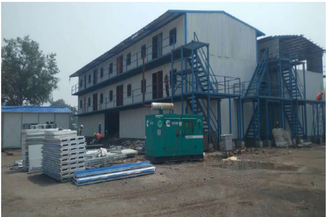
Photo No. 10: Labour Colony Construction Works in progress
