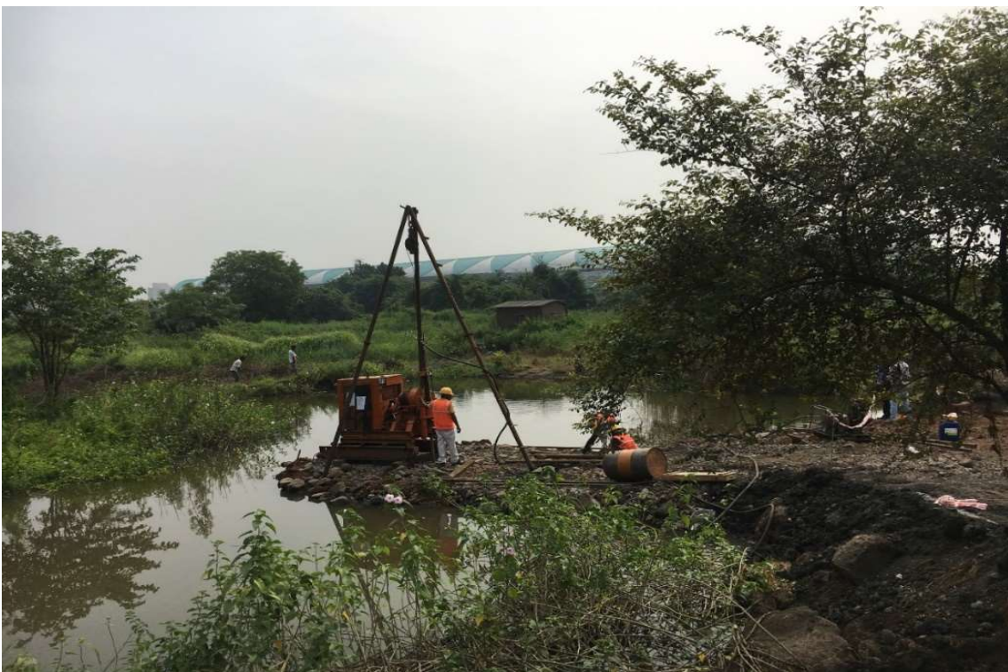
Photo No. 18: GTI work at Chainage 18+230 in progress
