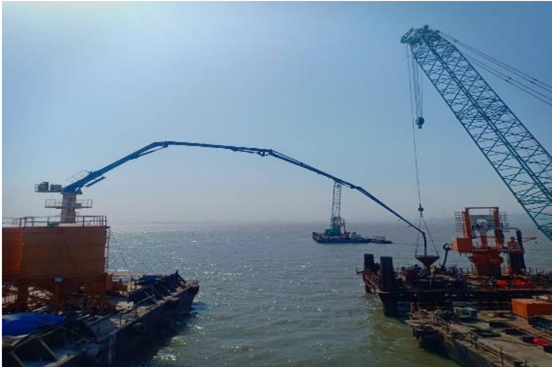
Photo No. 17: Pile Concreting at MP 162/02 RHS location in progress
