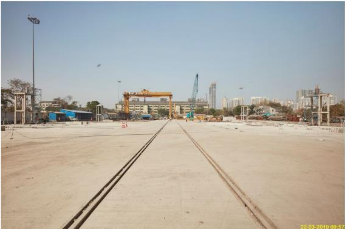
Photo No. 14: Casting Yard Development
