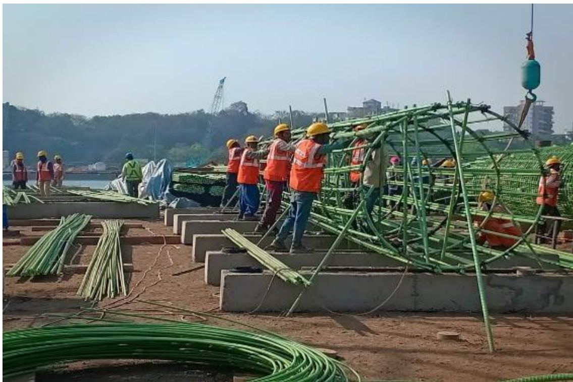
Photo No. 20: Pile Reinforcement works at Belapur Jetty location in progress
