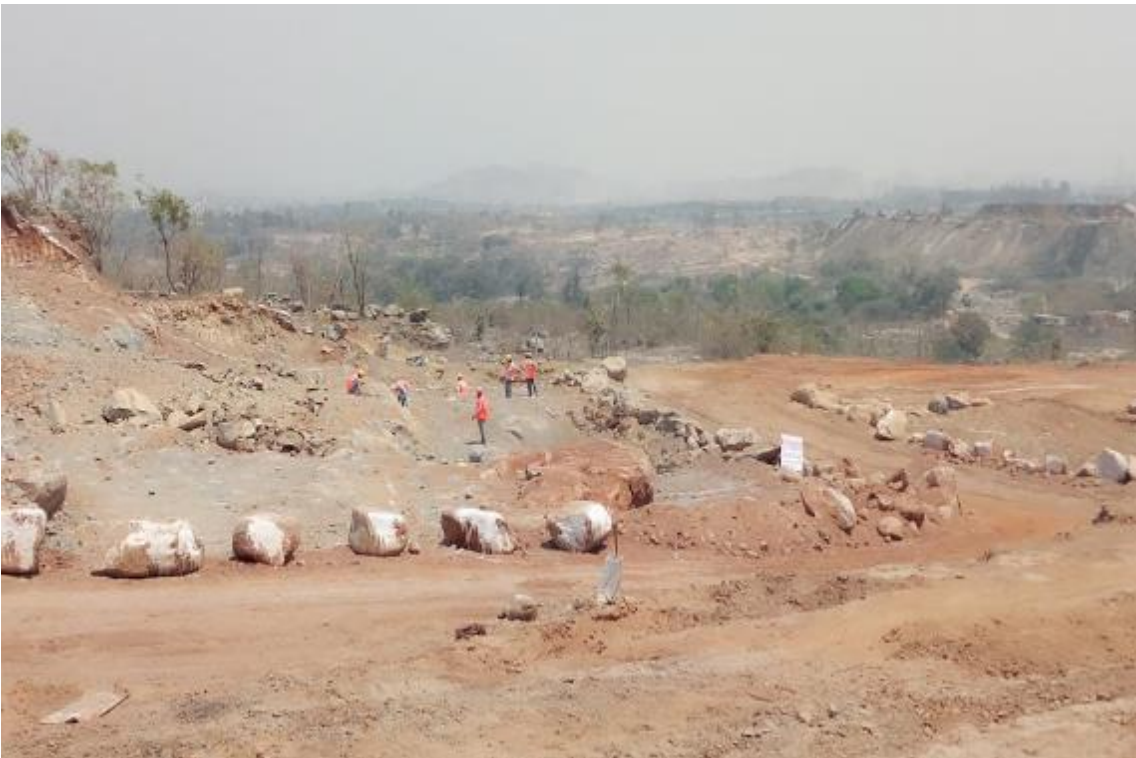
Photo No. 32: Blasting (at Grade) at CH 19+720 to CH 19+920 in progress
