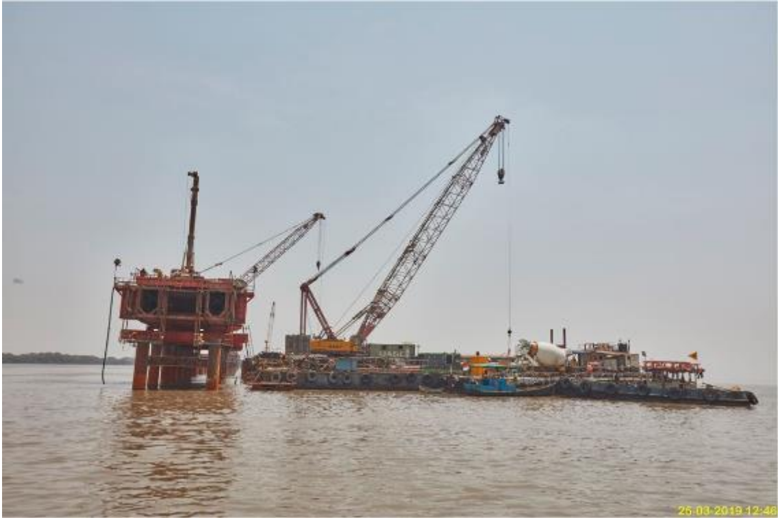
Photo No. 5: TAB Concreting from PG-3 in progress
