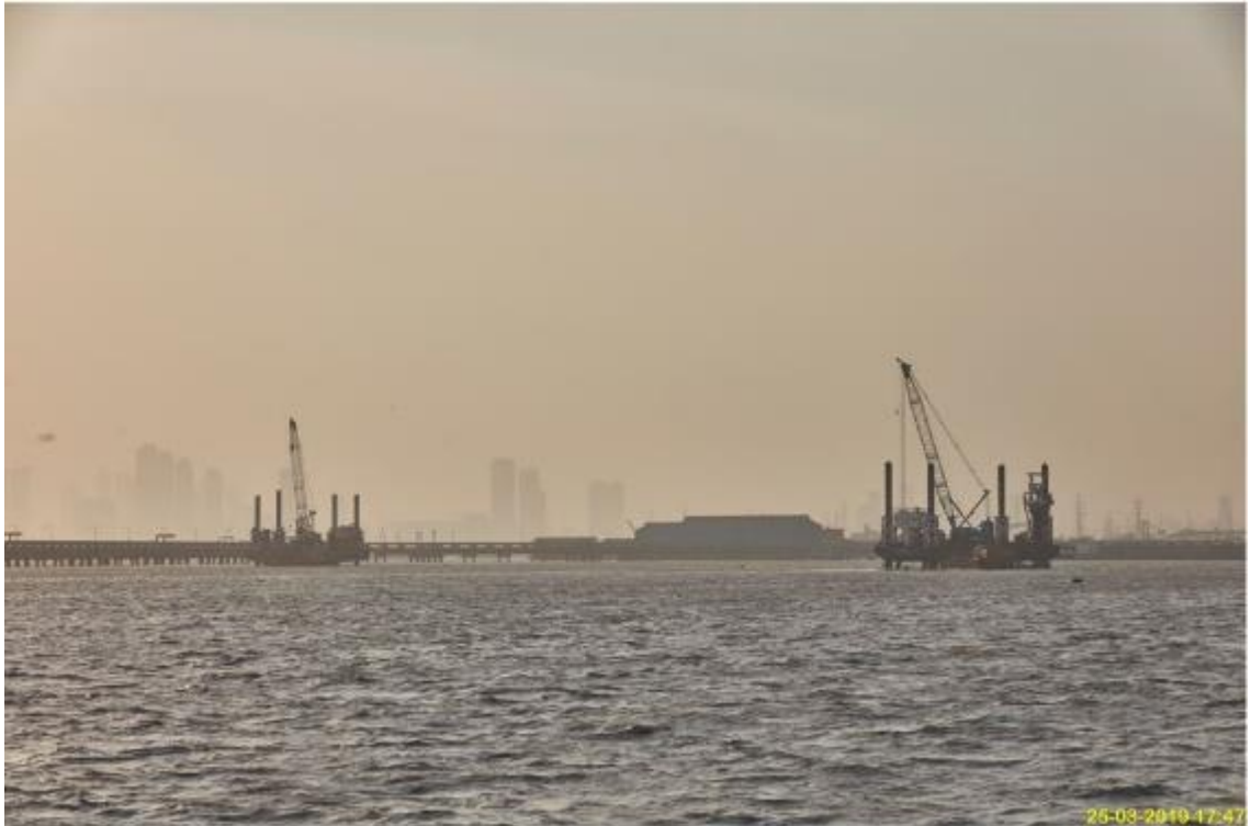
Photo No. 11: Piling at MP89 location in progress
