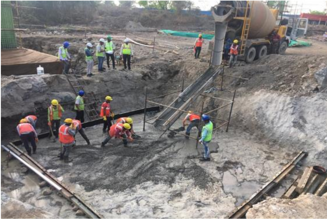
Photo No. 27: PCC Works at LMP 268 in progress
