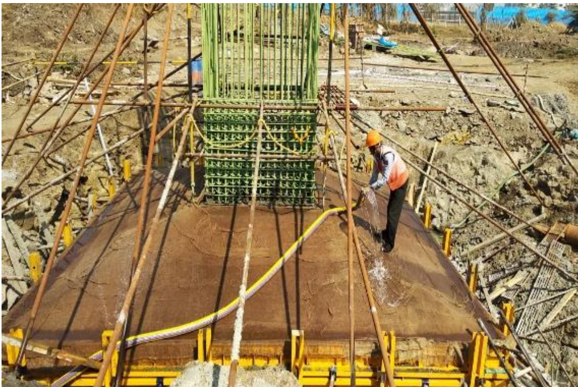
Photo No. 26: Curing Works for RMP 268 Foundation in progress
