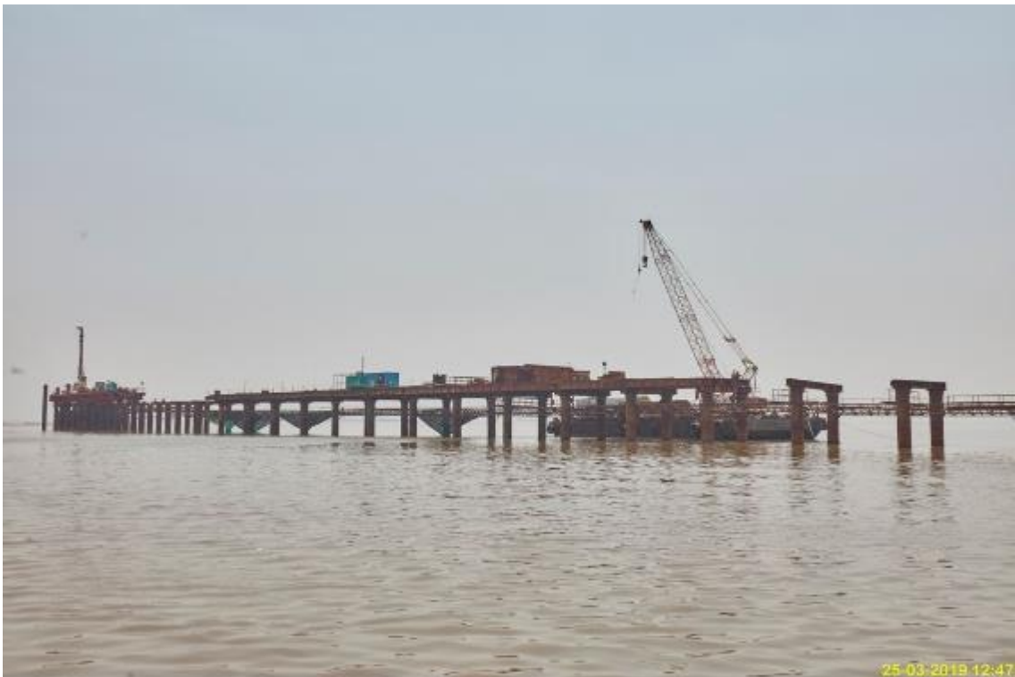
Photo No. 6: TAB Deck Erection at MP43 location in progress
