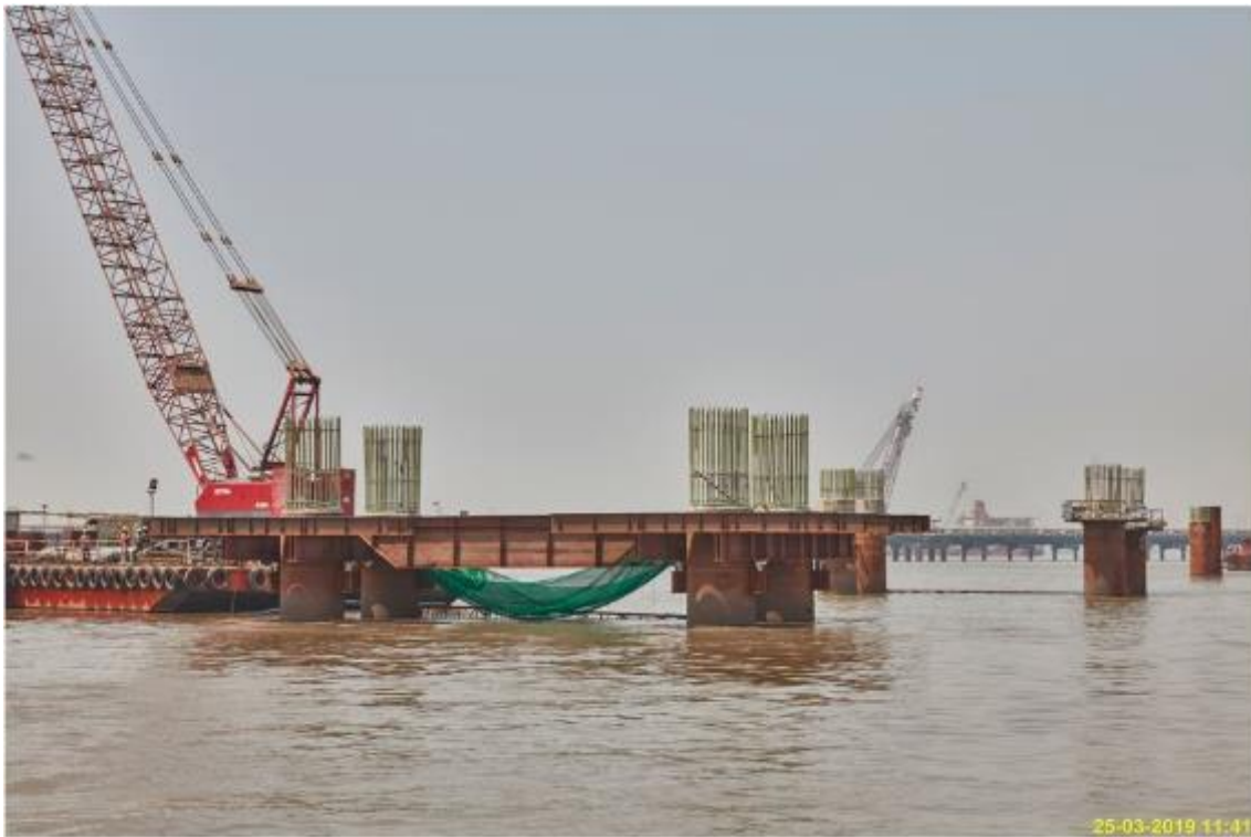
Photo No. 8: Pile Cap works at MP94 location in progress
