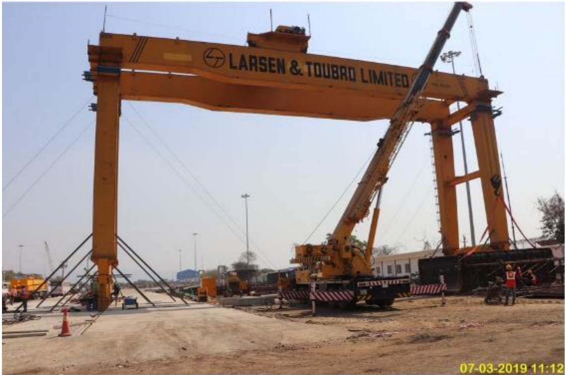
Photo No. 13: 175 T Gantry Crane Erection & Commissioning Completed
