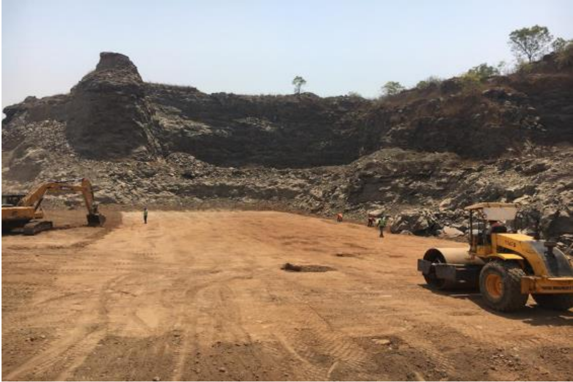
Photo No. 31: Embankment work at CH 18+990 to CH 19+050 in progress
