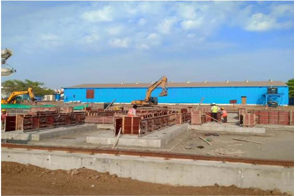
Photo No. 21: Mould Foundation-wall formwork at Casting Yard Bay-1 in progress
