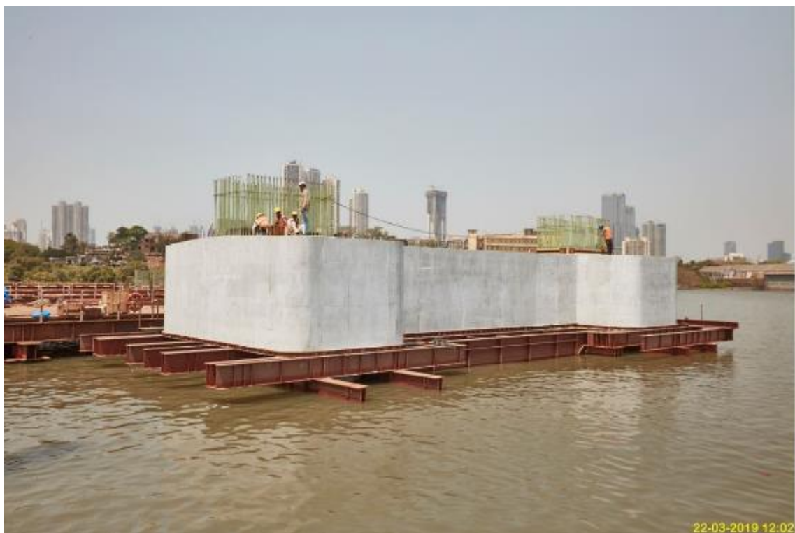
Photo No. 2: Pile Cap at MP7 after De-shuttering
