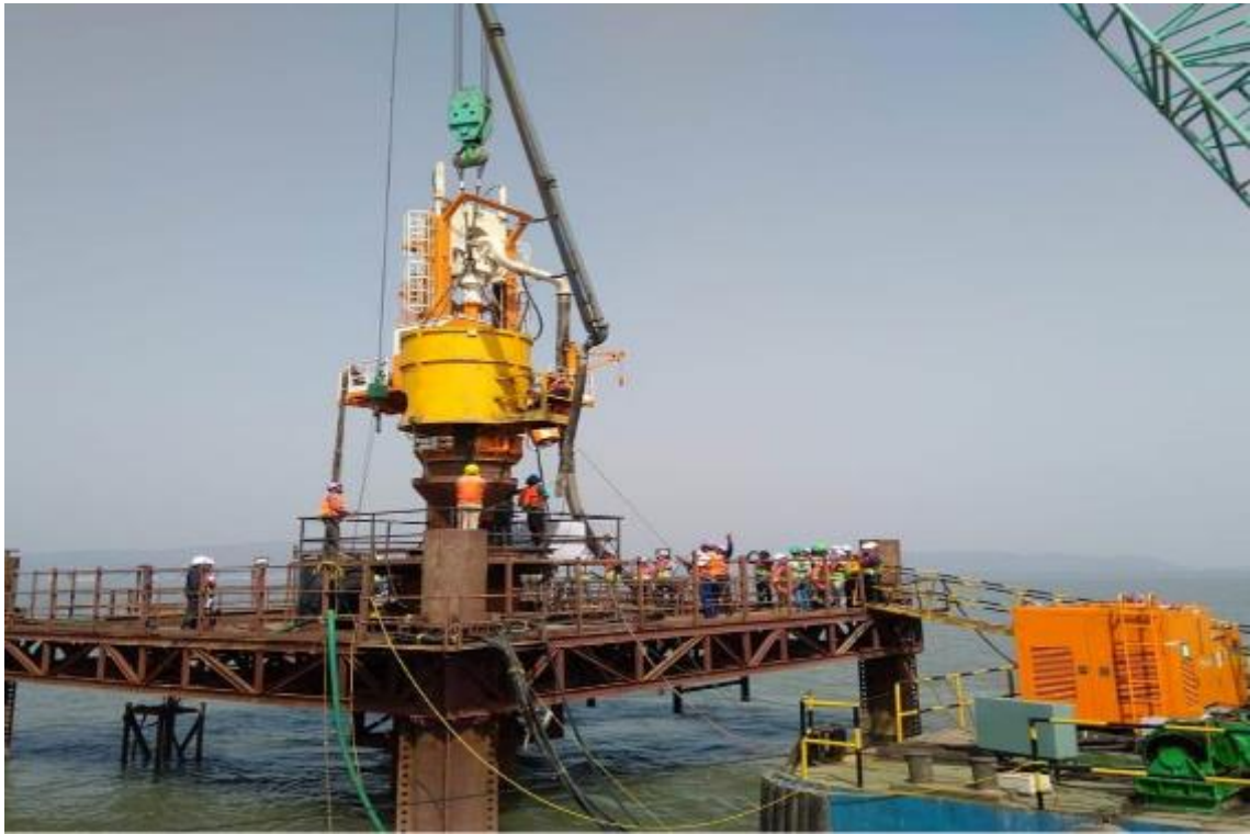
Photo No. 15: Pile Boring works at MP 165/03 RHS location in progress
