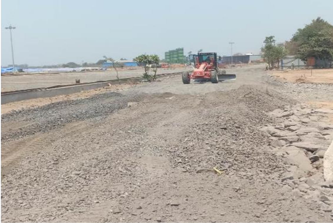
Photo No. 23: Internal Road works at Casting Yard in progress
