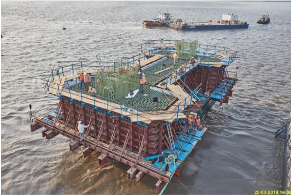
Photo No. 7: Pile Cap works at MP95 location in progress
