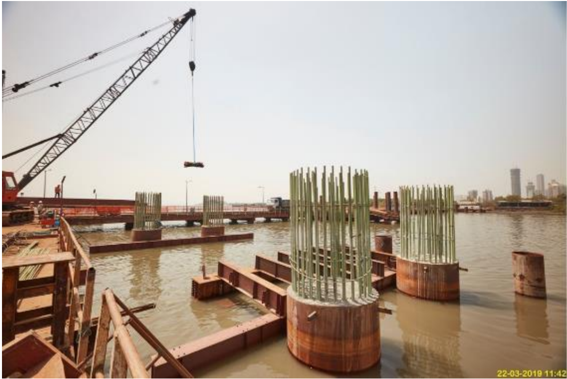
Photo No. 3: Pile Cap works at MP6 location in progress
