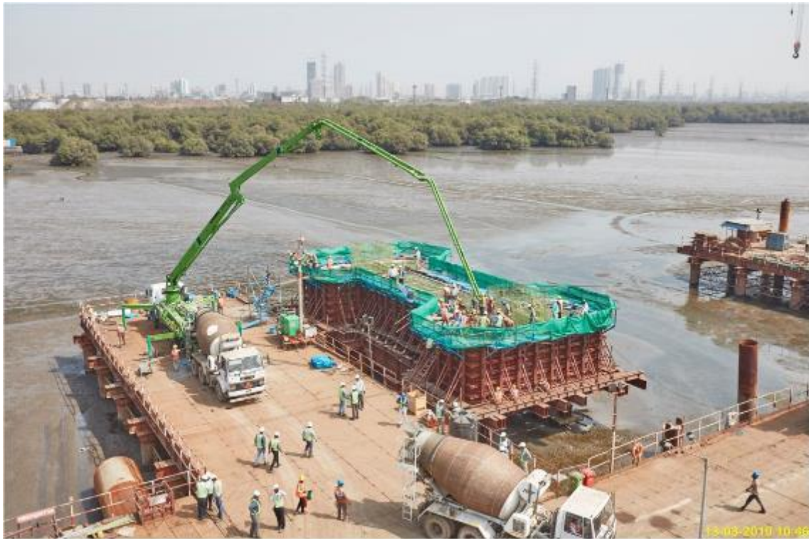
Photo No. 1: Pile Cap Concrete at MP7 location in progress
