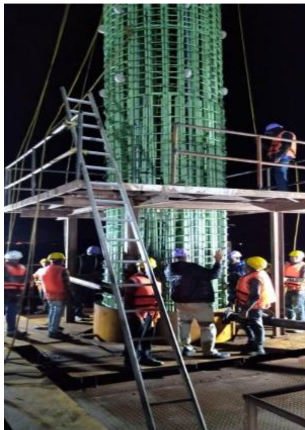
Photo No. 16: Reinforcement Cage installation at MP 162/04 location RHS in progress
