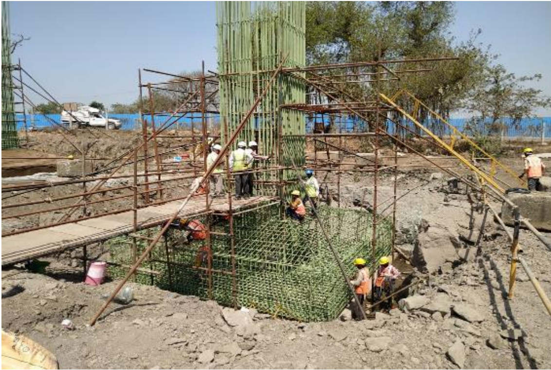
Photo No. 25: Reinforcement Works at LMP 267 Foundation in progress
