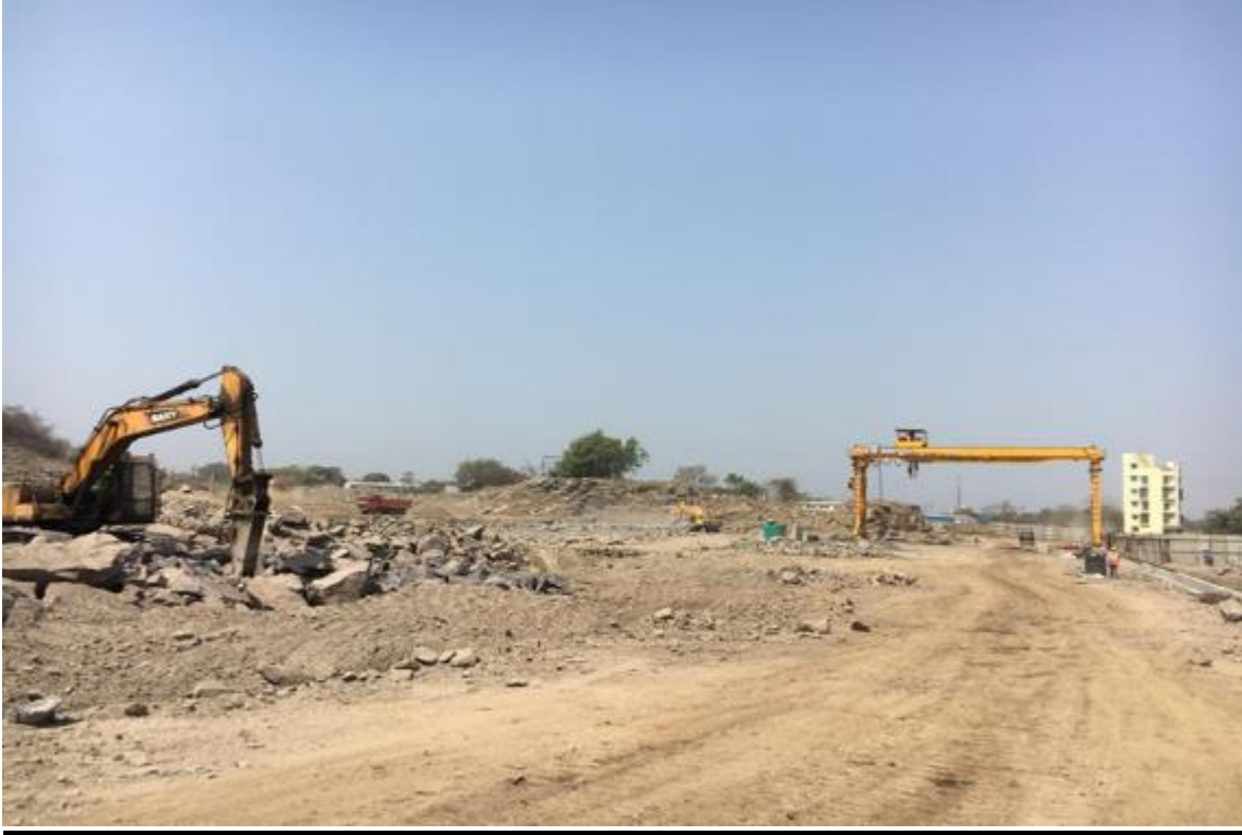
Photo No. 29: Track beam work at Casting Yard in progress
