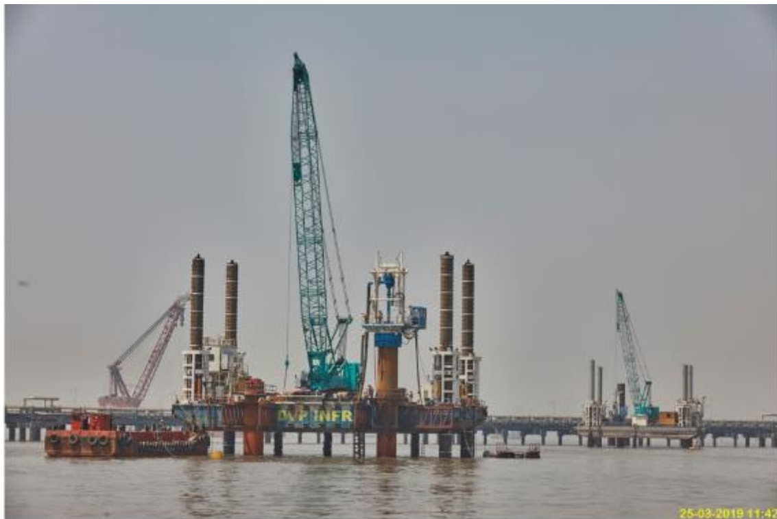
Photo No. 10: Piling Works at MP89 location in progress
