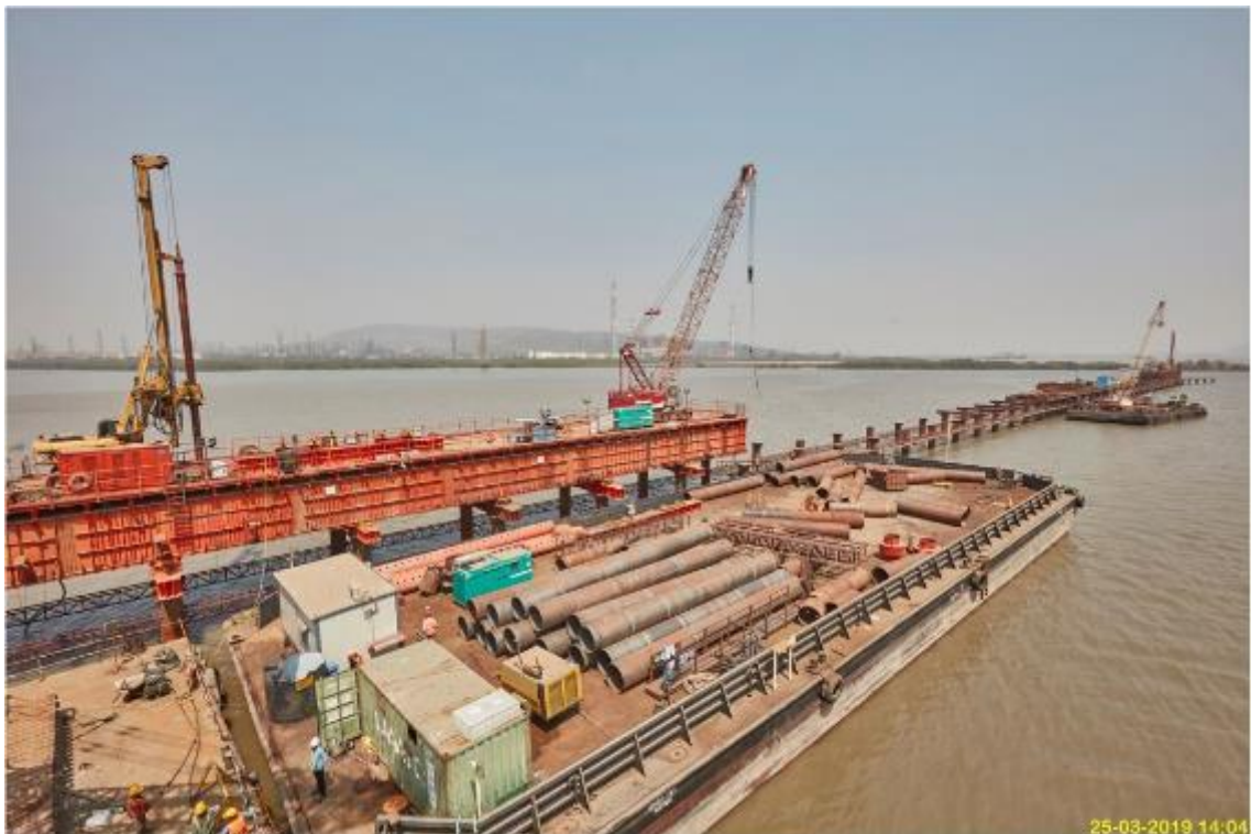
Photo No. 4: TAB Progress from MP43 location in progress
