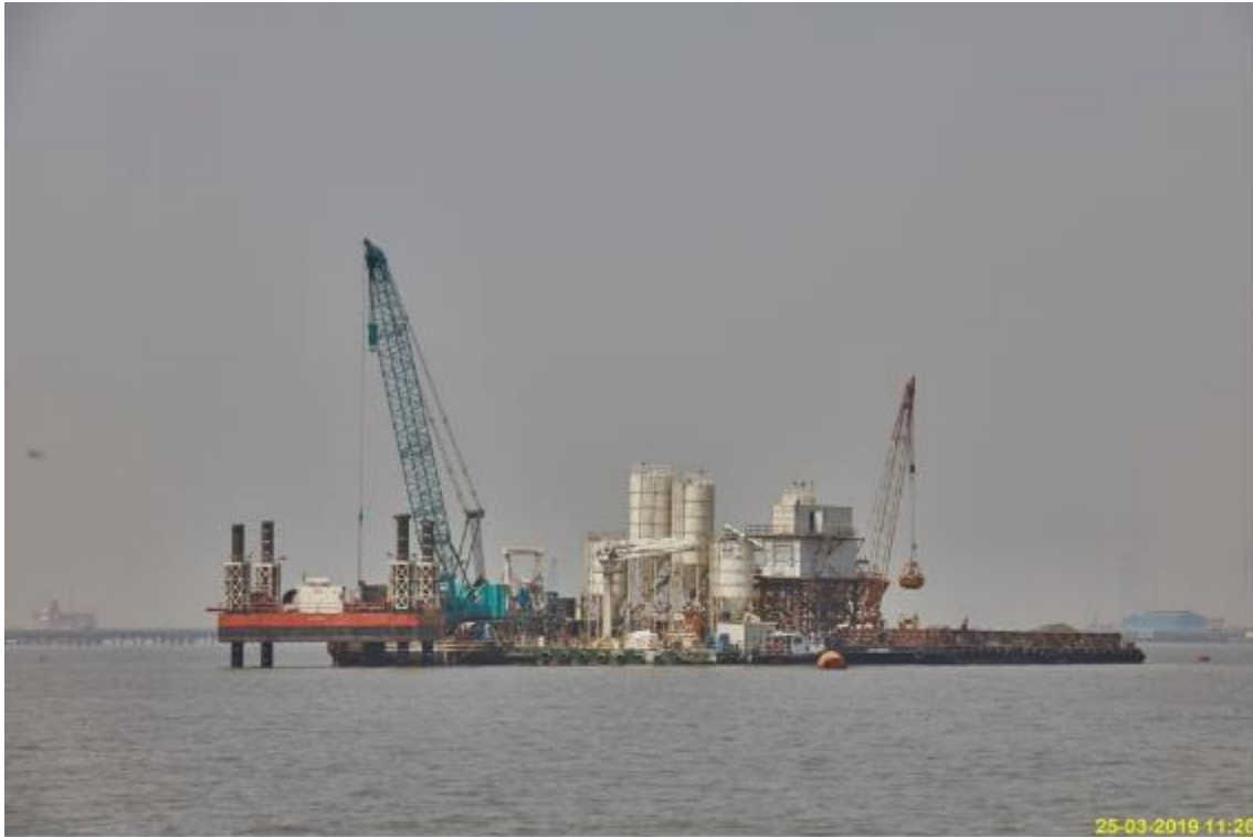
Photo No. 9: Test Pile Works at MP125 location in progress
