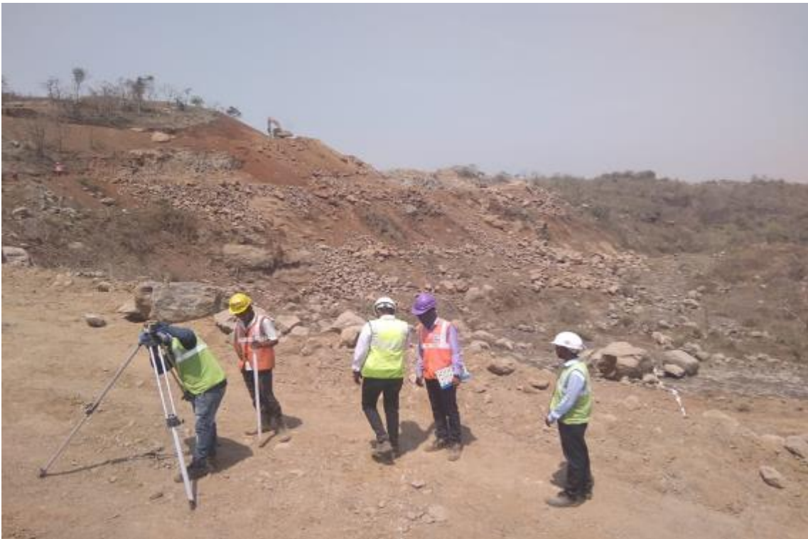
Photo No. 30: OGL survey at CH 19+980 location in progress
