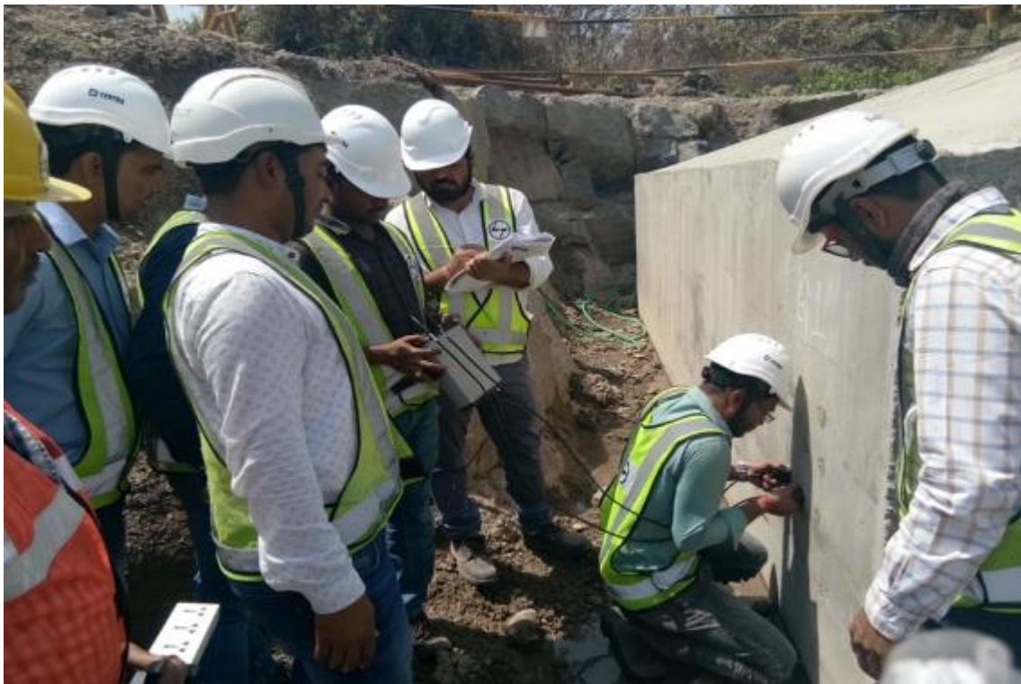
Photo No. 28: NDT Test at Foundation RMP 268 in progress
