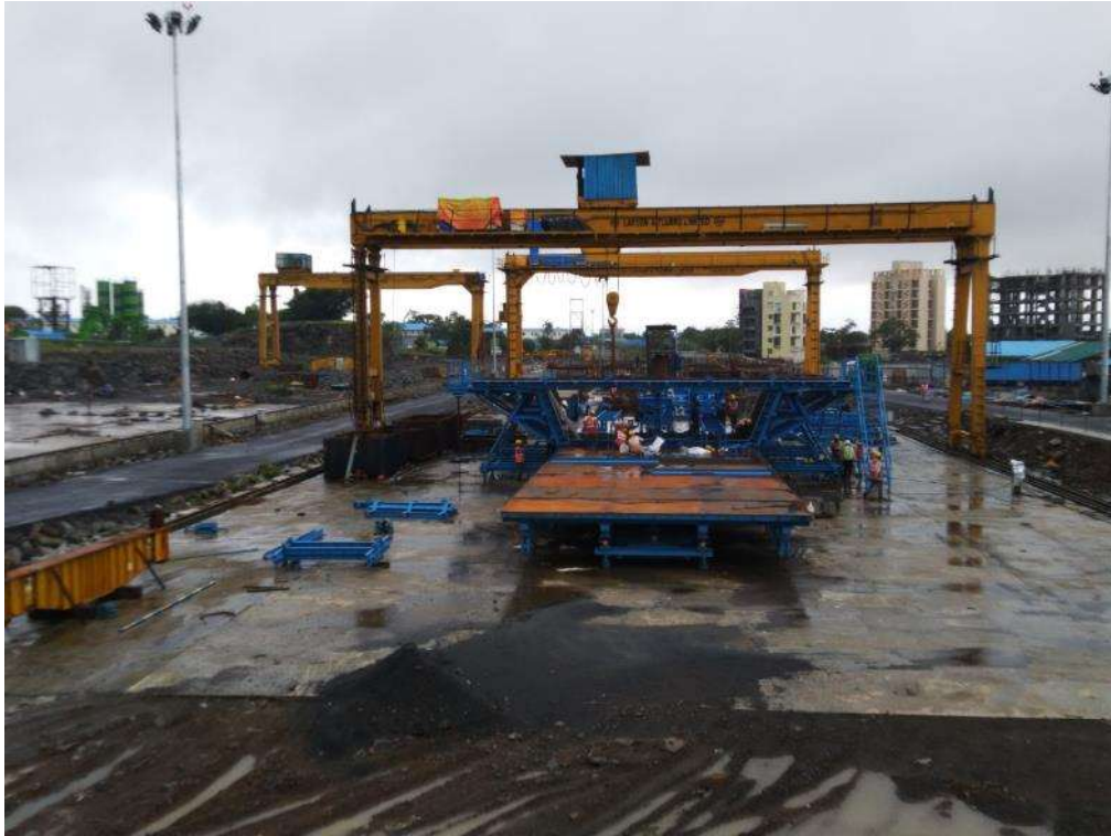
Photo No. 11: Casting Yard establishment at the Pkg-3 site
