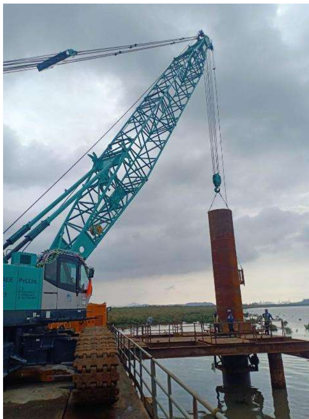
Photo No. 12: Liner driving in progress at MP 233 RHS in progress
