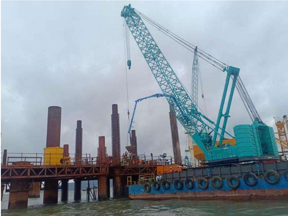
Photo No. 7: Pile Concreting at MP 158/04 RHS in progress
