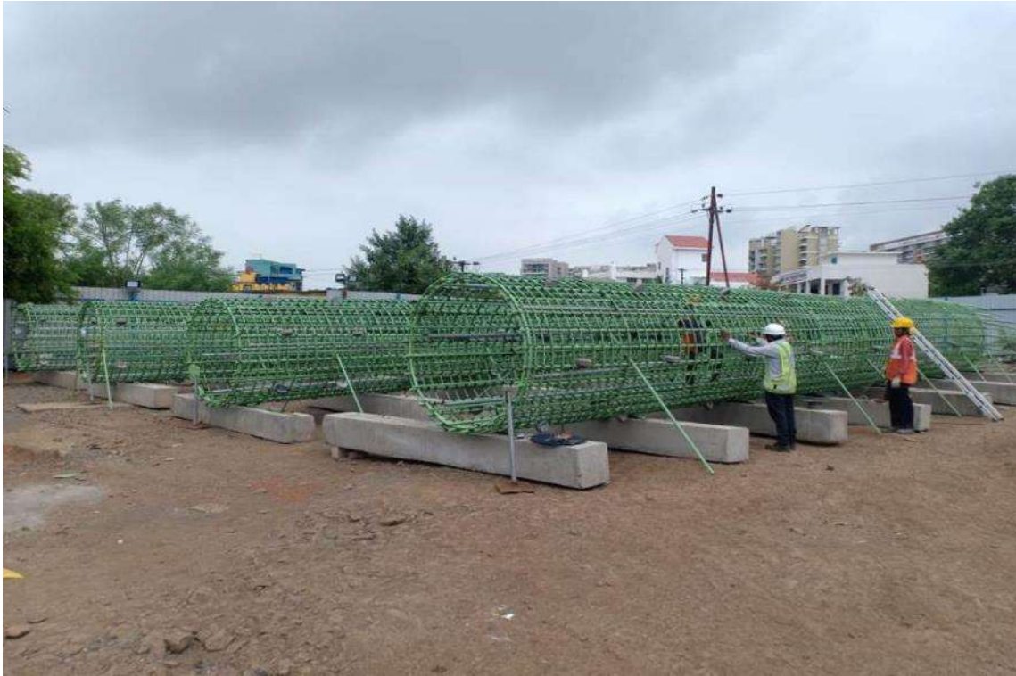
Photo No. 7: Pile Reinforcement Cage preparation at Casting Yard in progress
