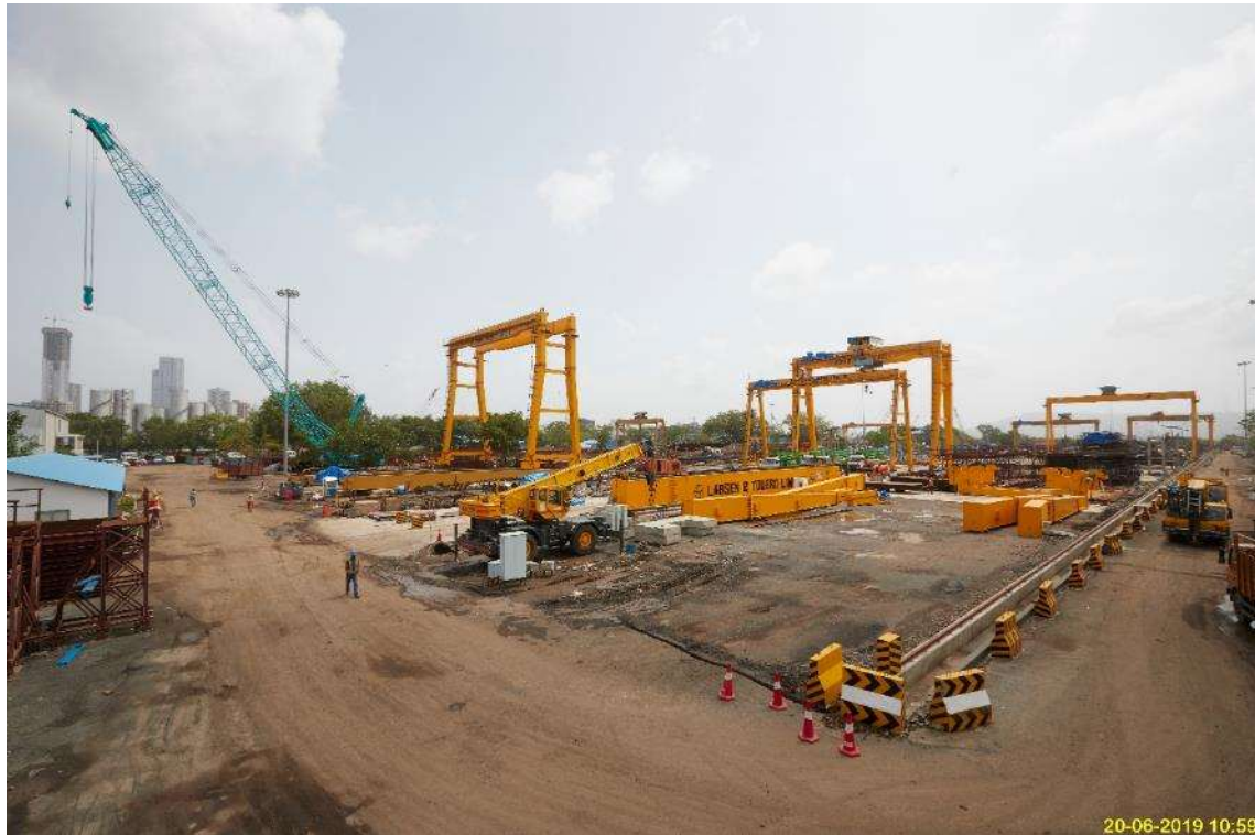
Photo No. 1: Casting Yard Development in progress
