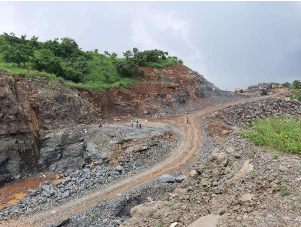
Photo No. 6: At-Grade area Access Road at CH 20+020 location
