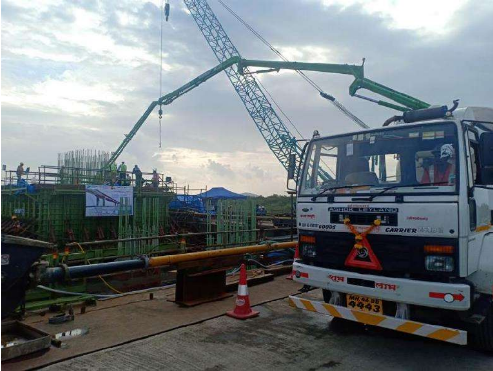
Photo No. 5: Pile Cap concreting at MP 238 RHS in progress
