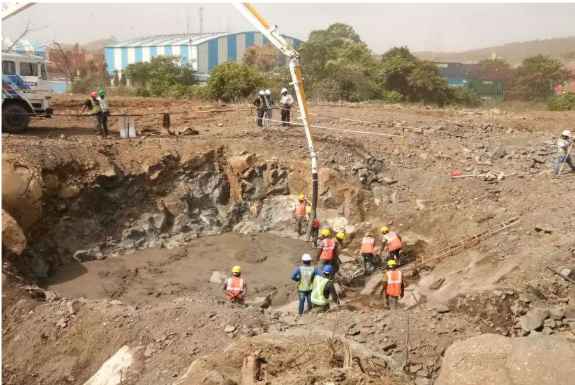
Photo No. 2: PCC works at location LP 08 in progress
