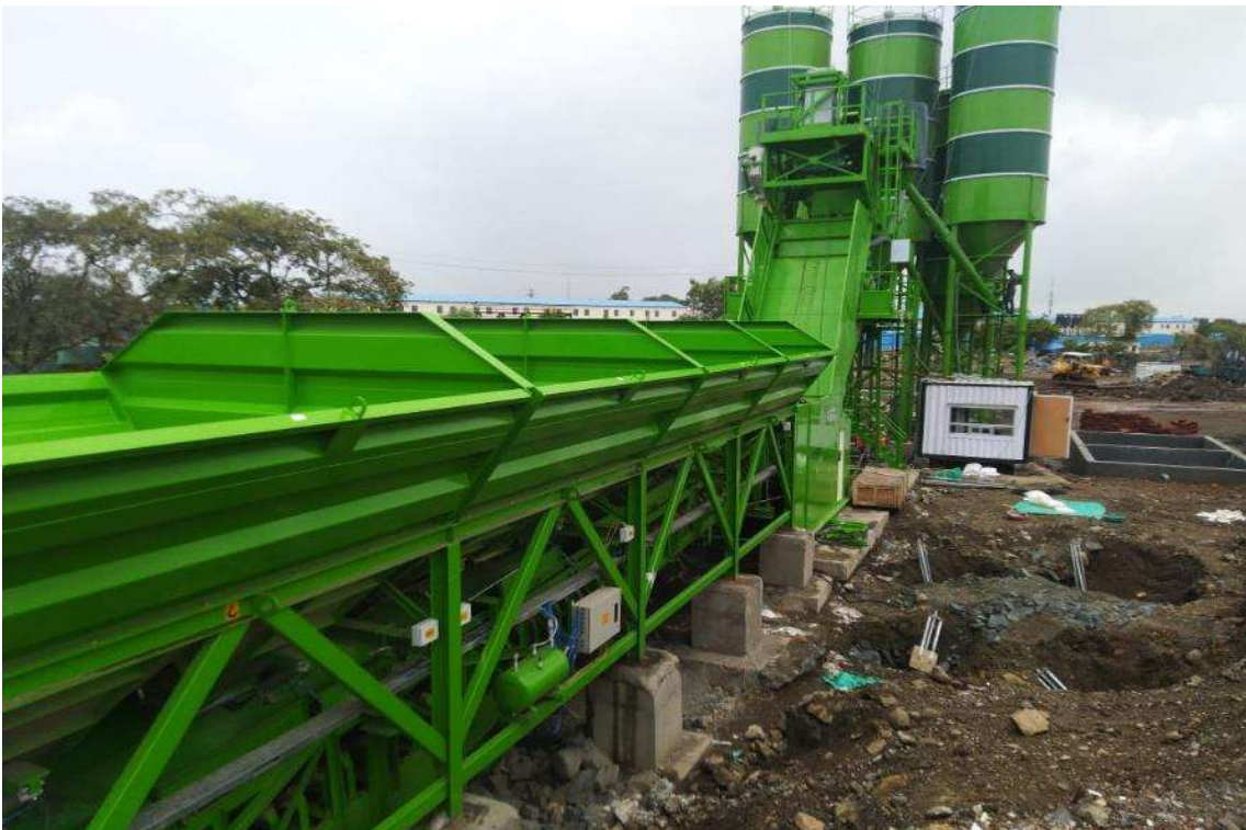
Photo No. 6: Commissioning of Concrete Batching plant in progress
