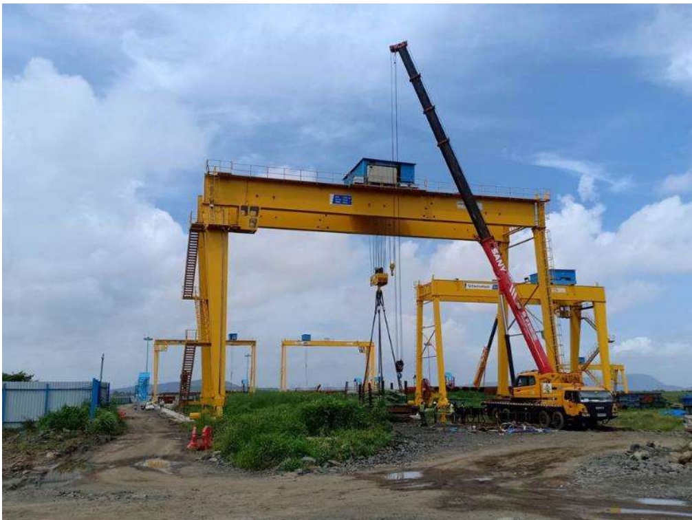
Photo No. 6: Preparatory works for Gantry Crane Load Test in progress
