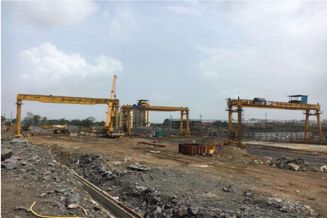
Photo No. 5: Casting Yard Establishment works in progress
