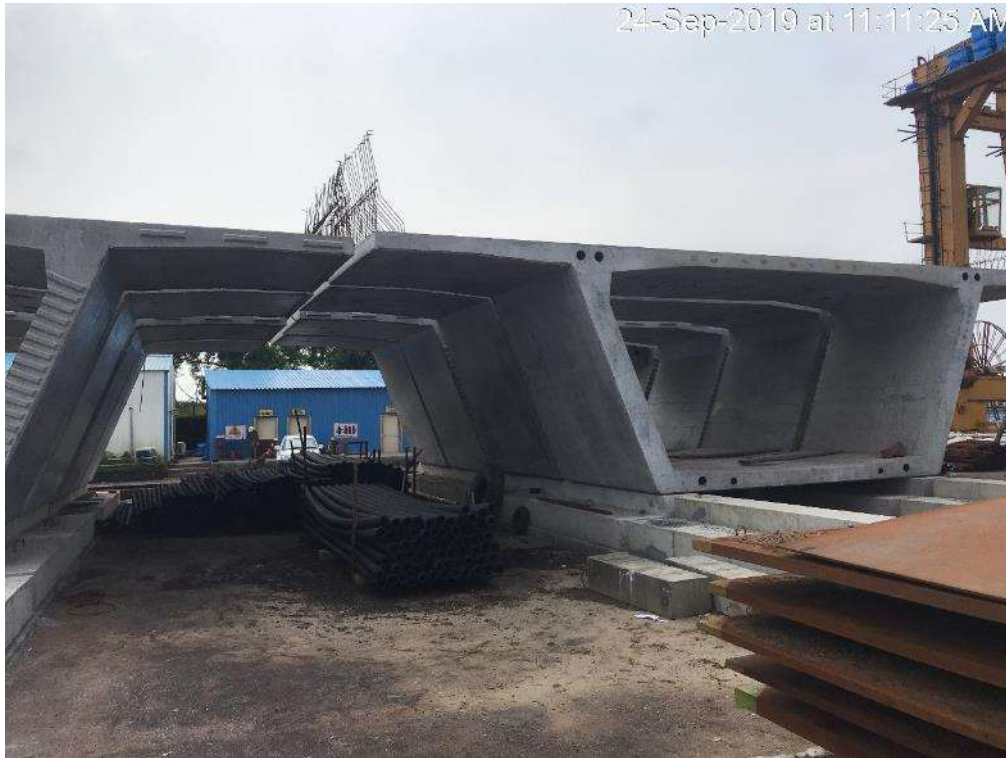
Photo No. 9: Stacking of the segment in the casting yard
