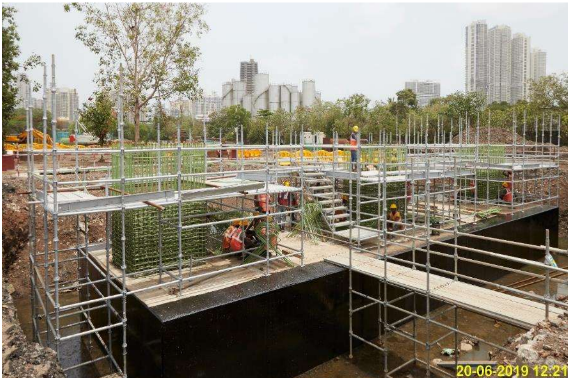
Photo No. 4: C2P5 Pile Cap and Pier Works in progress
