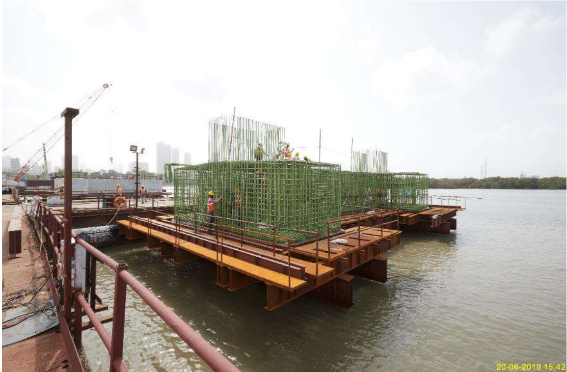
Photo No. 11: Pile Cap rebar tying works at MP11 in progress
