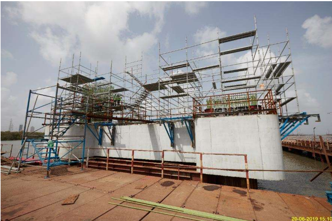
Photo No. 8: Pile Cap & Pier works at MP8 in progress
