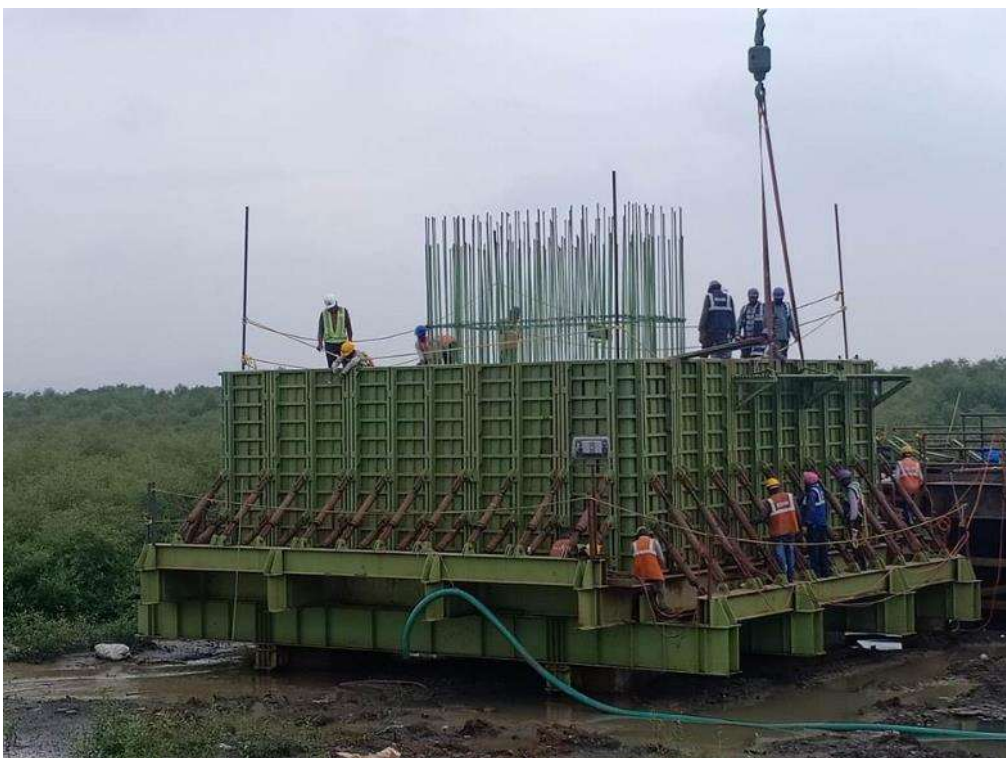
Photo No. 4: Pile Cap formwork at MP 238 RHS in progress
