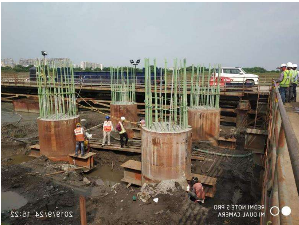
Photo No. 8: Pile Cap bottom formwork at MP 238 LHS in progress
