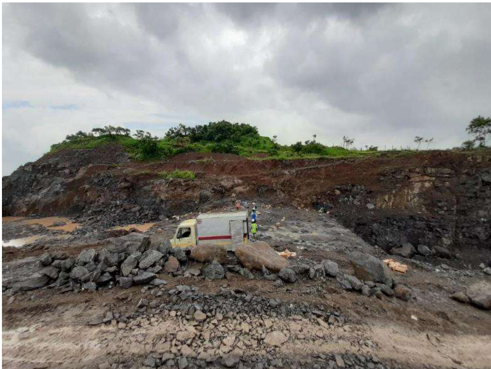
Photo No. 8: Charging for blasting works at Ch 19+800 location is ongoing
