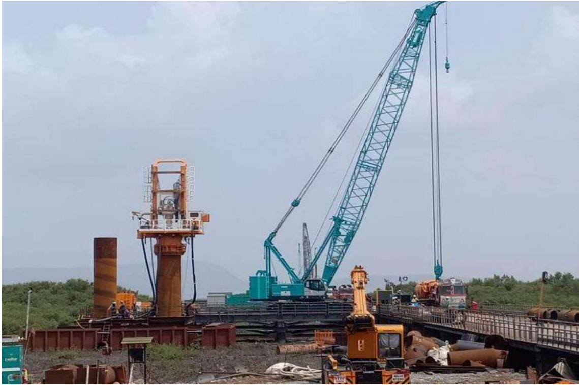
Photo No. 5: Liner Driving at MP 238/01 RHS location in progress
