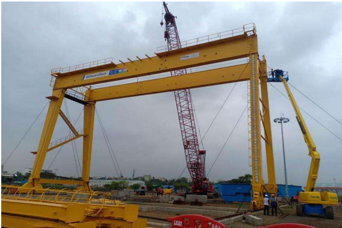
Photo No. 8: Gantry Crane erection works at Bay-3 location in progress
