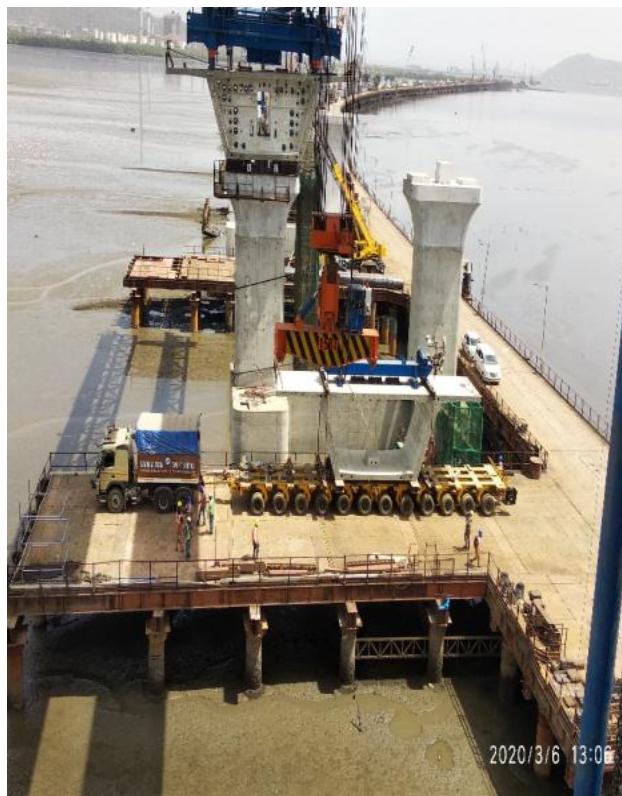
Photo No. 4: Segments Shifting For Erection- Intertidal Area
