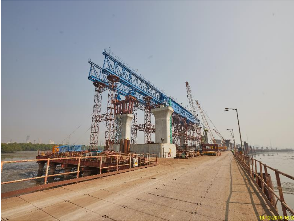
Photo No. 5: 4. Launching Girder Erection works – Intertidal is in progress
