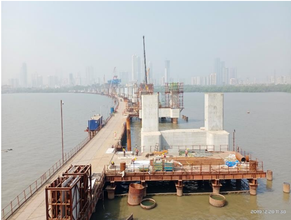
Photo No. 1: View along TAB at MP-23 seeing towards Mumbai
