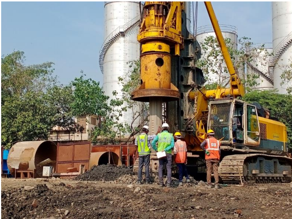
Photo No. 6: Pile boring works at Interchange area
