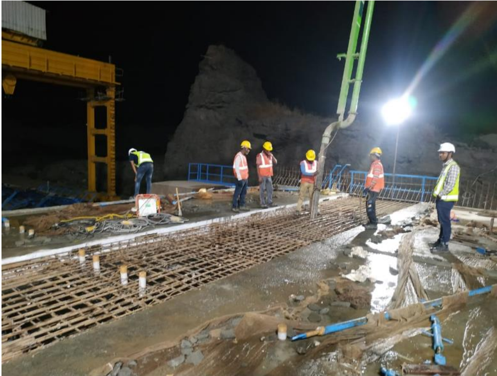
Photo No. 11: Segment Casting at PC yard is in progress
