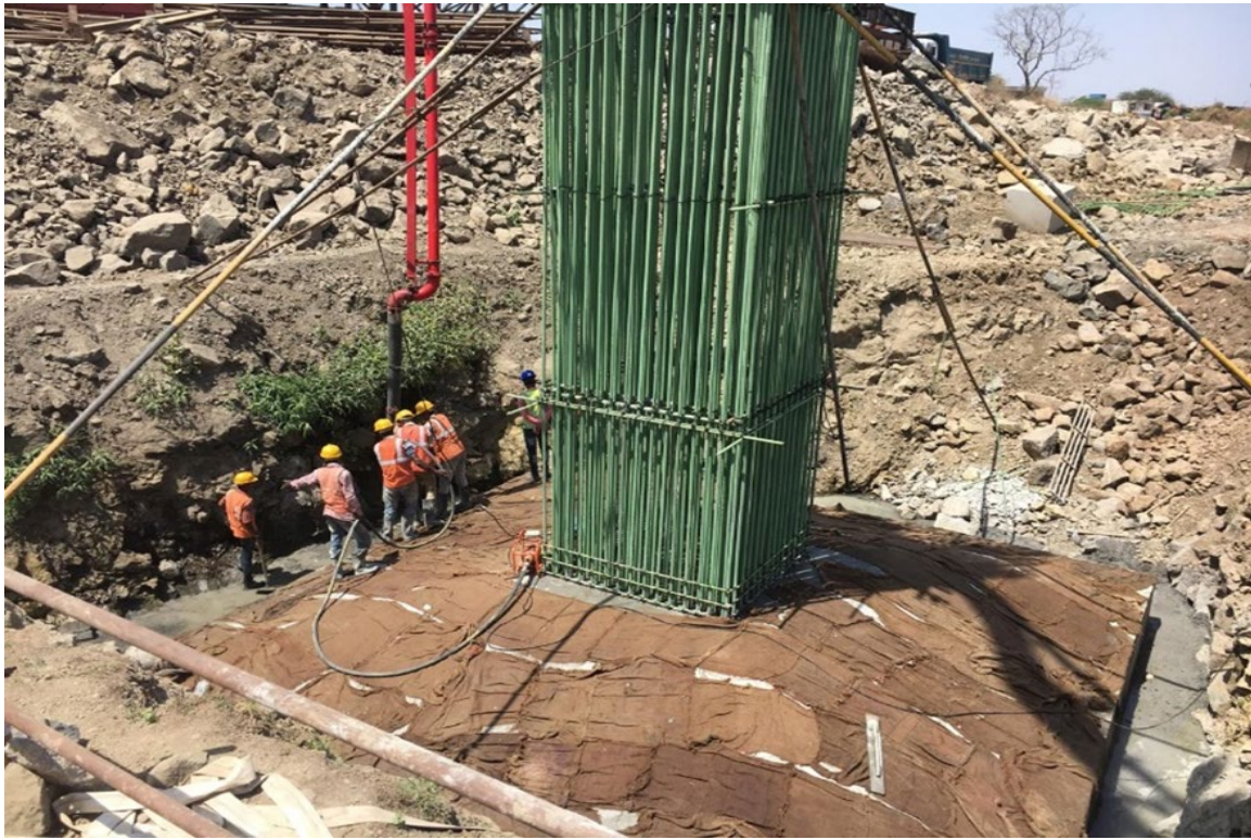
Photo No. 3: RMP 277 foundation annular filling in progress
