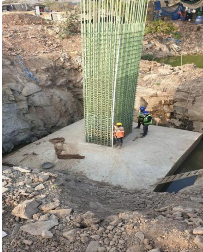
Photo No. 1: Casting of Foundation done at Location JMA1
