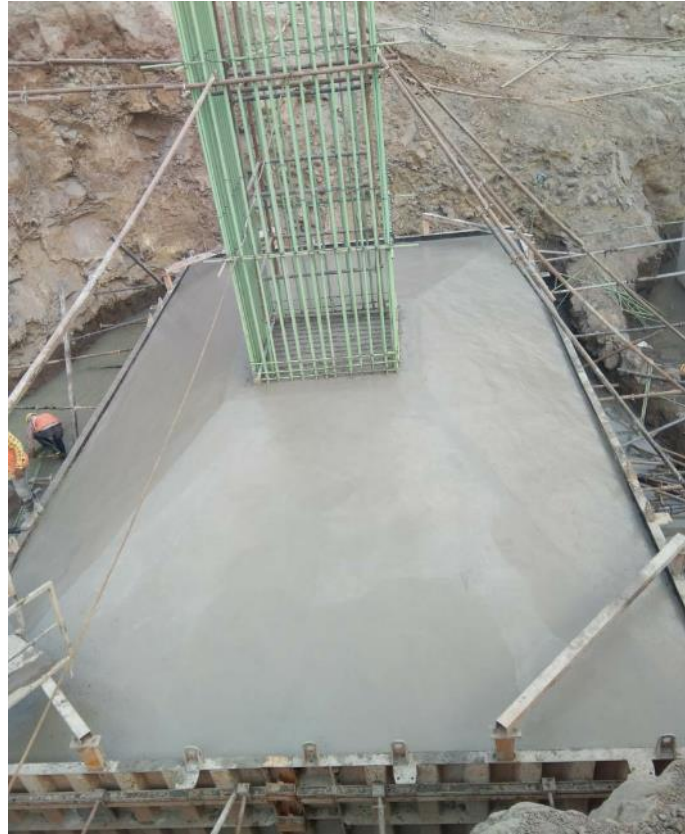
Photo No. 1: Foundation casting completed at LP 01 RHS Chirle location
