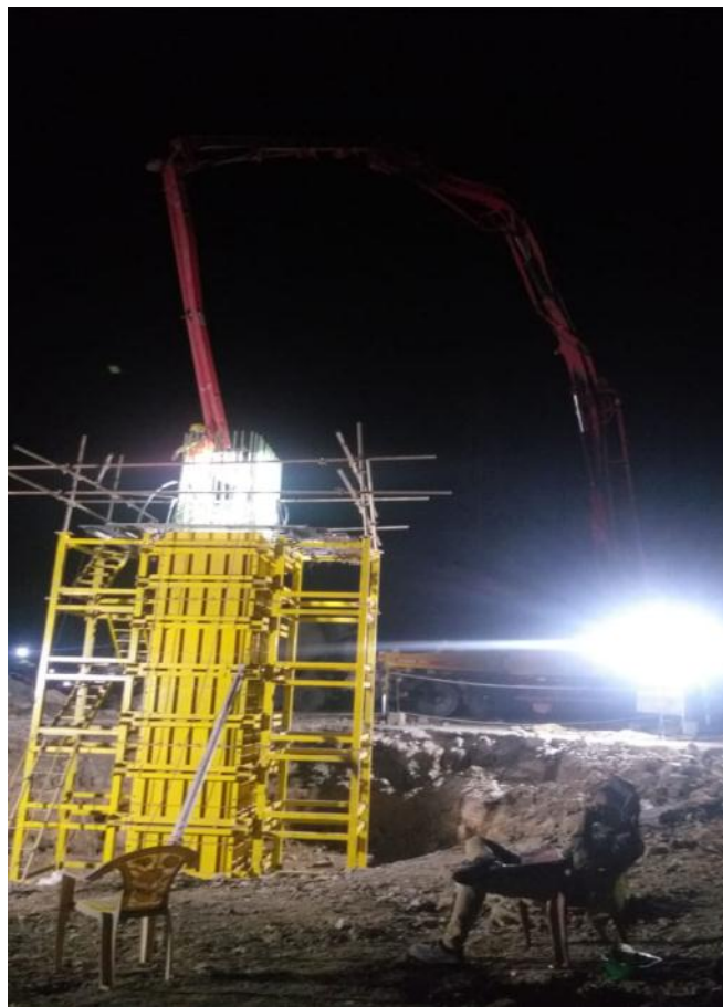
Photo No. 6: Pier Concrete at location JMP20 in progress
