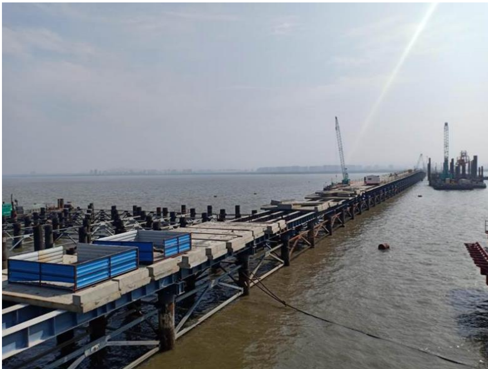
Photo No. 1: Precast Slab erection works at TAB in progress
