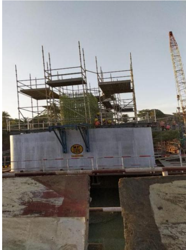
Photo No. 5: MP 02 Pier Reinforcement Inspection
