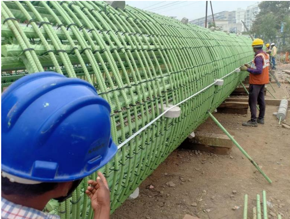
Photo No. 8: Pile reinforcement cage checking in progress
