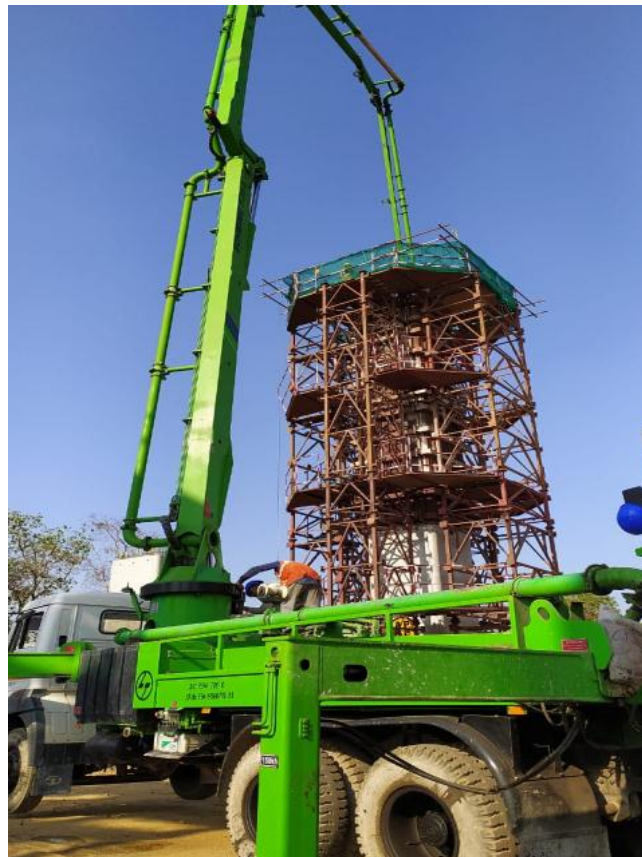
Photo No. 12: AP 46 Pier Concreting is in progress
