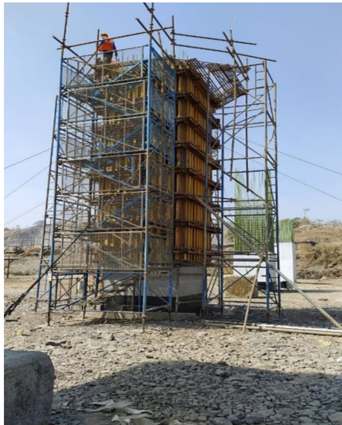
Photo No. 8: Pier Shuttering at location JMP20 in progress
