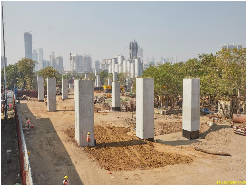
Photo No. 9: Pier Works at BP41 & BP44 – Interchange is in progress
