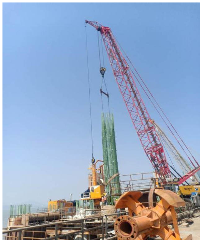
Photo No. 2: Pile reinforcement cage lowering at MP 223/02 RHS in progress
