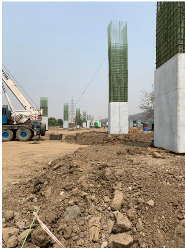
Photo No. 4: Pier Reinforcement at location LP31, RP31
