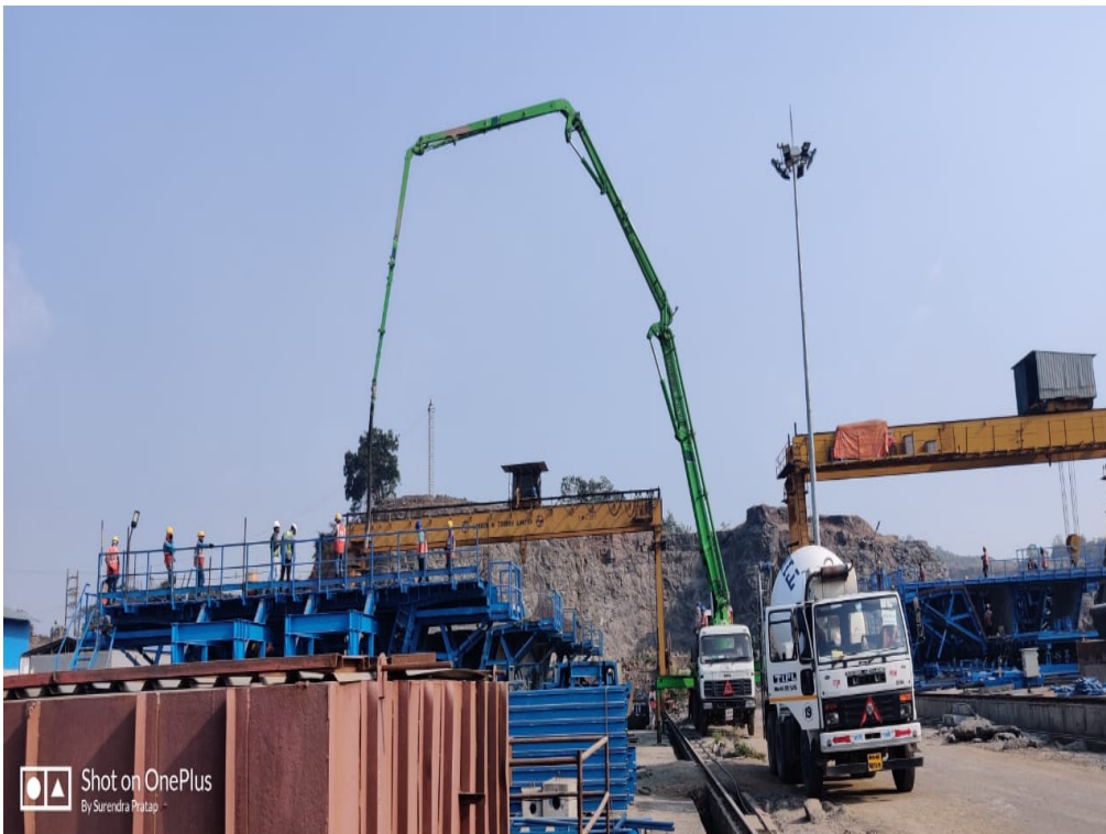
Photo No. 10: Segment Casting is in progress
