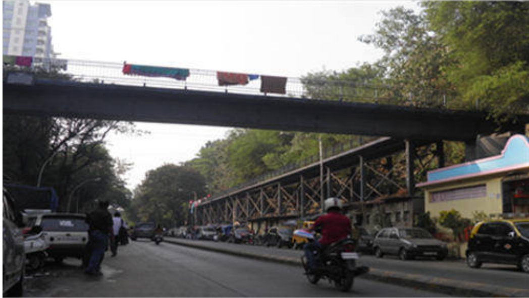
Foot Over Bridge
