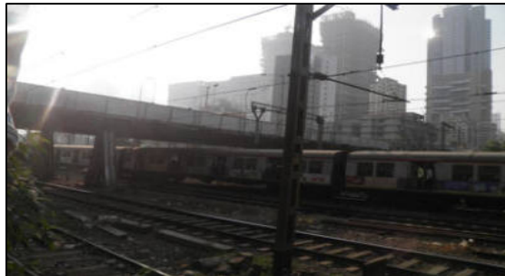
Elphinstone Station Flyover
