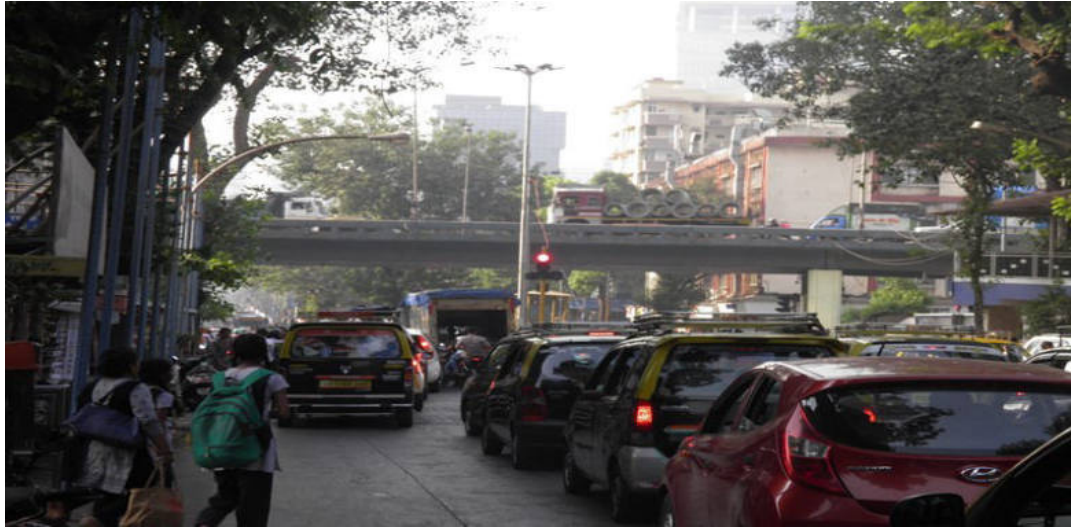
Hindmata Flyover (Parel Flyover)
