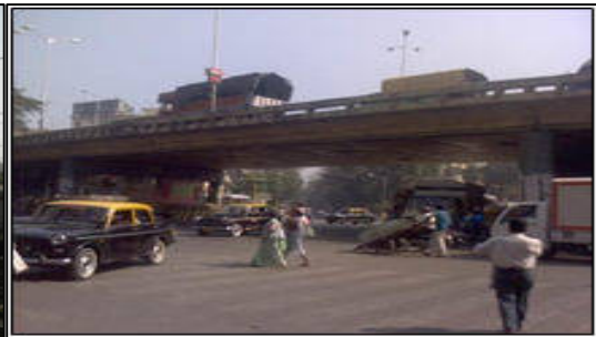
Elphinstone Station Flyover
