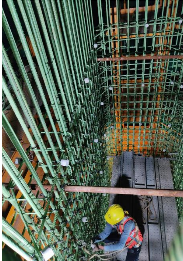
Photo No. 9: MP 118 S 2nd Lift Pier Reinforcement in progress
