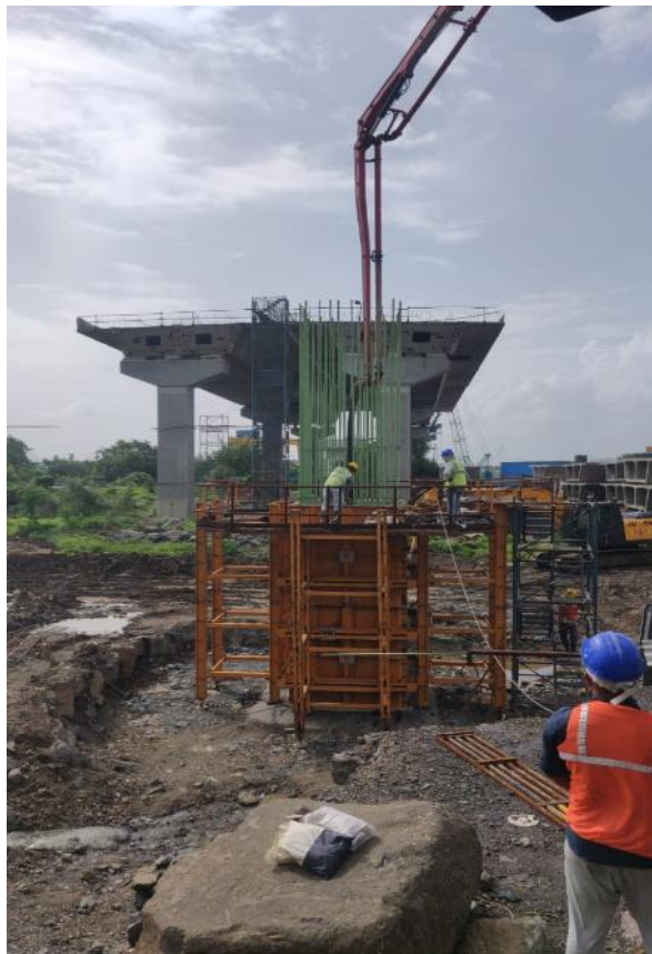
Photo No. 4: LMP 270 pier 1st lift during concrete pouring in progress
