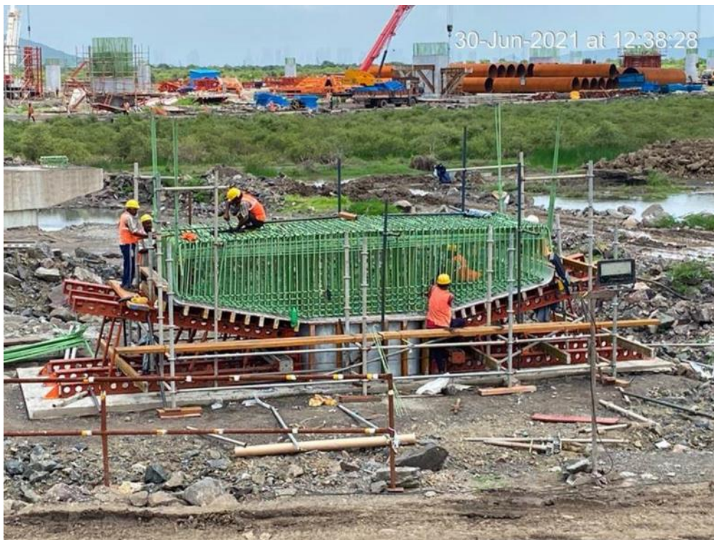
Photo No. 2: Pier cap reinforcement tying at JMP-10 in progress
