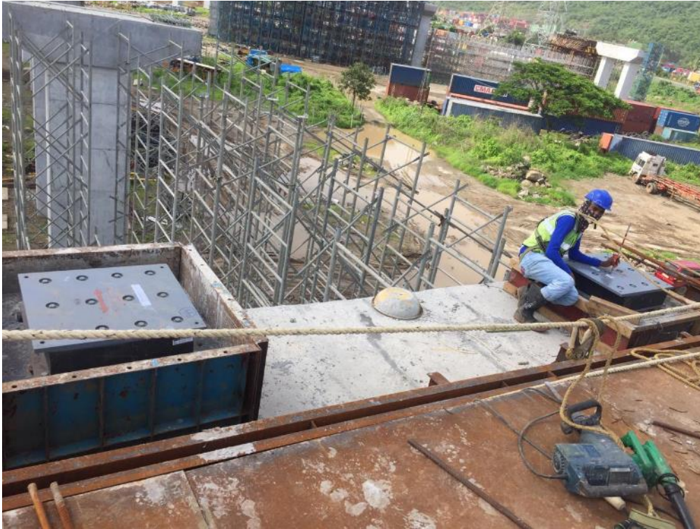
Photo No. 9: JMP15 bearing Installation inspection done
