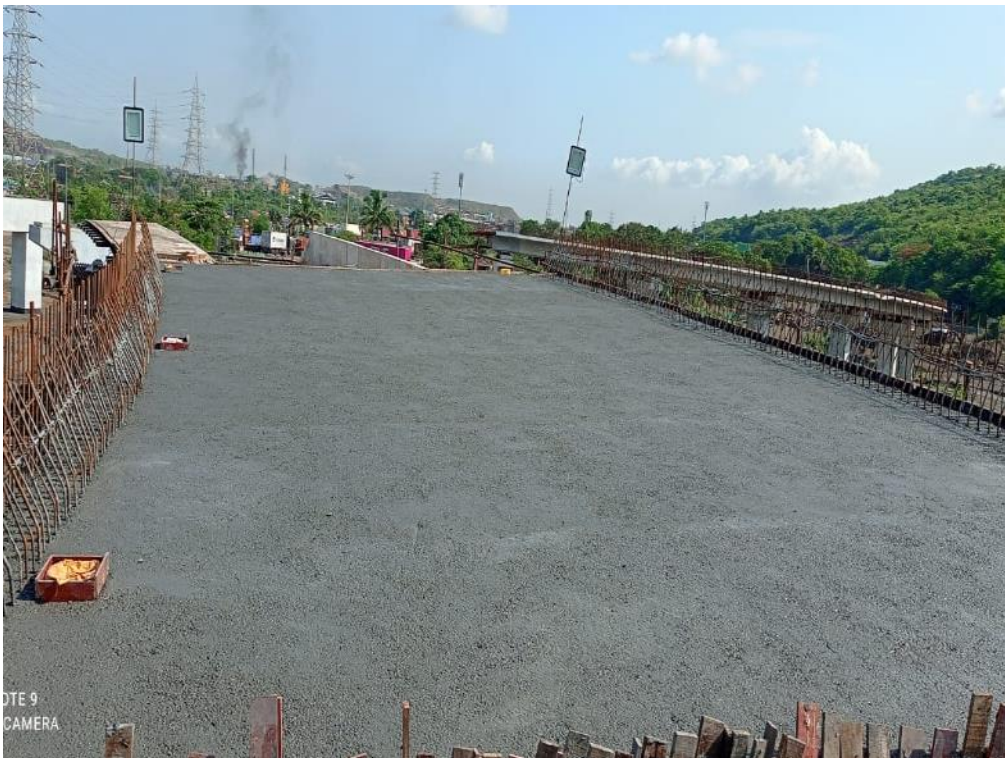
Photo No. 6: Voided slab PMP4-PMP5 concrete pour completed
