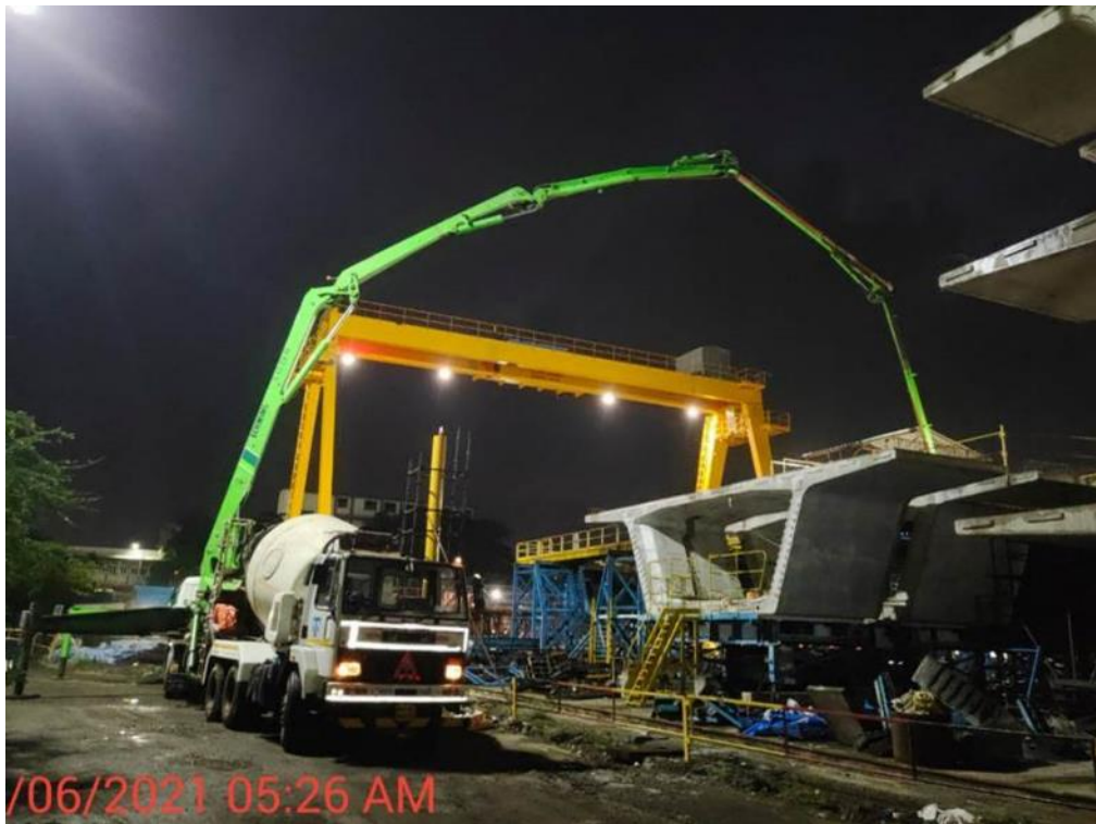
Photo No. 8: Segment concreting at Bay-4 in progress
