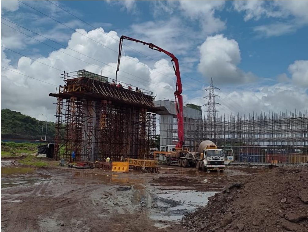
Photo No. 5: LP 33 Portal Pier Cap concrete pouring in progress
