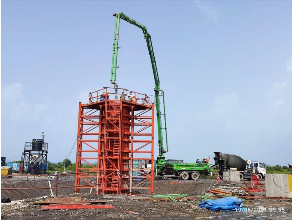
Photo No. 9: Pier concreting at JMP-1 LHS in progress
