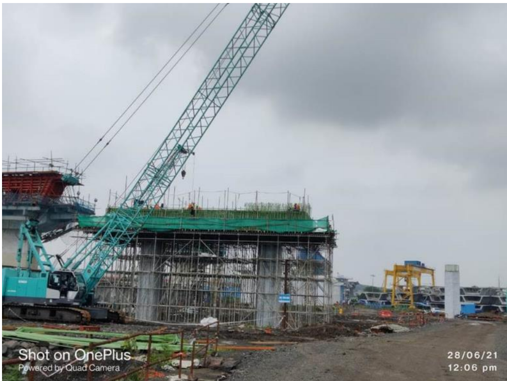
Photo No. 4: Portal Beam reinforcement tying at MP 259 RHS in progress
