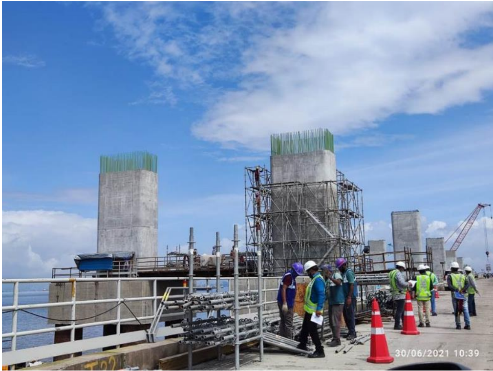
Photo No. 1: EJ Pier cap scaffolding at MP 216 LHS in progress
