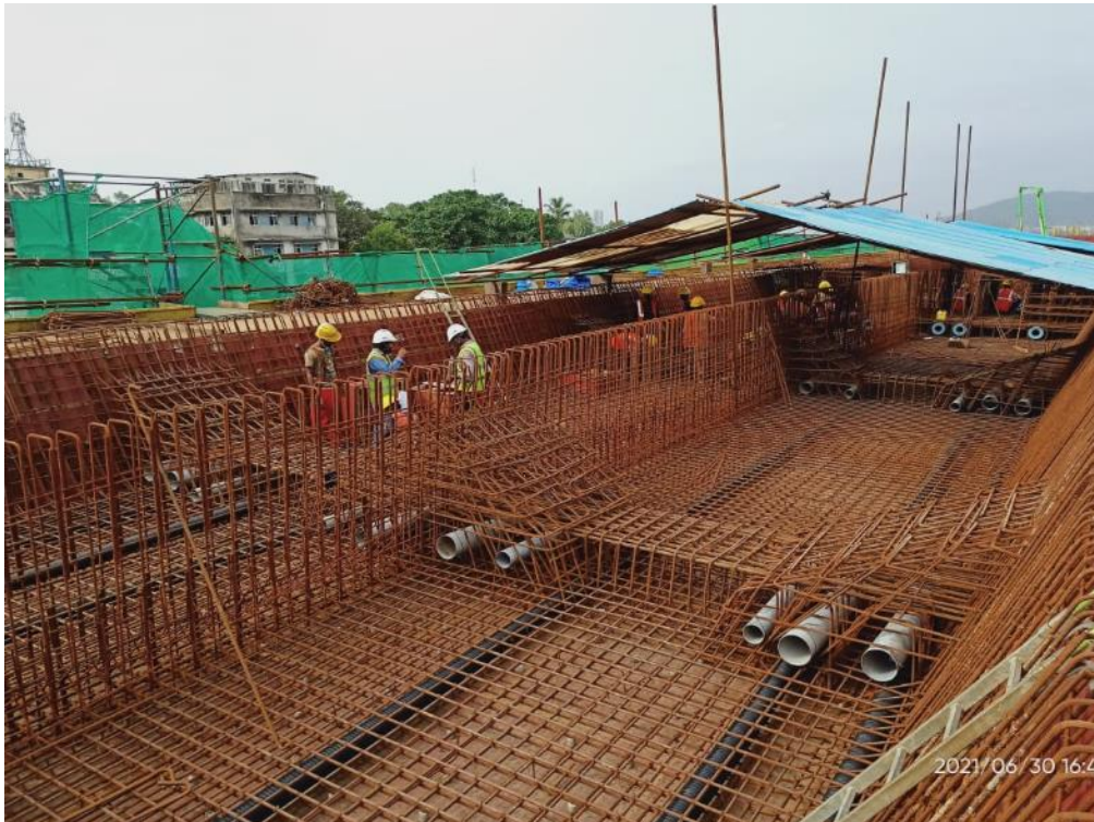
Photo No. 12: BP 49-50 Cast In-situ Rebar Works -Interchange Section in progress
