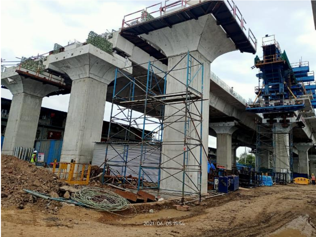
Photo No. 3: LG-05 at Ramp BP, C1 and C2 in progress
