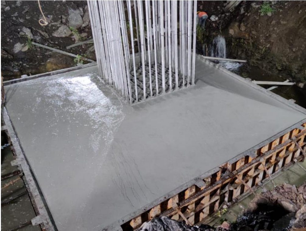
Photo No. 3: Foundation LMP 275 concrete pour completed
