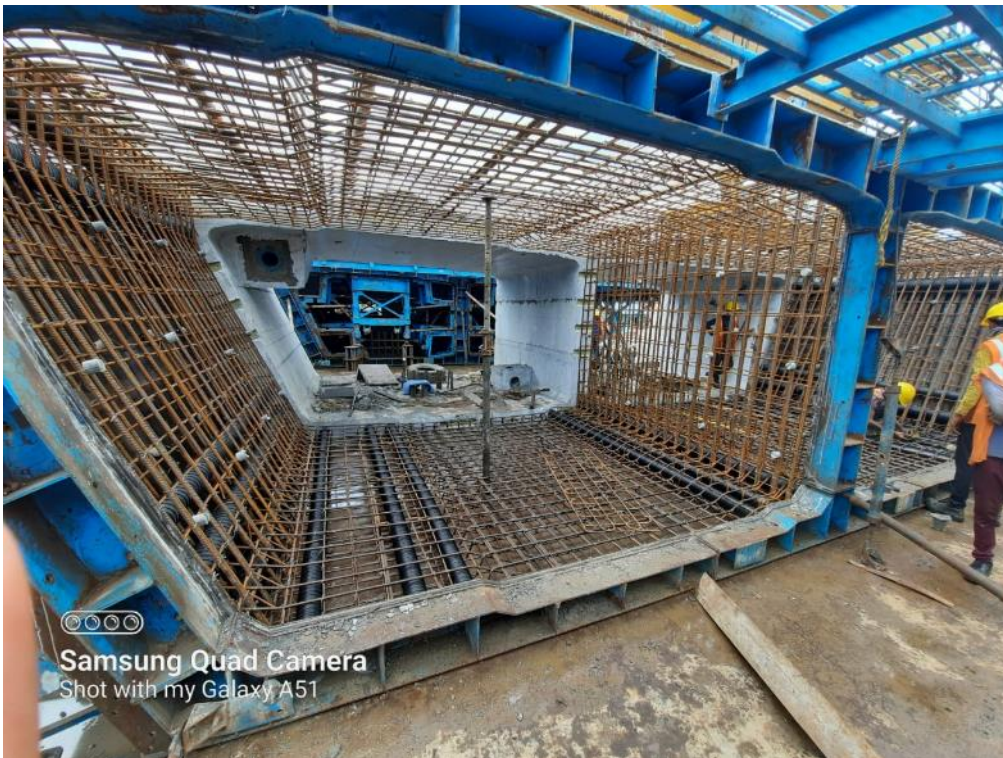
Photo No. 10: Precast segment reinforcement and profile
