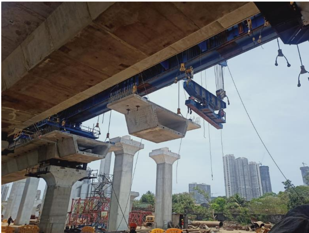
Photo No. 4: LG-05 Segments Lifting in progress
