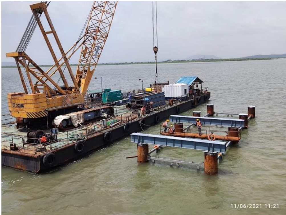
Photo No. 11: Crane platform erection works at Intertidal Zone in progress
