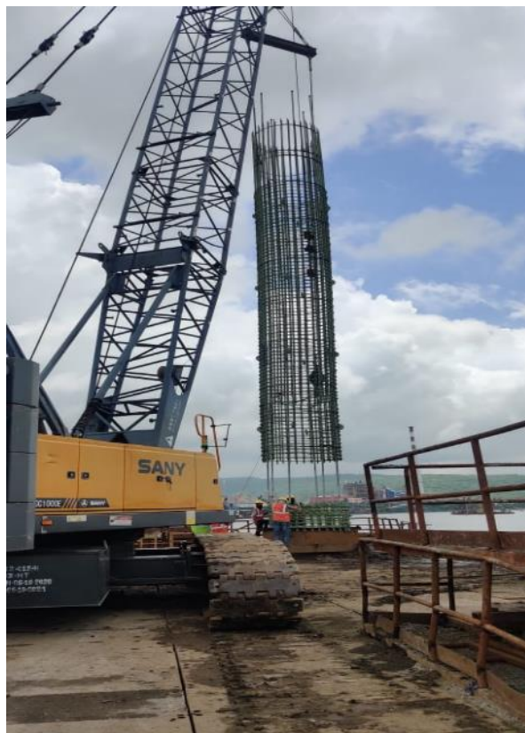
Photo No. 6: MP 60 N1 Pile Cage Lowering – Intertidal Section in progress
