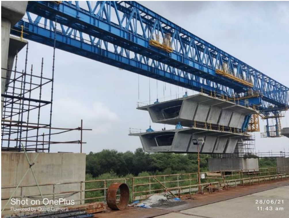
Photo No. 3: LG-1 Segment erection at Span MP 237-236 RHS in progress
