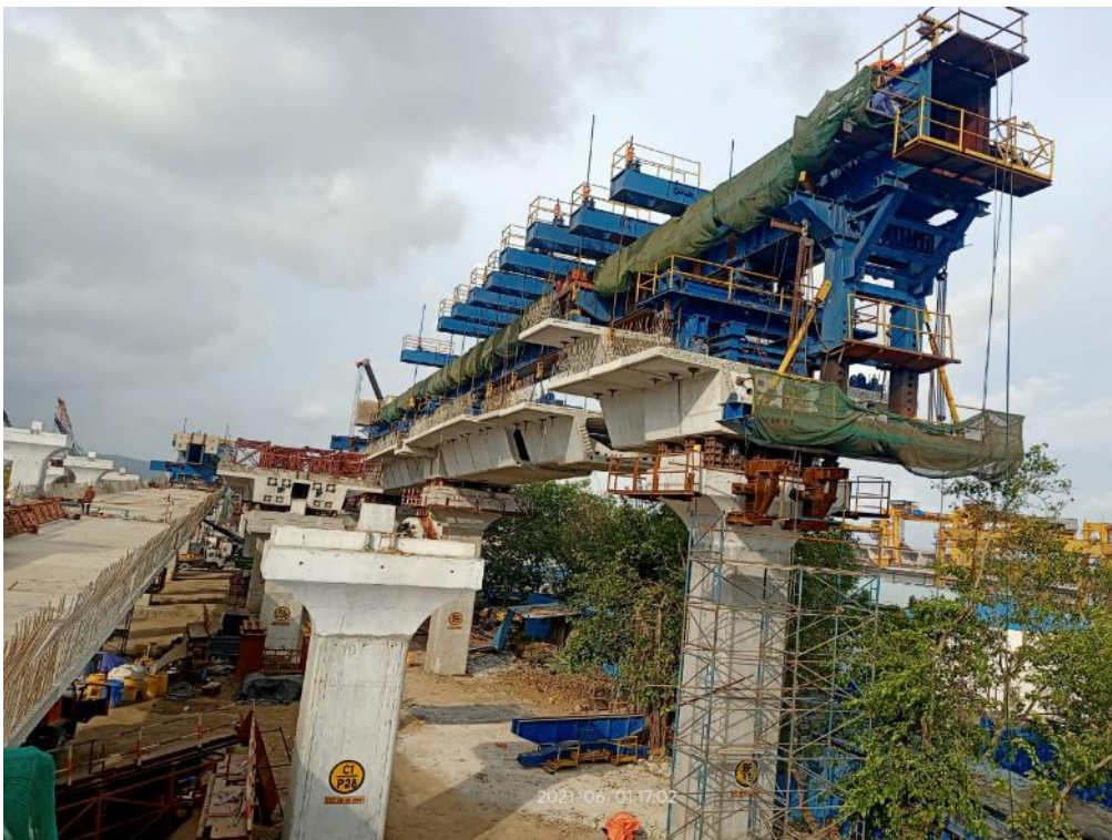
Photo No. 2: LG-06 BP 37-38 Erection Works - Interchange Section in progress
