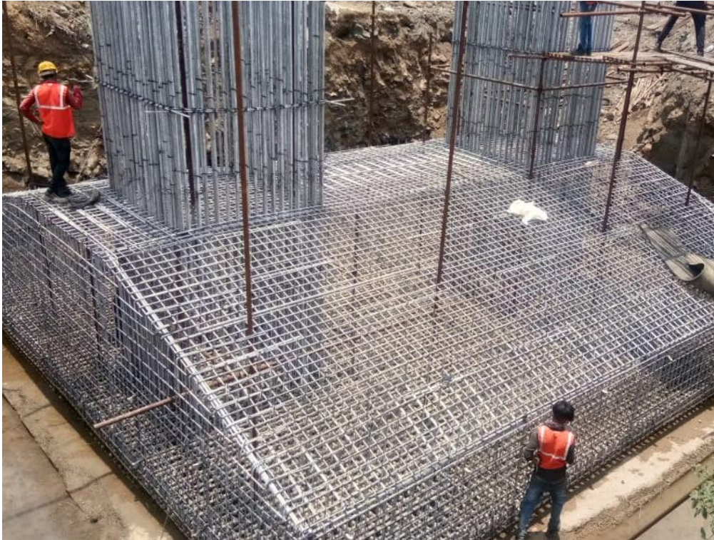
Photo No. 1: LMP 274 Foundation Reinforcement in progress
