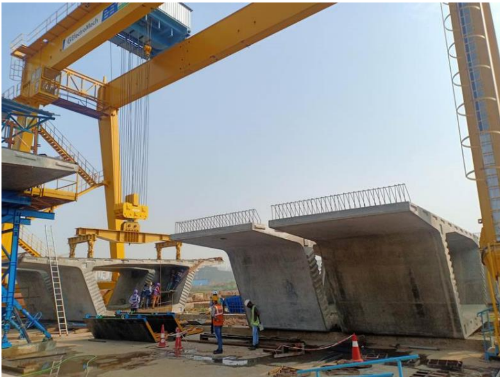
Photo No. 6: Segment lifting and stacking at Bay-3 in progress
