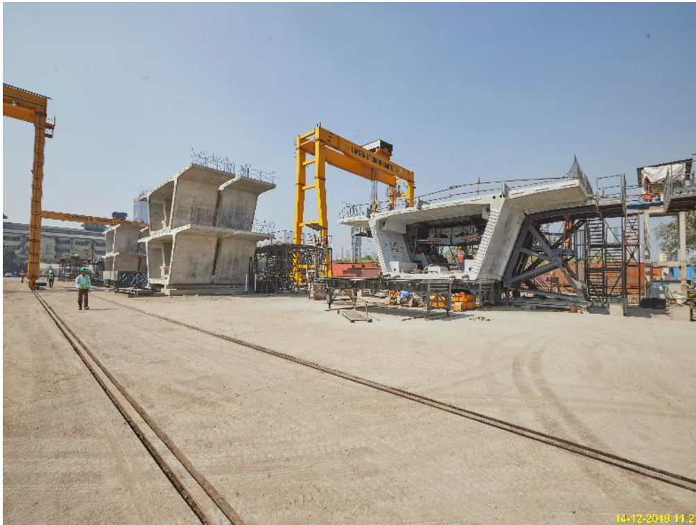
Photo No. 7: Precast Yard - Segment casting in BAY-2 is in progress
