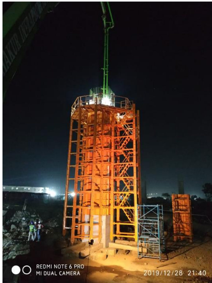
Photo No. 4: Pier casting works at Pier location LMP 280 in progress
