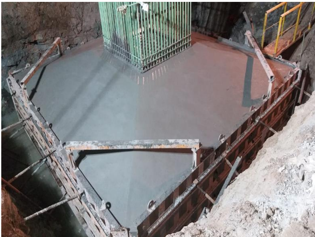
Photo No. 2: Foundation casting completed at LP 31 Chirle location
