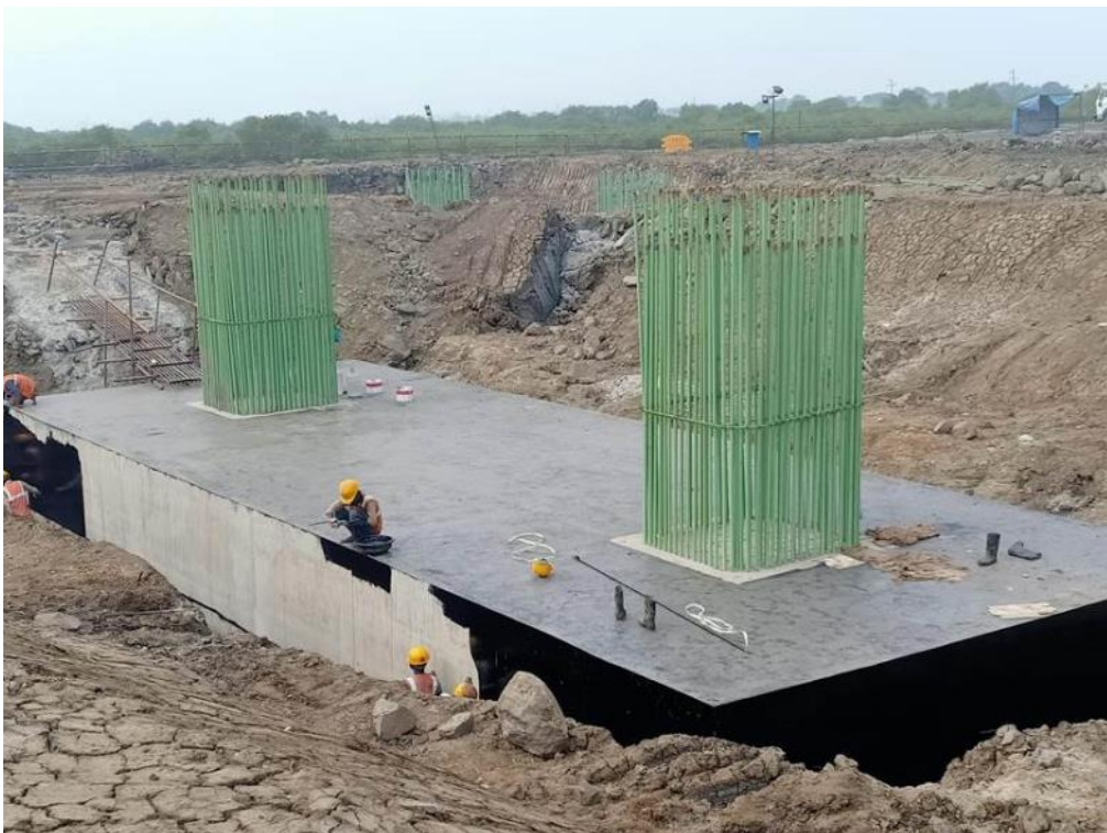
Photo No. 10: Coal Tar epoxy application at Open foundation MP 245 LHS in progress
