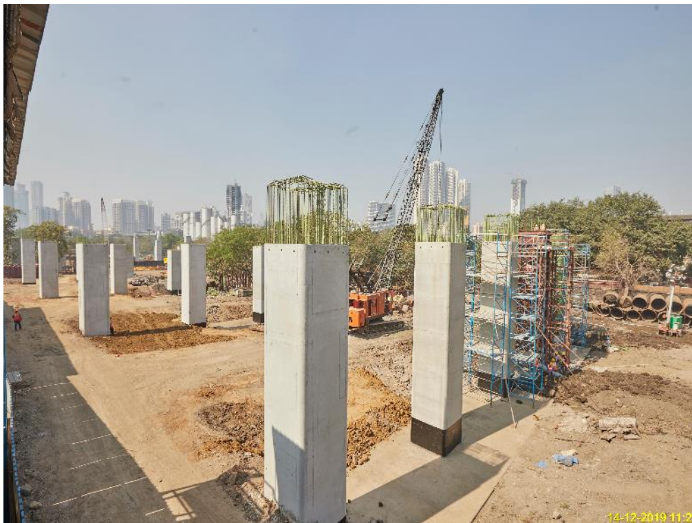
Photo No. 8: Pier Works at BP44 & BP45 – Interchange is in progress
