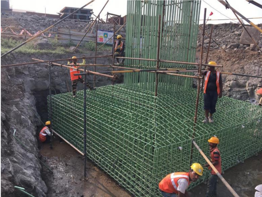
Photo No. 3: Foundation Reinforcement Works at RMP 280 is in progress
