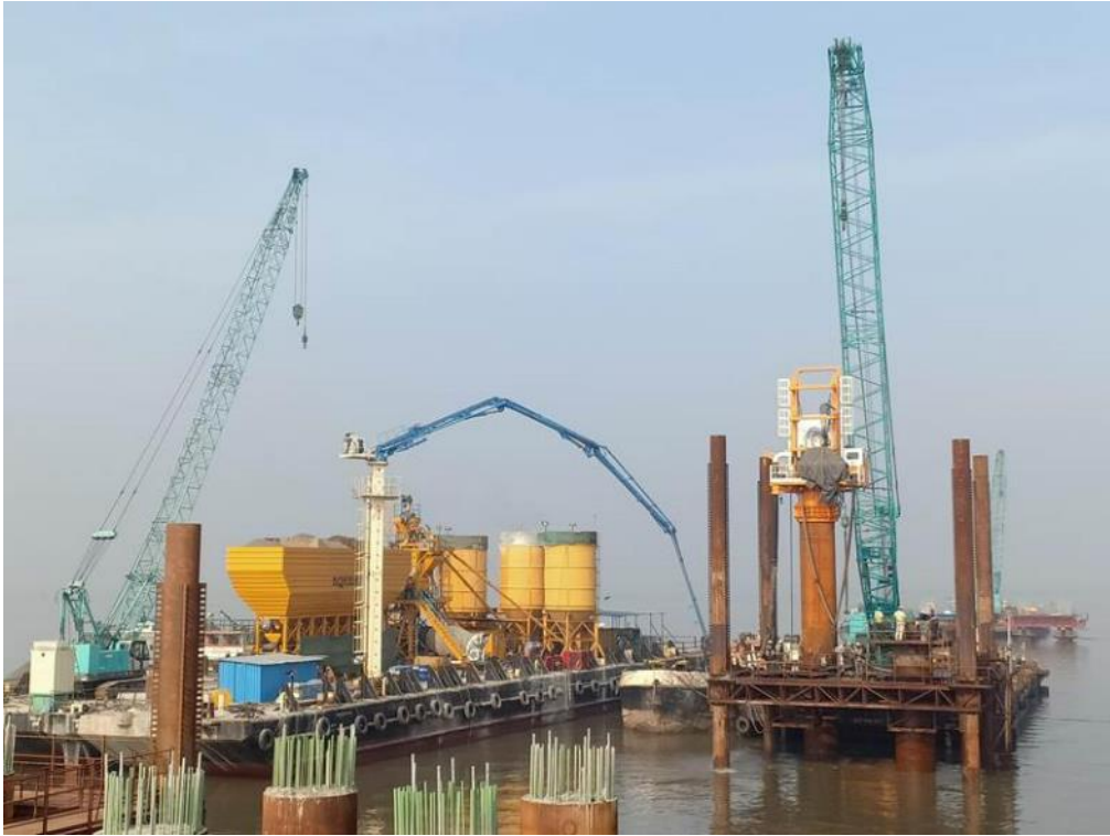
Photo No. 5: Preparatory works at MP 209 LHS location in progress
