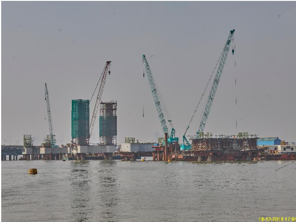
Photo No. 3: Work in Progress between MP81 & MP85
