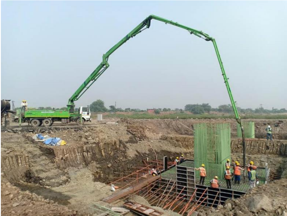
Photo No. 9: Open foundation concreting at MP 243 LHS in progress
