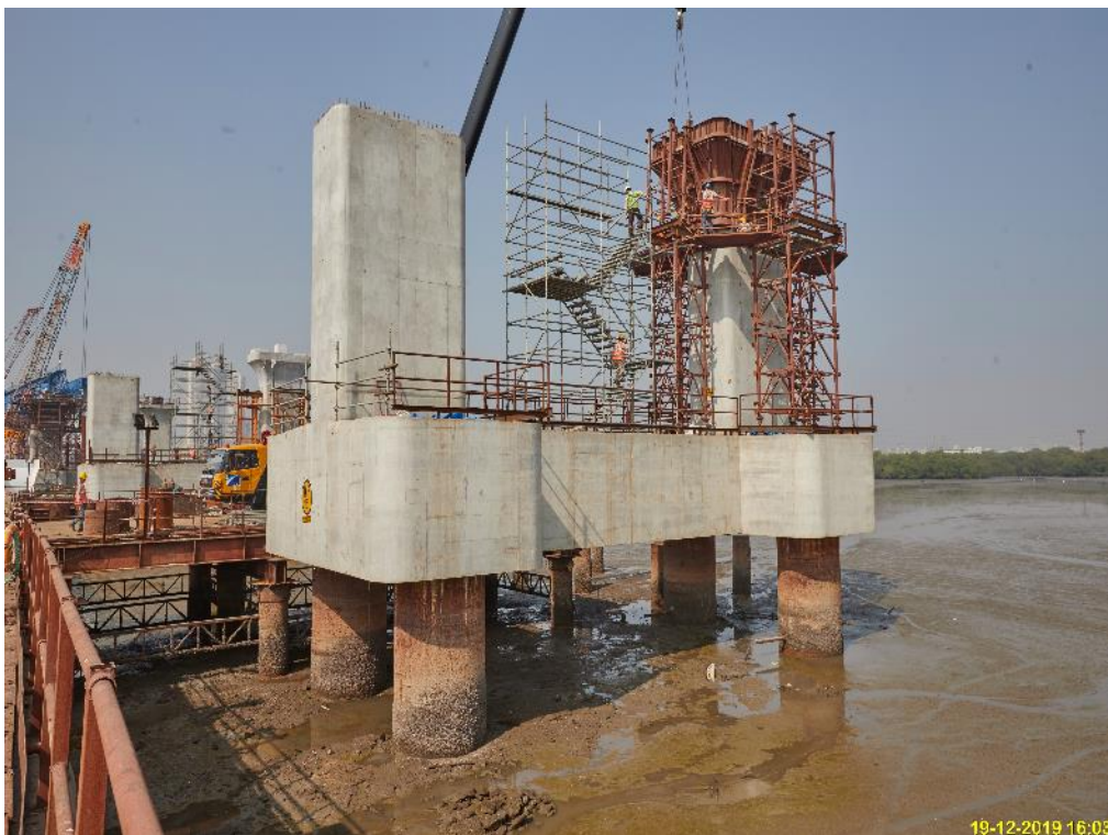
Photo No. 4: MP15 Pier cap works – Intertidal is in progress
