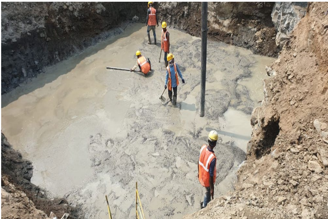
Photo No. 2: PCC concrete pouring at location JMP09
