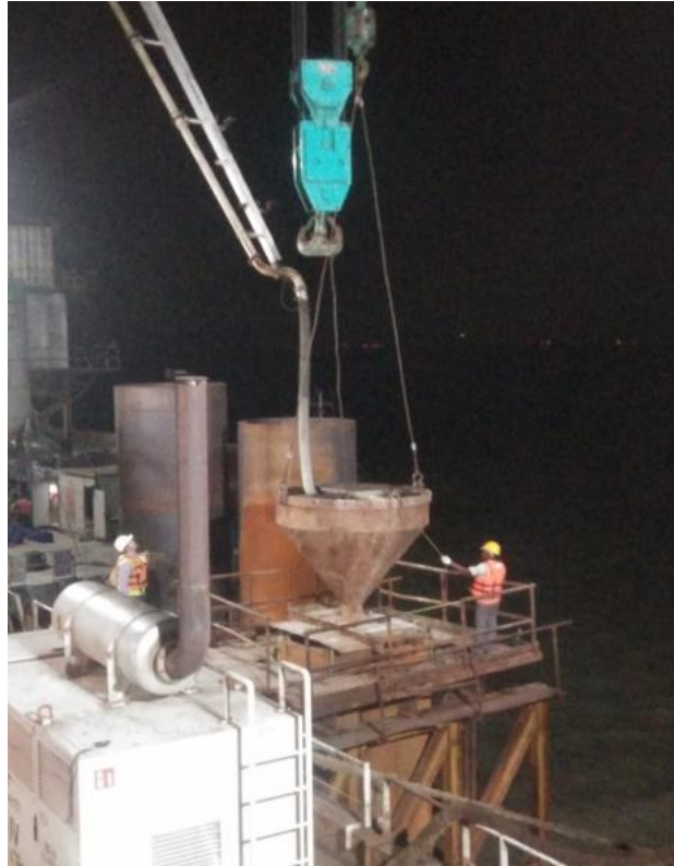
Photo No. 3: MP 104 Pile Concreting- Marine Area
