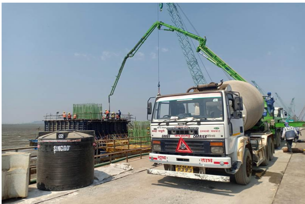
Photo No. 6: Pile cap concreting at MP 228 RHS in progress
