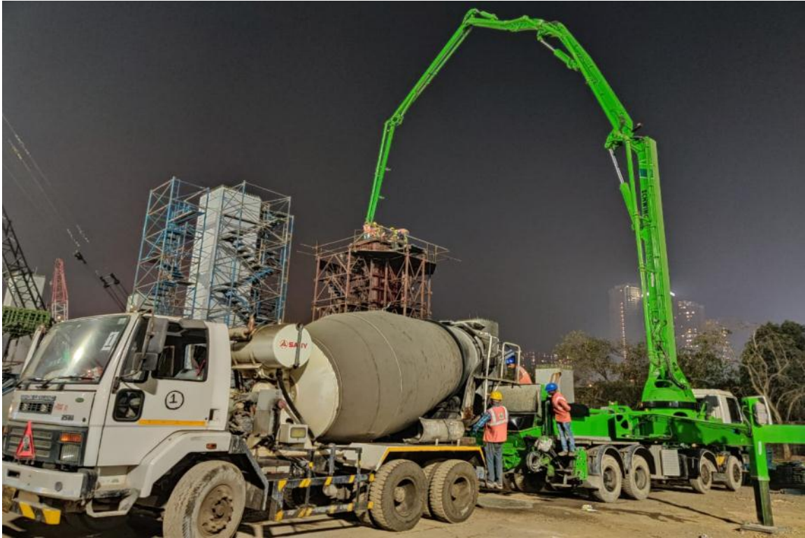
Photo No. 7: Intertidal pier concreting in progress
