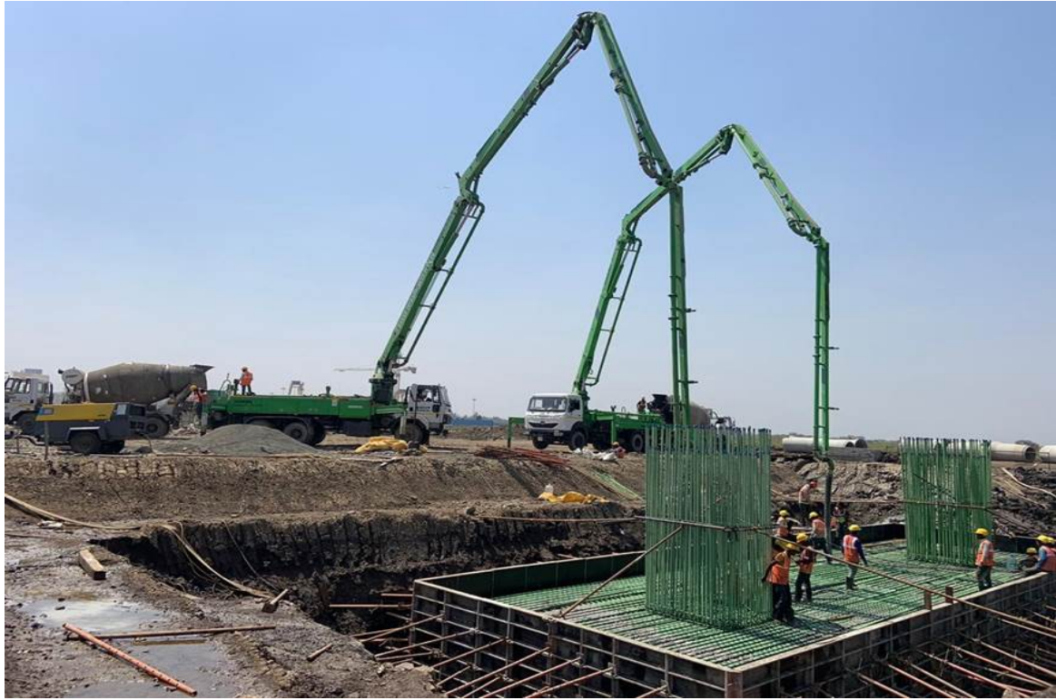
Photo No. 11: Open foundation concreting at MP 261 RHS in progress
