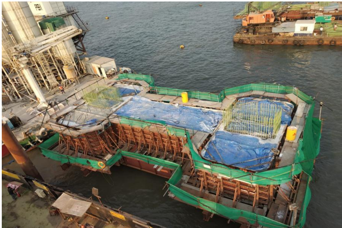
Photo No. 2: MP 104 Pile Cap Concreting- Marine Area
