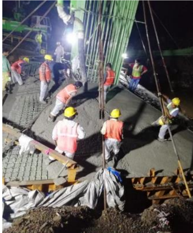
Photo No. 3: Concreting Works at Foundation No. RP 01 LHS in progress
