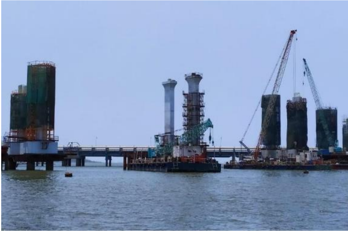
Photo No. 11: Marine Section- Progress View looking at MP 81-85
