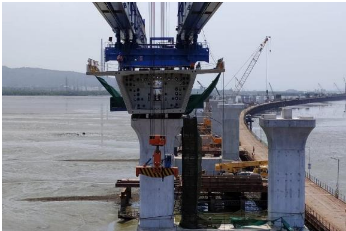
Photo No. 6: MP 15-16 Pier Head Erection Intertidal Section In Progress
