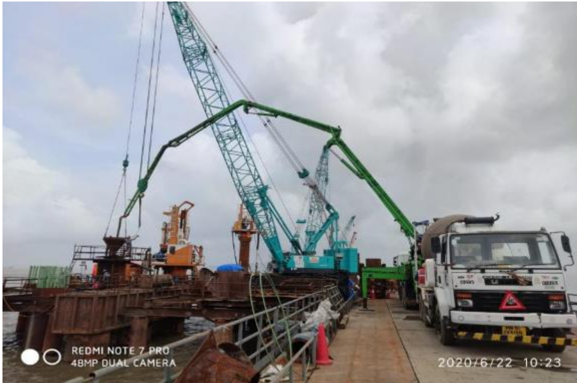
Photo No. 9: Pile concreting at MP 220/02 RHS in progress
