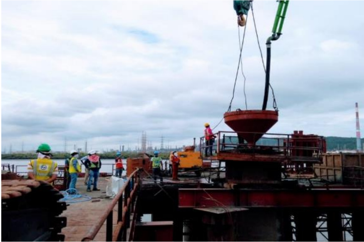
Photo No. 9: MP 44 S1 Pile Concreting – Intertidal in progress
