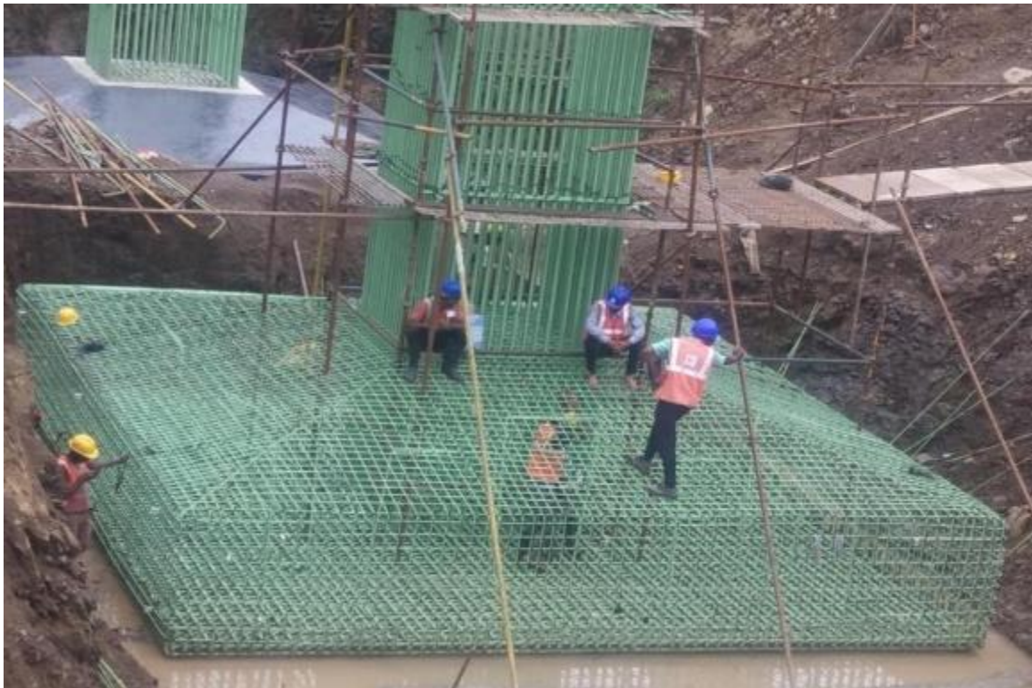
Photo No. 2: Chirle RP 01 LHS foundation reinforcement work is in progress
