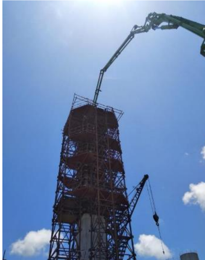
Photo No. 3: AP-44 Pier Final Lift Concreting in progress
