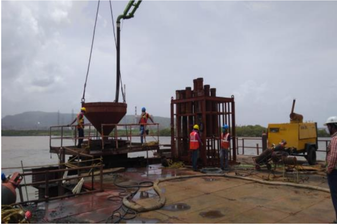
Photo No. 7:- MP 44 N1 Pile Concreting - Intertidal Section in progress
