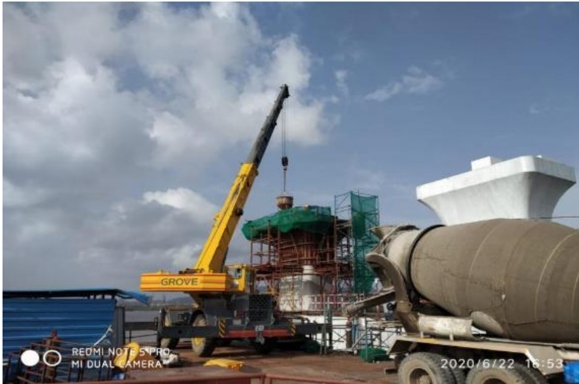
Photo No. 5: MP29 N Pedestal, Shear Key Concreting in progress
