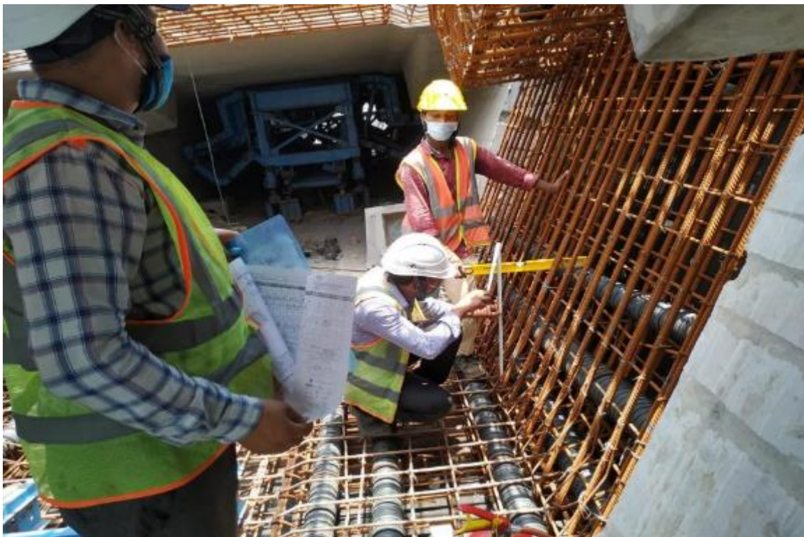
Photo No. 10: Segment Profile checking in progress
