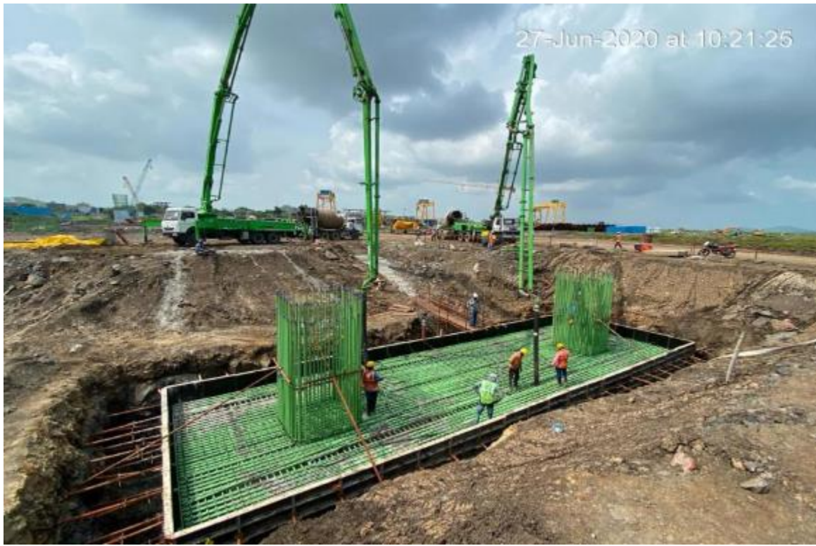
Photo No. 1: Concreting at Open Foundation MP 259 RHS in progress
