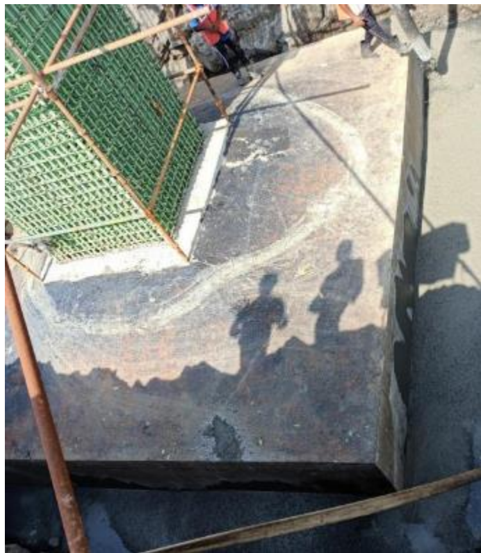
Photo No. 6: Annular filling at Foundation RP-33 LHS (Chirle) in progress
