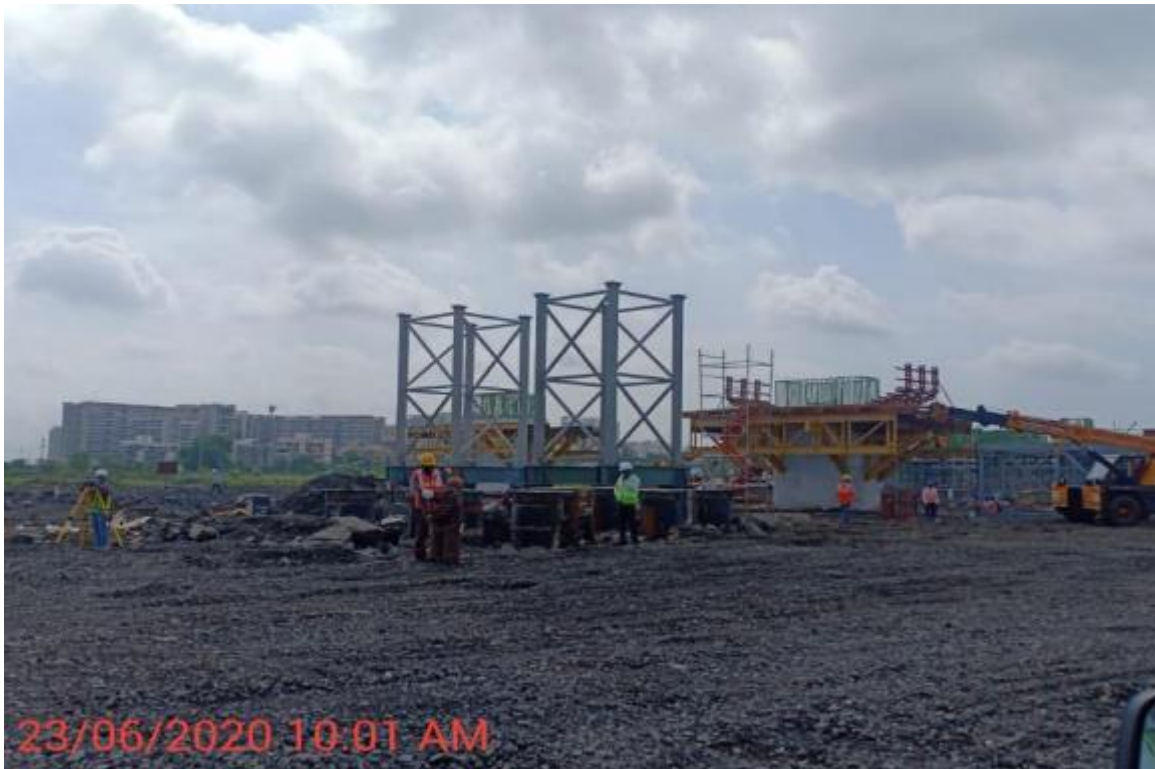
Photo No. 8: Frame erection for Launching Girder in progress
