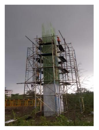
Photo No. 2: JMP-10 (Chirle) Pier reinforcement inspection completed
