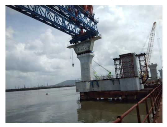
Photo No. 12: MP-19 N Pier Head Segment Erection - Intertidal Section in progress
