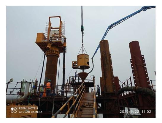
Photo No. 3: Pile concreting at MP 181 LHS in progress
