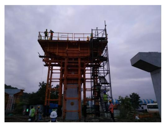
Photo No. 4: LP-06 (Jasai) Pier Cap Pre-pour inspection completed
