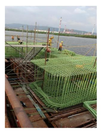
Photo No. 3: MP 43 Pile Cap Bottom Reinforcement Inspections - Intertidal in progress
