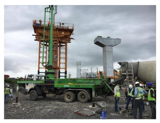
Photo No. 8: RMP 281 Pier Cap concrete pouring in progress
