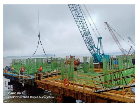
Photo No. 2: Pile Cap Reinforcement Works at MP 216 RHS in progress
