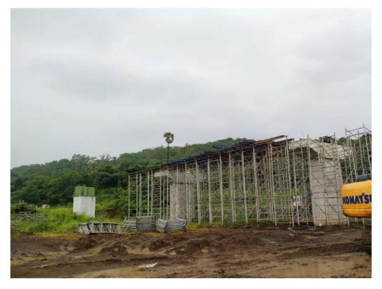
Photo No. 12: Staging Arrangement for Cast in-situ voided slab of span MJP-7 to 8 (Chirle) in progress
