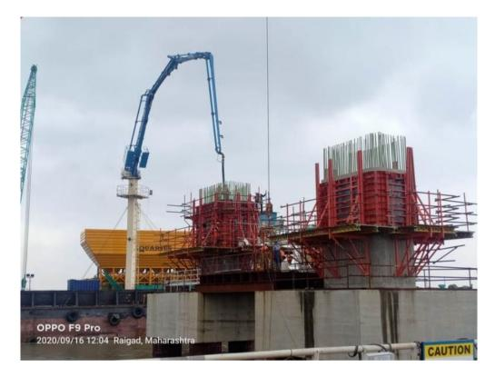
Photo No. 9: Pier final lift concreting at MP 206 RHS in progress
