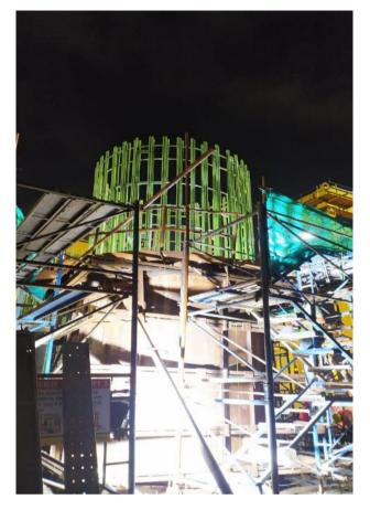
Photo No. 11: AP 39 Pile Cap concreting in progress
