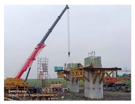
Photo No. 4: Pier Cap bottom formwork preparatory works at MP 241 LHS and RHS in progress
