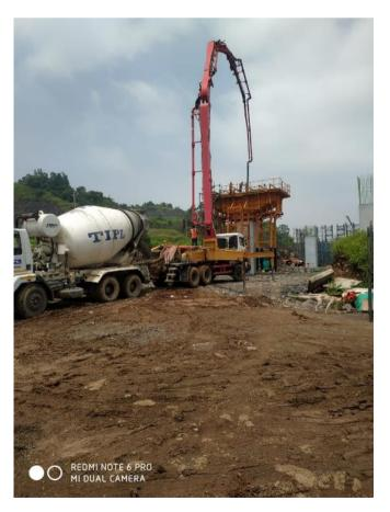
Photo No. 6: JMP02 (Jasai) Pier Cap concreting in progress
