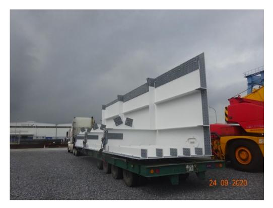
Photo No. 7: Transportation of OSD Girder Bridge P1-OS01-NG Package to Port for Shipment-3 in progress
