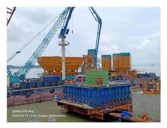
Photo No. 11: Pile Cap concreting at MP 212 RHS in progress
