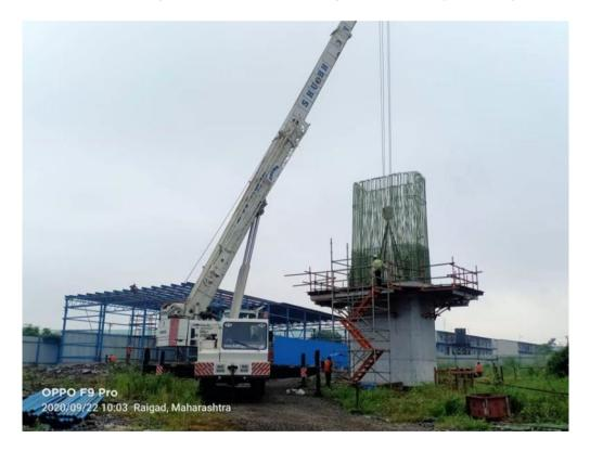
Photo No. 6: Pier Formwork fixing at MP 265 LHS in progress
