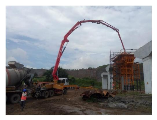
Photo No. 5: LP06 Pier cap concrete pouring in progress
