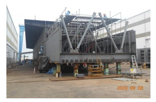
Photo No. 6: Trial Assembly of OSD Girder Bridge P1-OS04-NG (Lot6) / Seg. 28~32 in Vietnam in progress
