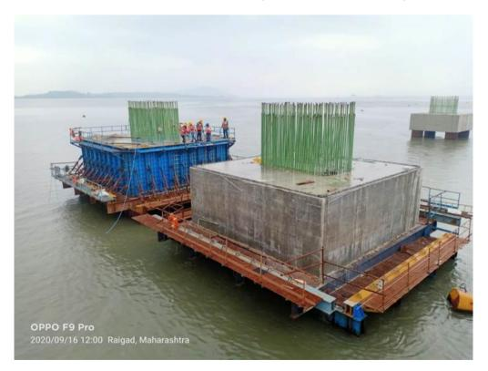
Photo No. 10: Pile Cap curing Works at MP 212 LHS and RHS in progress
