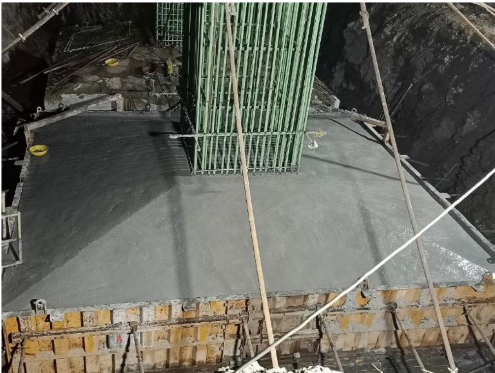
Photo No. 2: Foundation RP-23 RHS (Jasai) concreting done
