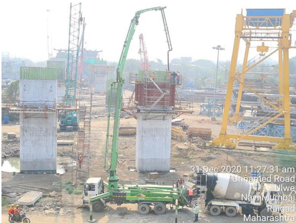
Photo No. 2: Pier final lift concreting at MP 263 RHS in progress
