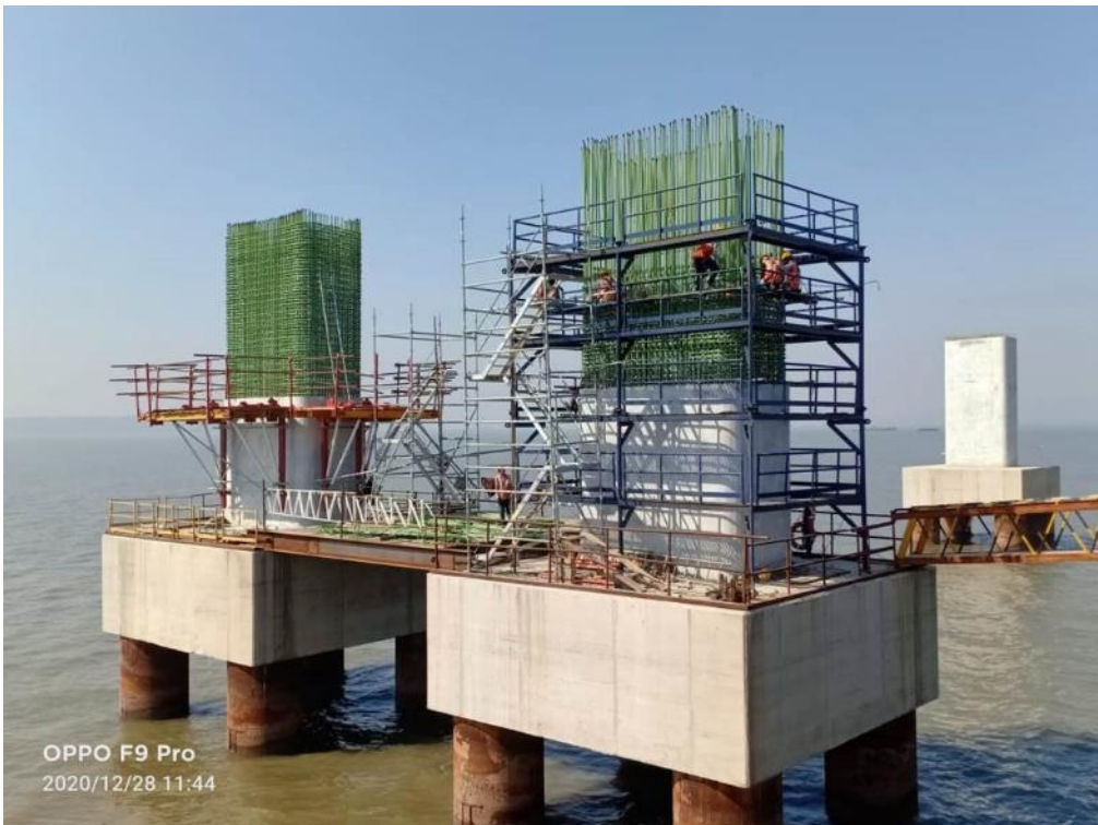
Photo No. 6: Pier reinforcement tying at MP 212 LHS in progress
