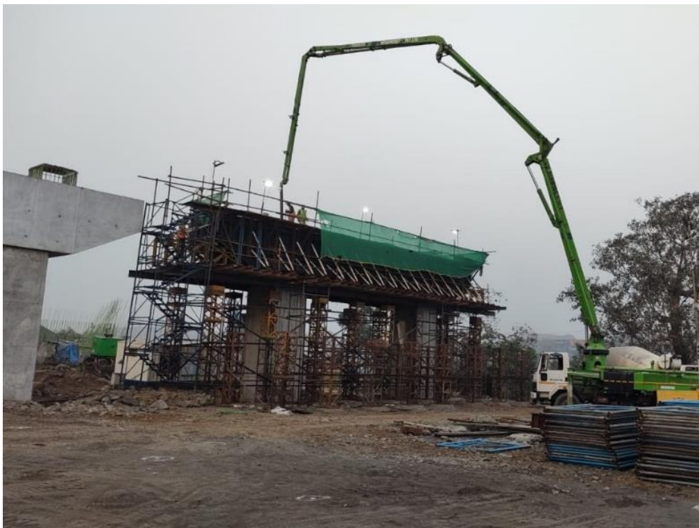
Photo No. 6: LP01 portal cap concrete pouring work in progress
