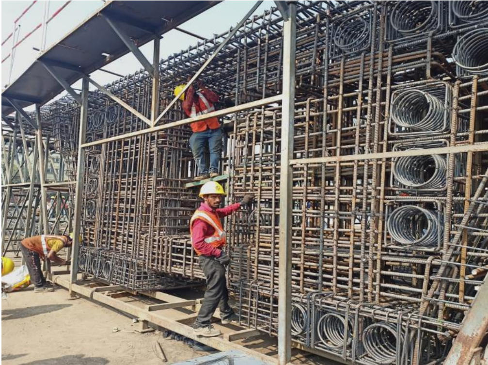
Photo No. 7: MP27-28 SS01 Reinforcement Checking Completed
