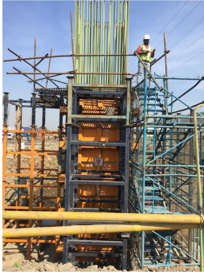
Photo No. 3: Pier No. RP33 RHS coordinates & formwork checking in progress
