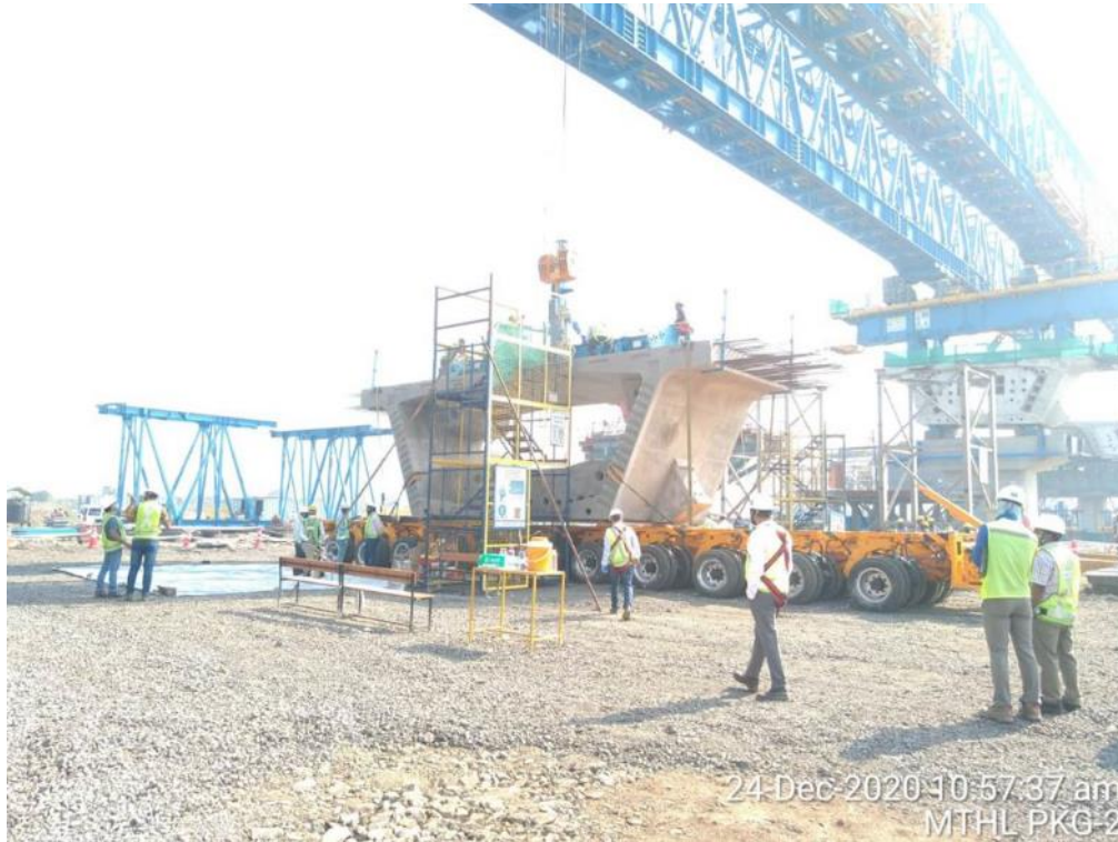
Photo No. 11: Preparatory works for LG Load Testing in progress
