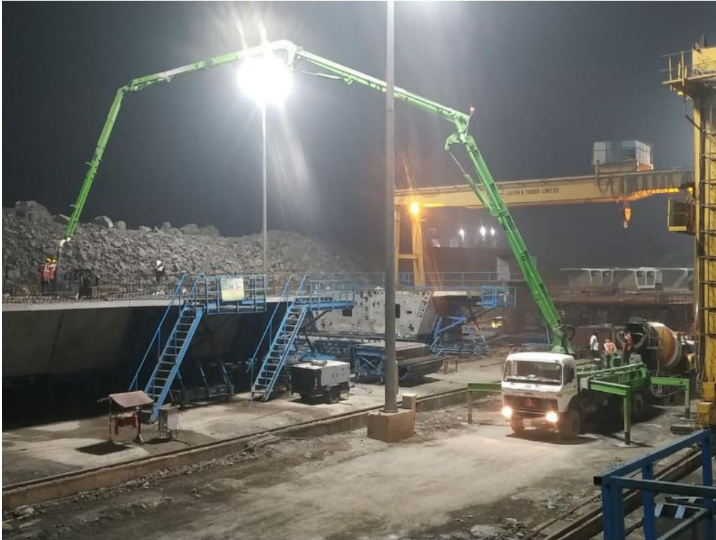
Photo No. 11: Bay 2, Segment Y-53, Span RMP 280-281 concrete pouring in progress
