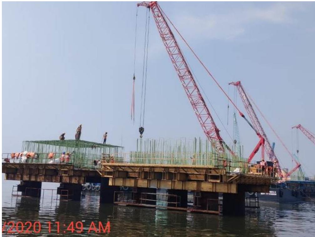
Photo No. 8: Pile cap reinforcement tying at MP 191 LHS in progress
