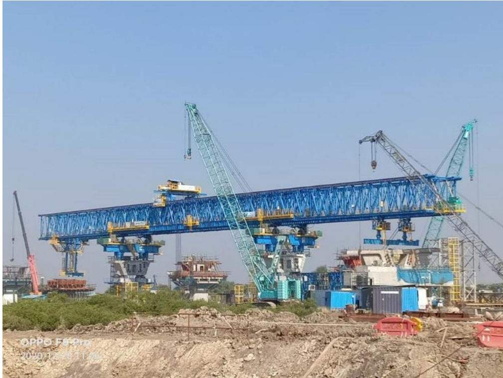
Photo No. 7: Electrification works of LG in progress
