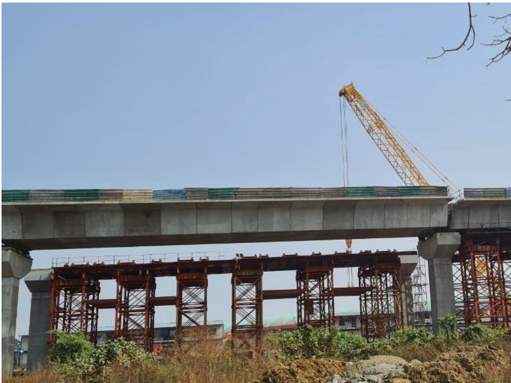
Photo No. 12: Segment Span RMP 267- 268- 269 erection in progress
