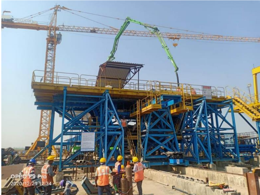
Photo No. 3: Segment concreting at Bay-1 in progress
