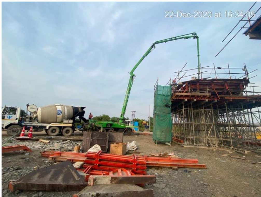
Photo No. 12: Pier cap concreting at MP 242 LHS in progress
