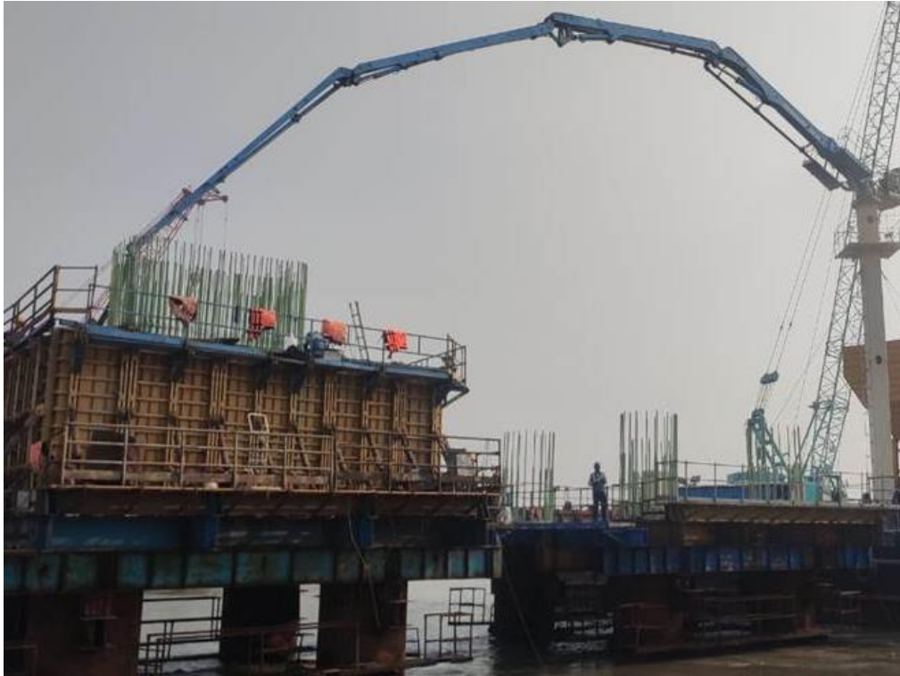
Photo No. 1: Pile cap concreting at MP 189 LHS in progress
