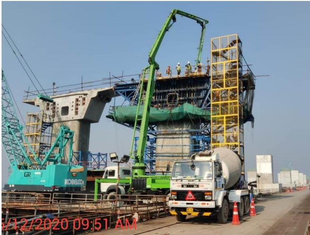
Photo No. 9: Pier head segment concreting at MP 233 LHS in progress
