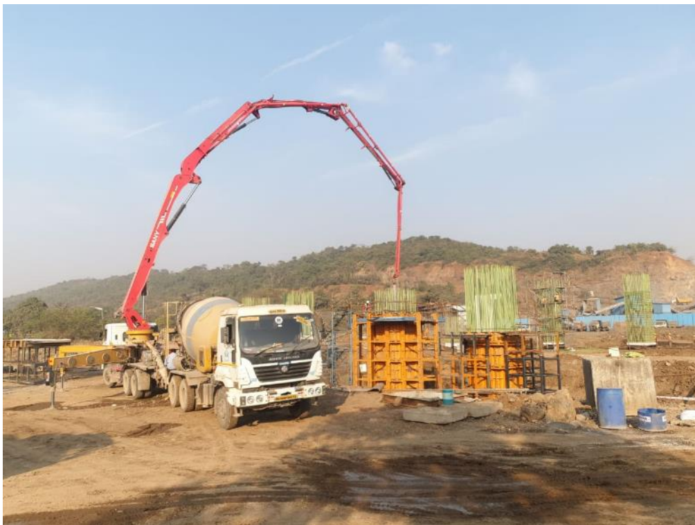
Photo No. 4: RP 37 LHS 1st lift (6m) concrete pouring in progress
