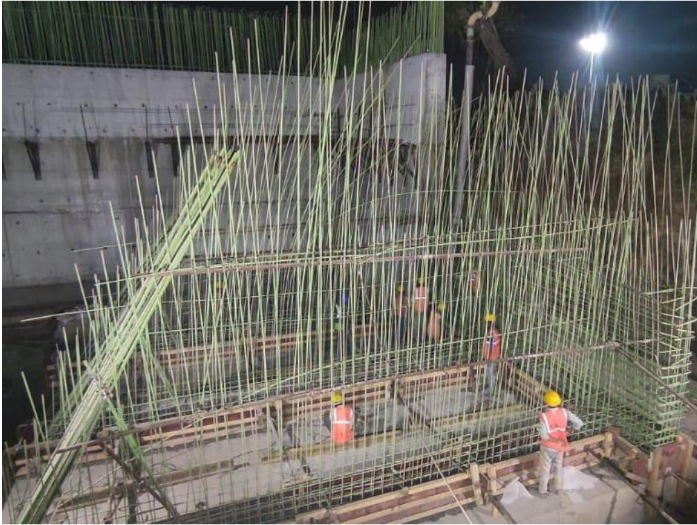
Photo No. 1: LMP A2 Retaining wall concrete pouring in progress
