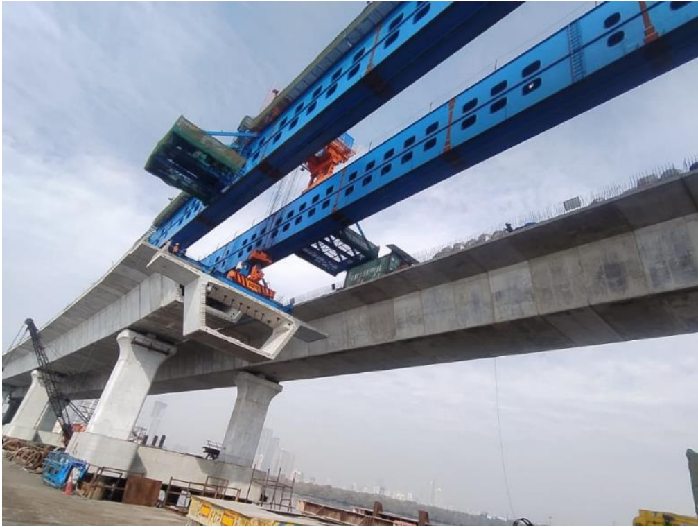
Photo No. 1: LG -1 & LG-2 - Segment Erections - Intertidal Section in progress
