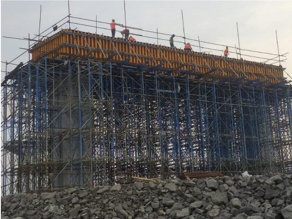
Photo No. 7: LMP 279 Portal Cap Formwork in progress
