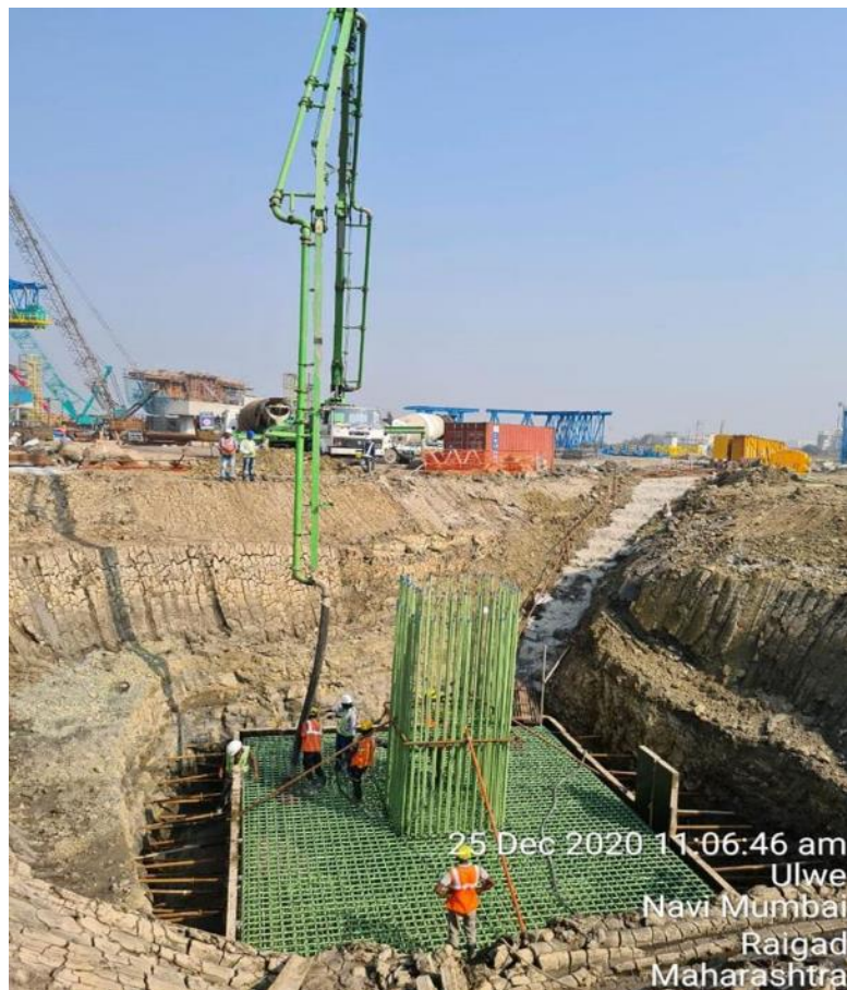
Photo No. 10: Portal Beam reinforcement tying at MP 249 RHS in progress
