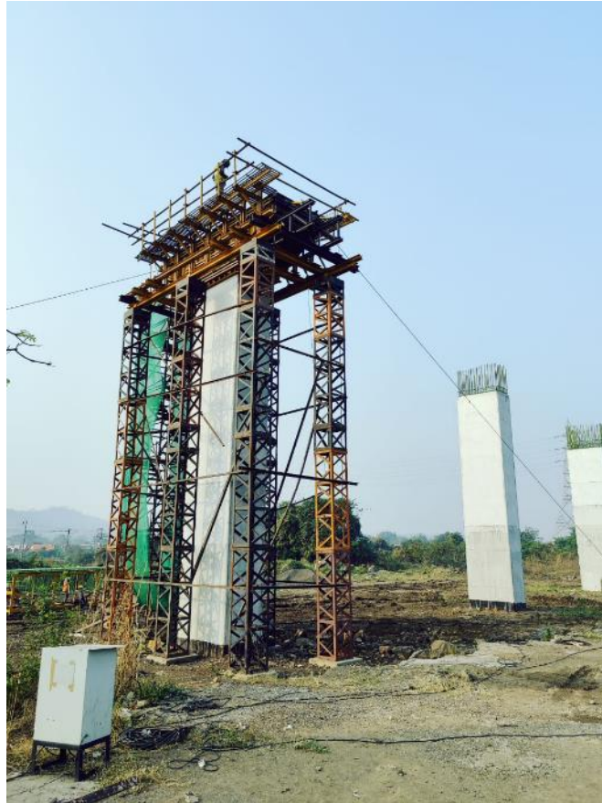
Photo No. 5: MPP-11 (Chirle) Pier Cap pre-pour inspection in progress
