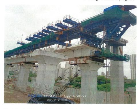
Photo No. 2: LG-7 Installation LPN3-LPN4 - Interchange Section in progress
