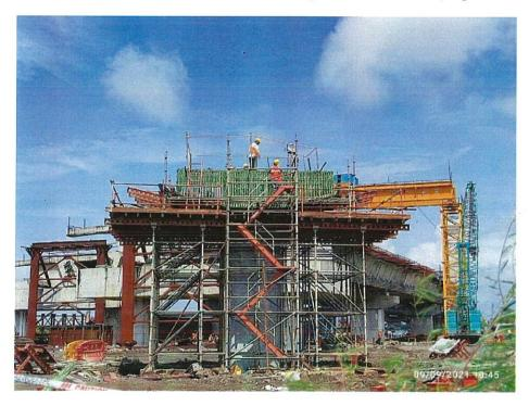
Photo No. 10: Pier cap reinforcement tying at MAP-1 in progress
