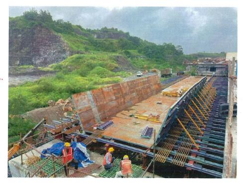
Photo No. 12: Span JMP 01-02 (SH-54 Ramp) CIS single cell box girder Bottom soffit work
