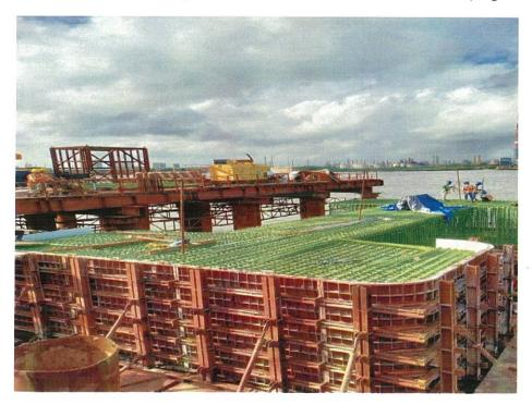
Photo No. 8: MP63 Pile Cap Shuttering Work - Intertidal Section in progress
