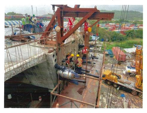
Photo No. 2: Span LP 04-05, 1st stage prestressing work in progress
