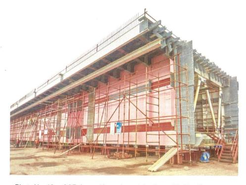
Photo No. 12: - OSD Assembly works - at the Assembly Yard in progress
