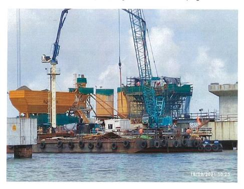
Photo No. 8: Pier cap concreting at MP 201 RHS in progress
