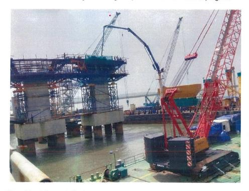
Photo No. 4: Integral Pier head segment concreting at MP 212 RHS in progress
