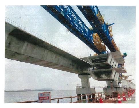
Photo No. 3: LG-2 Segment lifting at Span MP 231-232 LHS in progress
