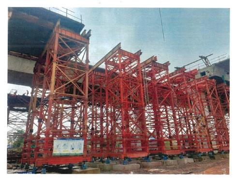
Photo No. 3: Span LMP 281-282 under slung trestle & soffit erection work in progress
