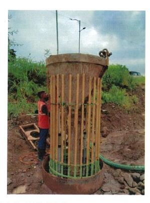
Photo No. 7: Pile RP34/3 concrete pouring in progress
