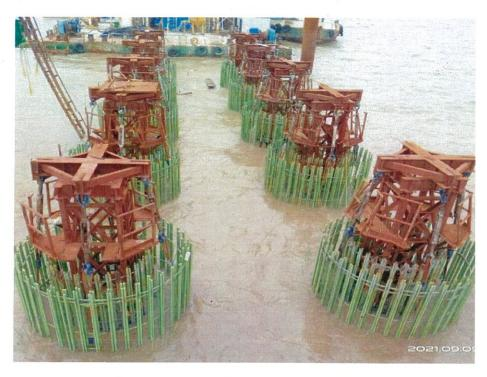
Photo No. 9: OSD MP 70 Protection Ring Lowering - Intertidal Section Completed
