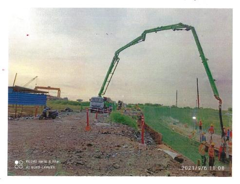
Photo No. 12: Retaining wall raft concreting at Ramp AC in progress
