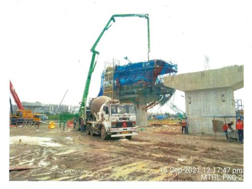
Photo No. 9: Pier head segment concreting at MP 246 LHS in progress
