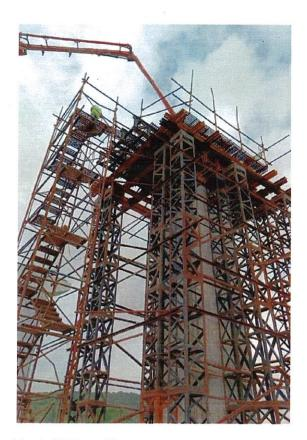
Photo No. 9: MPP 09 Pier Cap concrete pouring in progress
