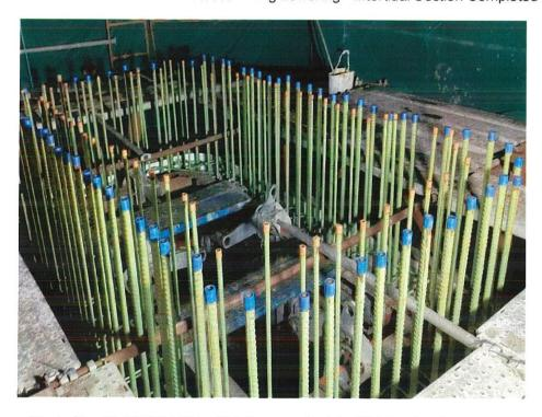
Photo No. 10: MP 58 N Pier Reinforcement - Intertidal Section in progress
