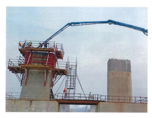
Photo No. 11: Pier lift concreting at MP 198 RHS in progress
