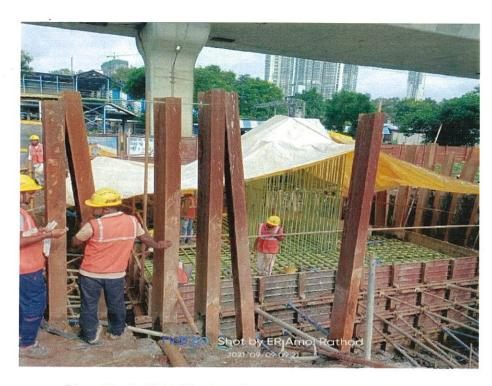
Photo No. 3: EP08 Pile Cap - Interchange Section in progress
