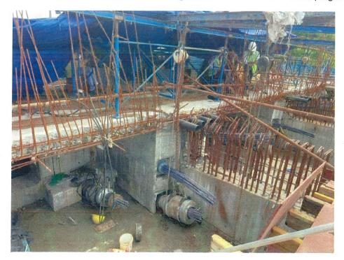
Photo No. 4: 1st stage prestressing work at CIS Span RP 03-02 in progress
