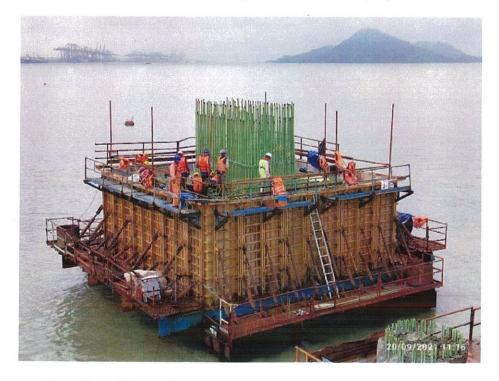
Photo No. 6: Pile cap formwork alignment at MP 160 RHS in progress
