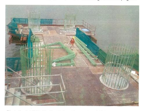
Photo No. 6: MP 65 Pile Cap Bottom Shutter - Intertidal Section Completed
