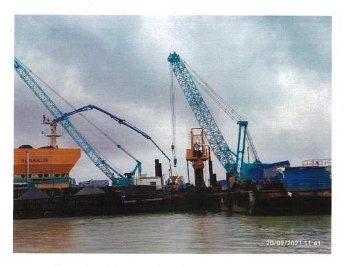
Photo No. 5: Pile concreting at MP 176 RHS in progress
