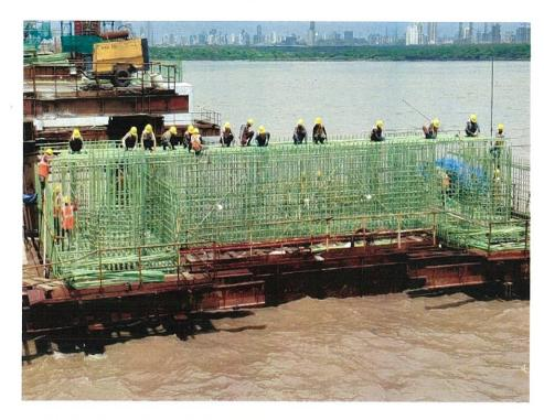
Photo No.7: MP 60 Pile Cap Reinforcement Work - Intertidal Section in progress
