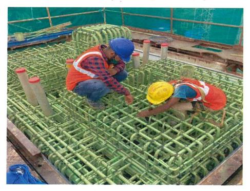
Photo No. 4: AP58 Pier Head Reinforcement - Interchange Section in progress
