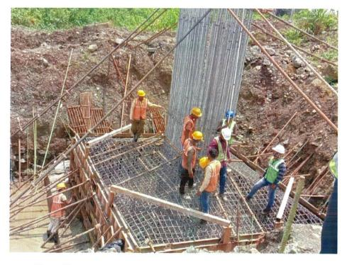
Photo No. 6: Foundation RP 27 R pre-pour inspection in progress
