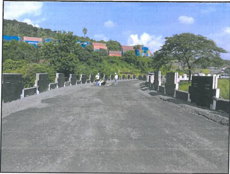
Photo No. 9: Chirle MJP Loop FDD inspection works in progress
