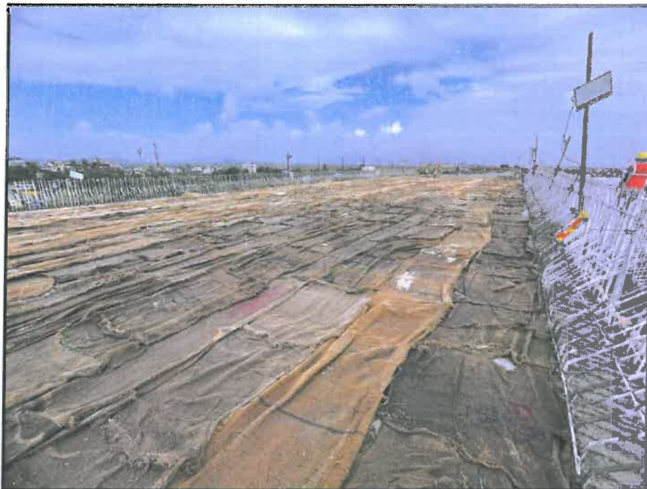
Photo No. 6: Gavan ROB span RMP 274-275 deck concrete completed
