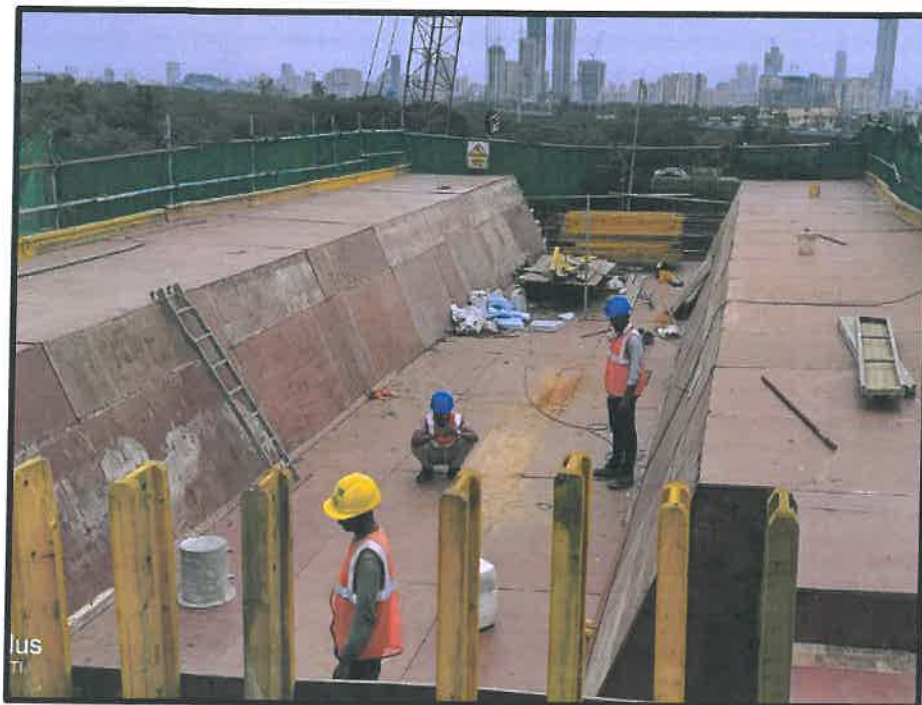
Photo No. 5: BP 33 Cast in situ Shutter Checking
