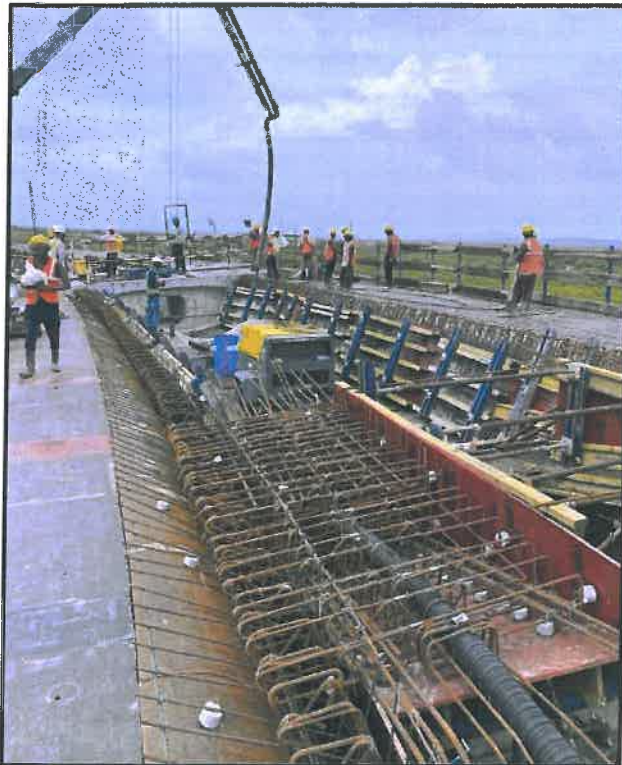
Photo No. 12: Web concrete at Ramp JM in progress
