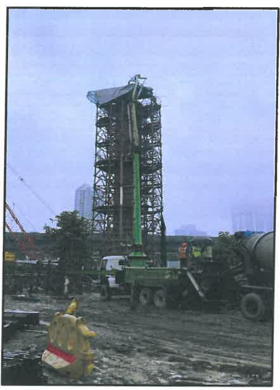
Photo No. 7: AP 35 Pier cap casting in progress
