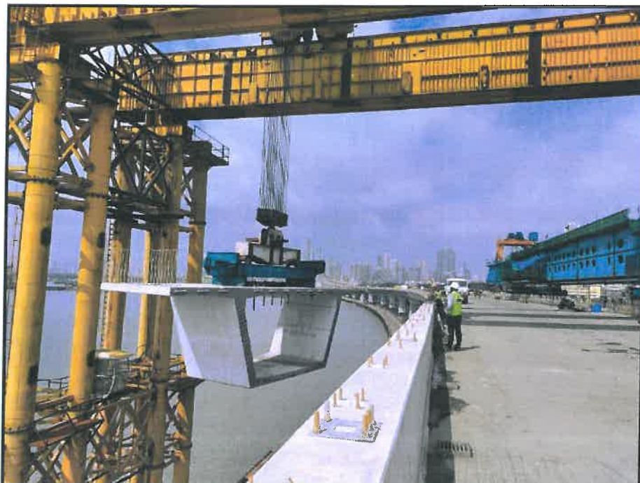
Photo No. 9: MP 13 gantry lifting segment in progress
