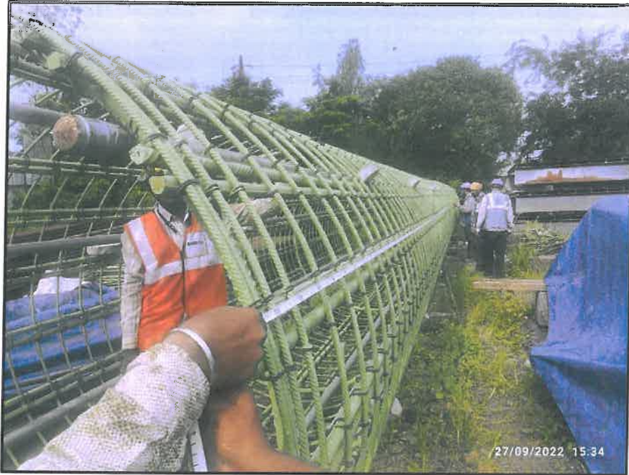
Photo No. 5: Pile reinforcement cage inspection at MP 240 R Substation in progress
