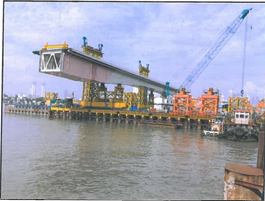
Photo No. 2: OSD 2 SPAN 1SOUTH MP 69-70 loading out in progress
