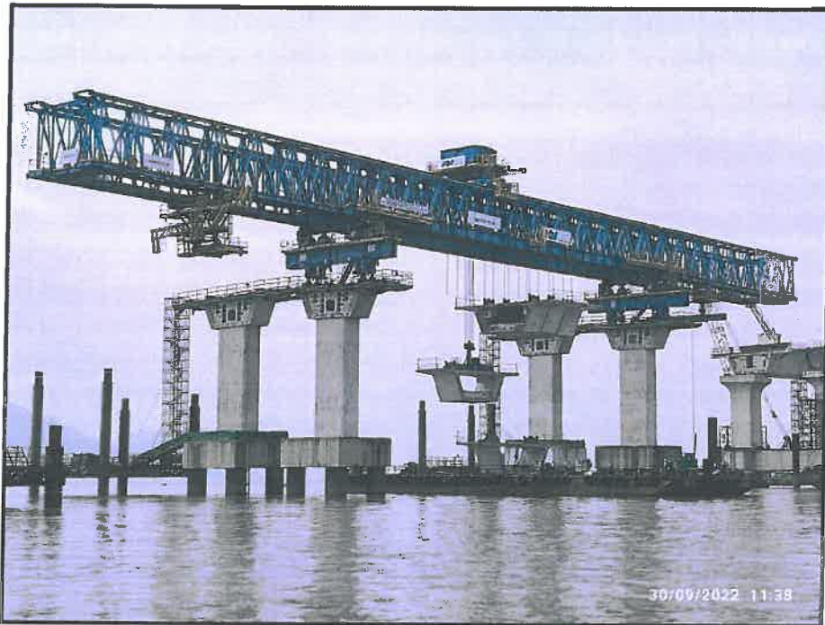
Photo No. 1: LG-1 Load Testing at MP 148A- MP 148B LHS in progress
