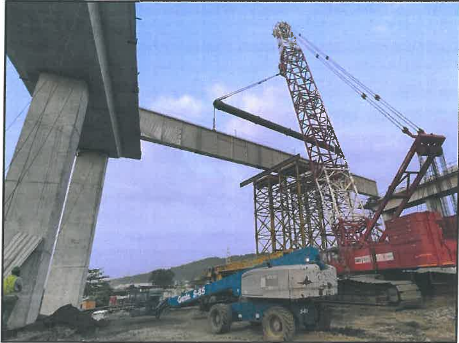
Photo No. 11: Jasai ROB Span LP25-26 Girder's Erection works in progress
