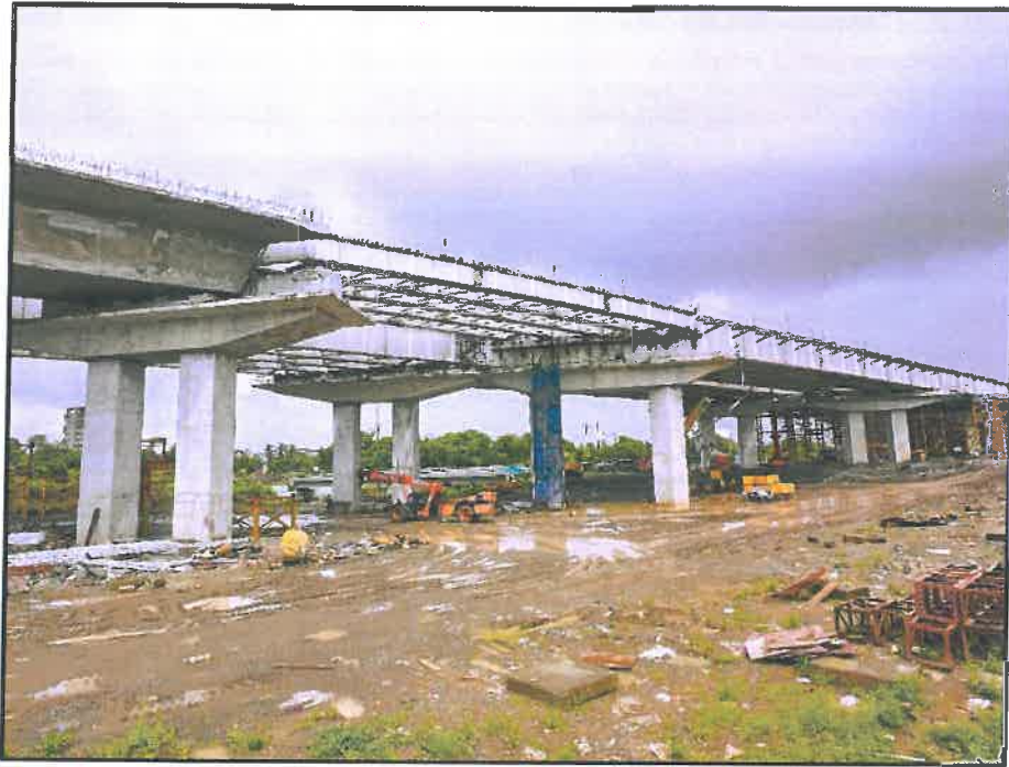
Photo No. 1: Gavan ROB structural works in progress
