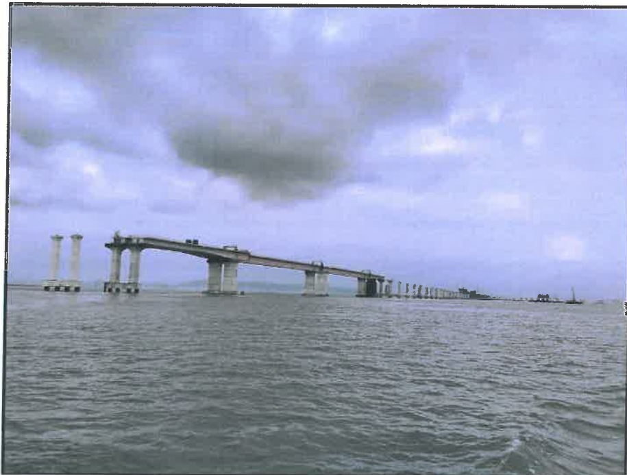
Photo No. 3: A view of erected OSD -4 Span
