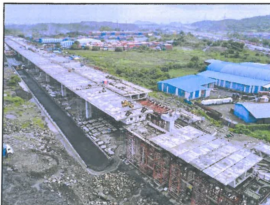
Photo No. 4: Jasai viaduct works in progress
