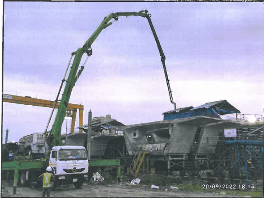
Photo No. 11: Segment concreting at Bay-1 in progress
