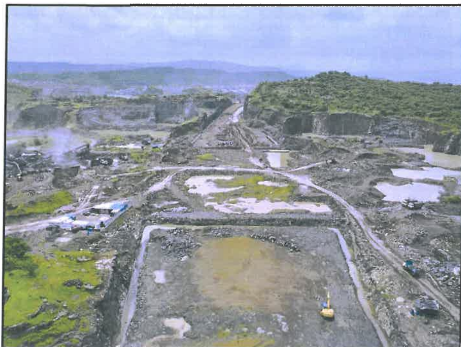
Photo No. 3: Toll-plaza area ground clearance works in progress
