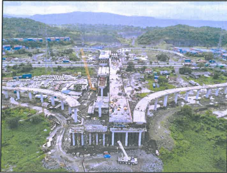
Photo No. 5: Chirle Interchange works in progress
