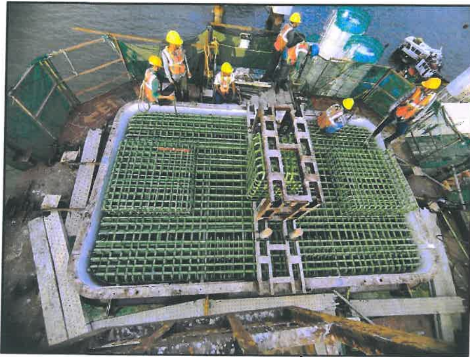
Photo No. 4: MP 113 S Pier Head Shuttering
