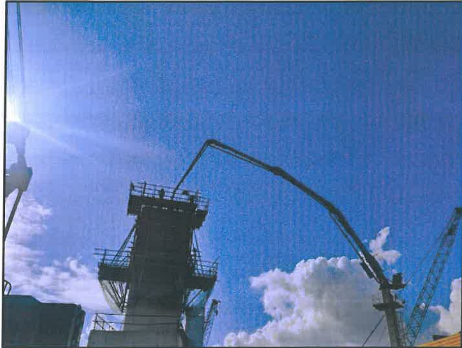
Photo No. 7: Pier 1st lift concrete at MP 174 RHS in progress
