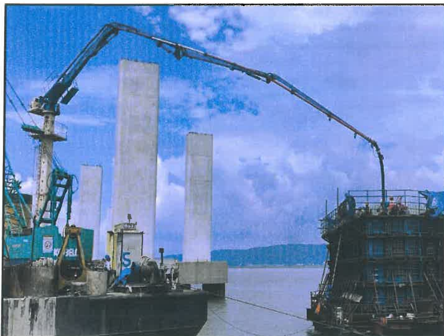
Photo No. 8: Pile cap concrete at MP 171 LHS in progress
