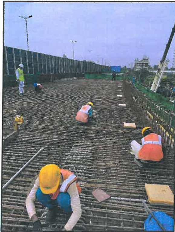
Photo No.8: EP 08-09 Top slab Cast in situ reinforcement in progress
