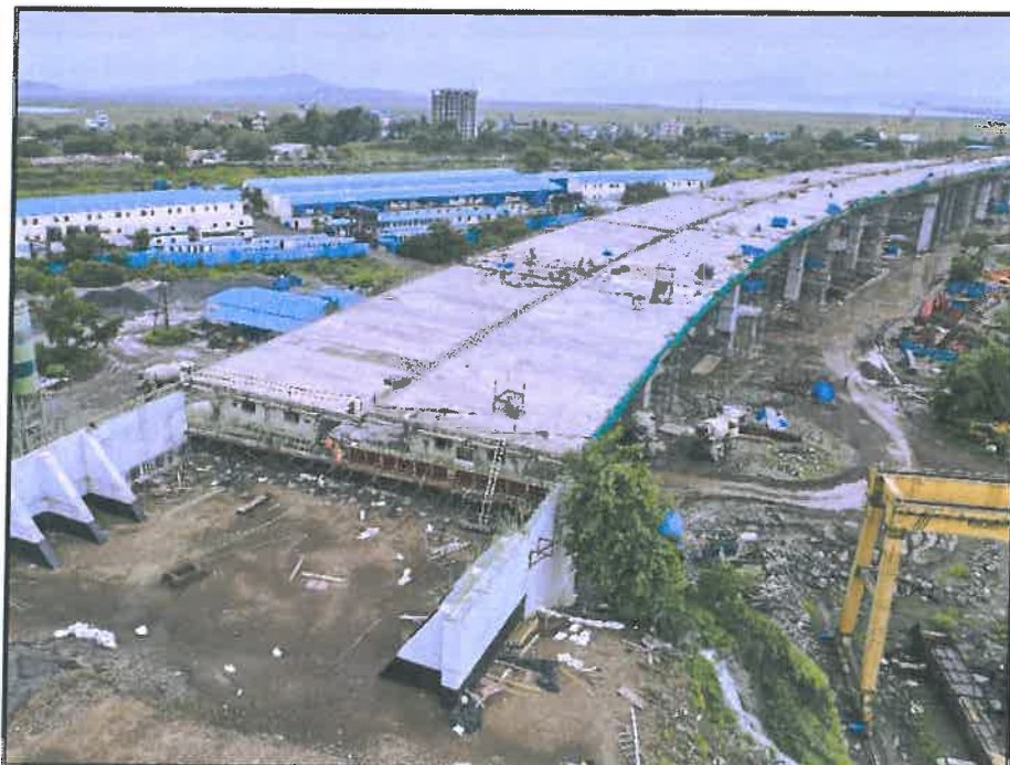
Photo No. 2: Gavan superstructure works in progress
