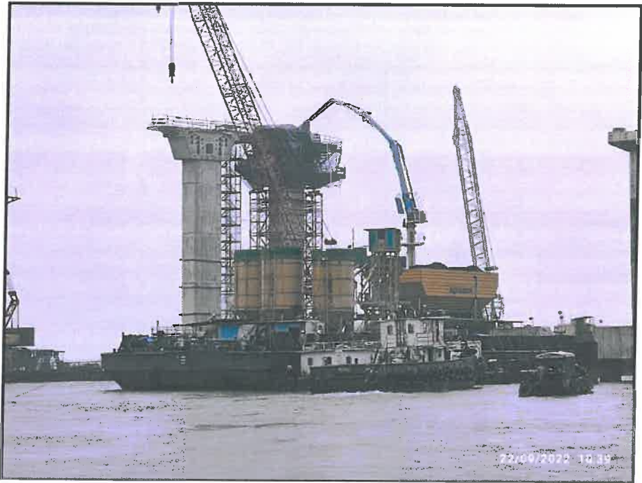
Photo No. 9: Integral pier head segment concrete at MP 190 LHS in progress
