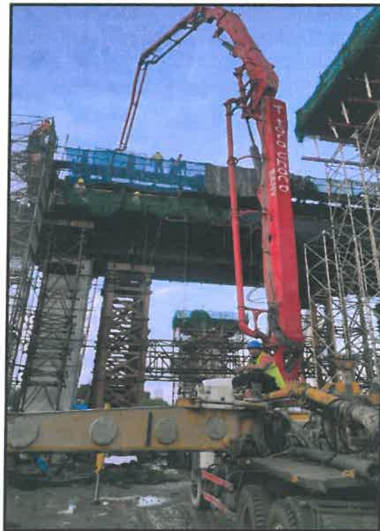
Photo No. 11: BP 33 portal pier cap casting in progress
