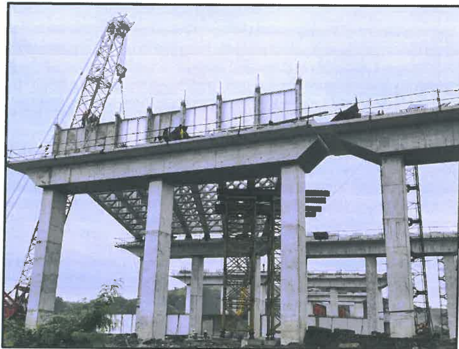
Photo No. 10: Jasai ROB Span RP26-27 Girder's Erection completed
