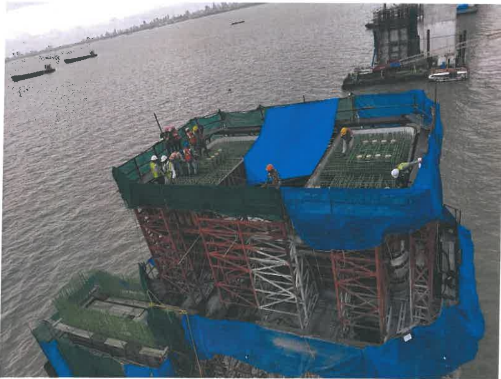
Photo No. 3: MP 72 Pier Head Shutter Checking in progress
