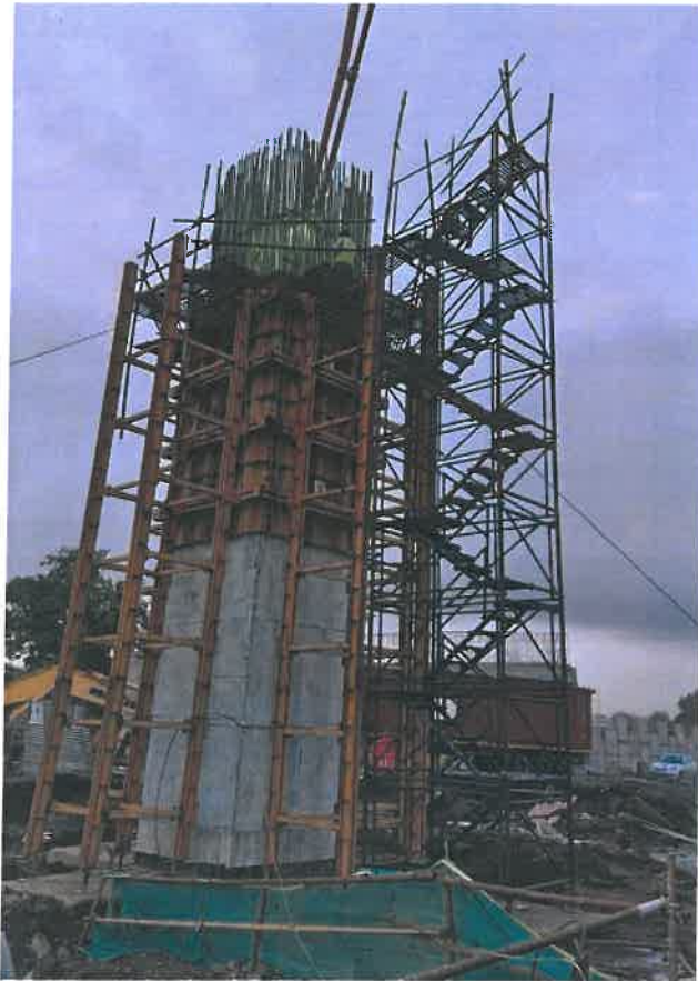
Photo No. 11: Jasai LP-20, Pier 3rd lift concrete work
