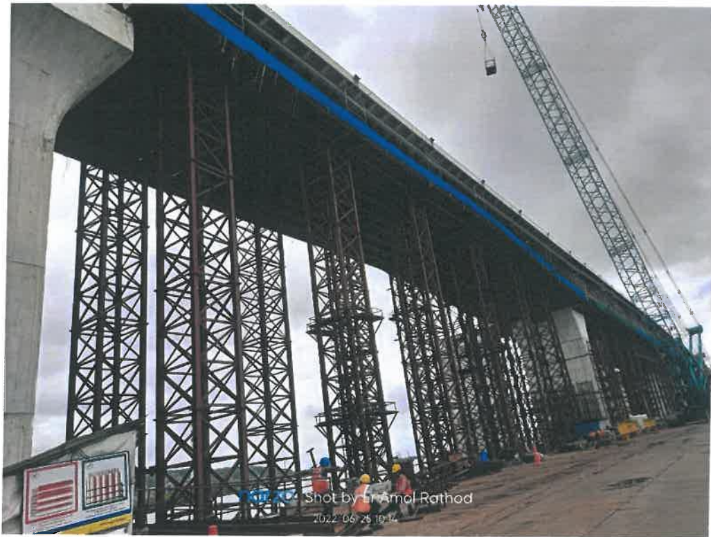
Photo No. 5: OSD-1 Span Erection in Progress
