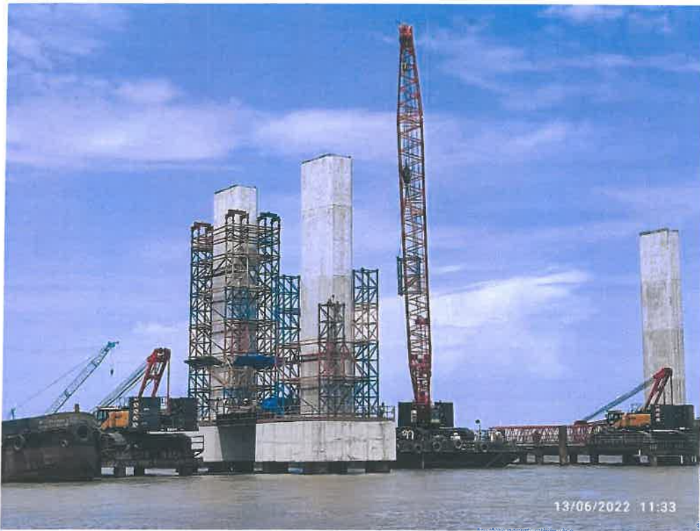
Photo No. 3: Integral pier head segment scaffolding at MP 188 RHS and LHS in progress
