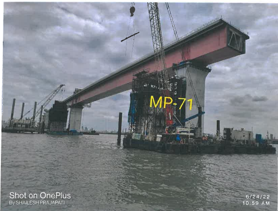
Photo No. 4: MP 71 OSD -2 Span towards Navi Mumbai
