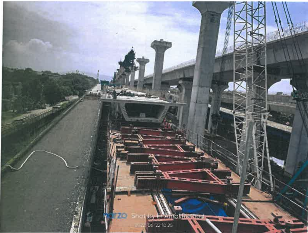
Photo No. 7: EP 15 Segments shifting for Erection in progress
