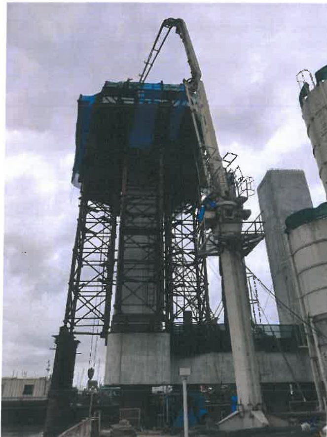
Photo No.8: AP 16 Pier Reinforcement in progress
