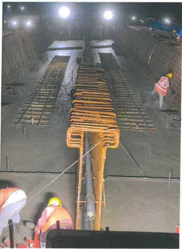
Photo No. 7: Gavan Span RMP 272-273, Soffit concrete casting completed
