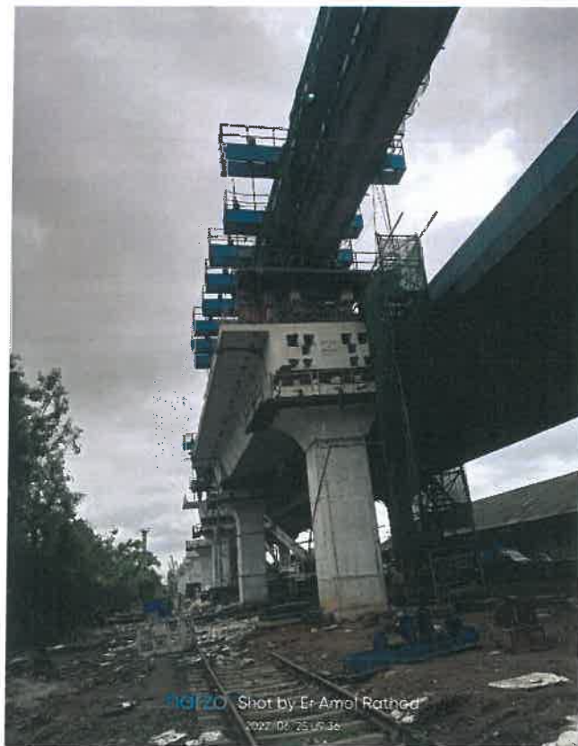
Photo No. 12: LG-06 AP 08-09 Span Erection in progress
