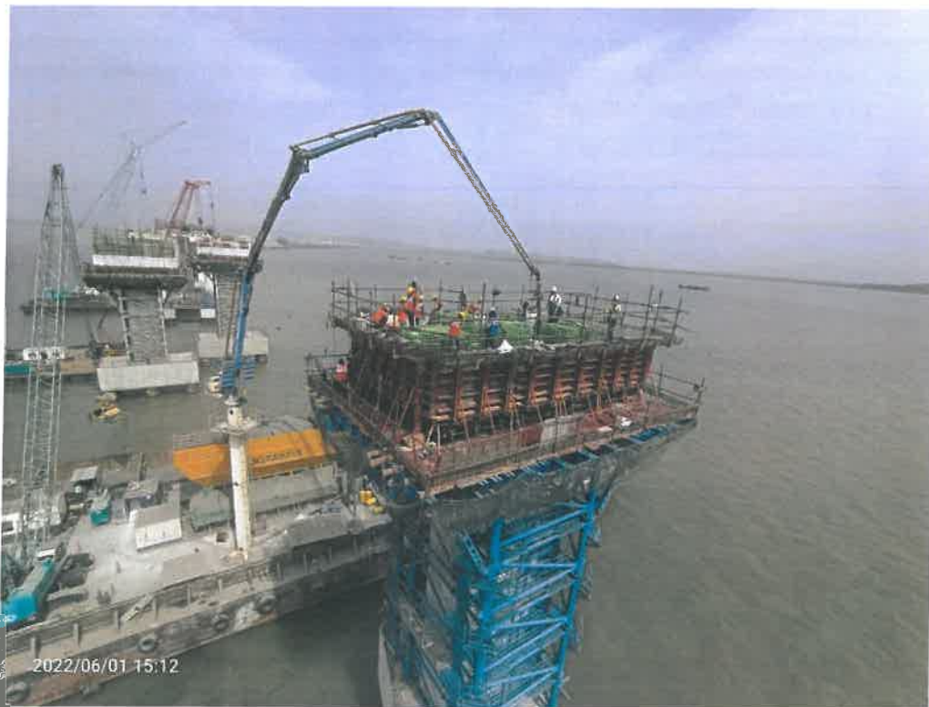
Photo No. 6: Pier cap concreting at MP 175 RHS in progress
