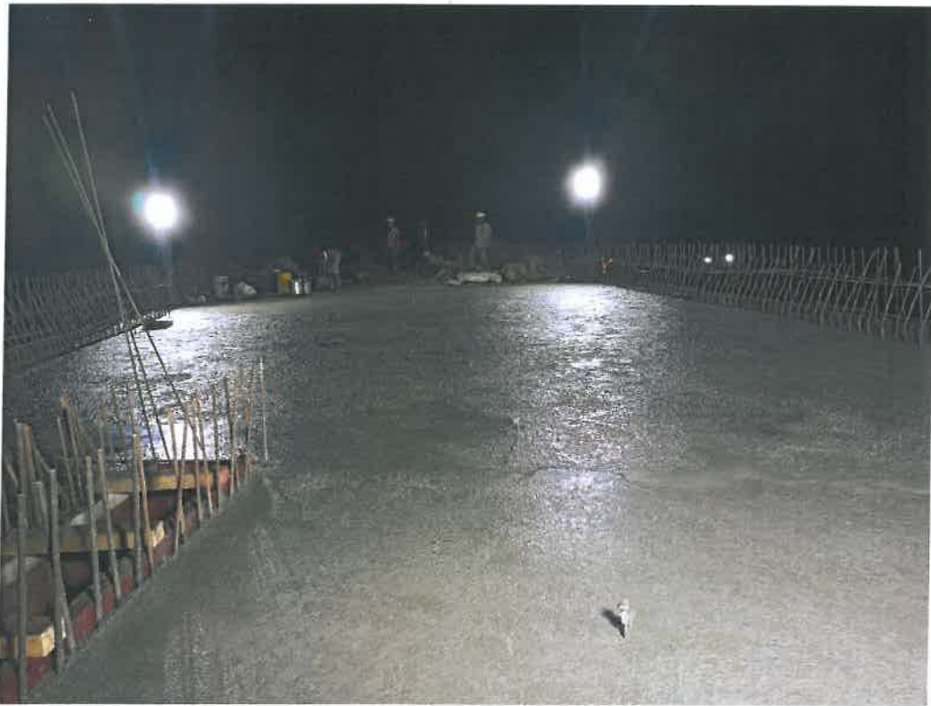
Photo No. 3: Chirle interchange ramp MJP1-2 voided slab concrete casting completed
