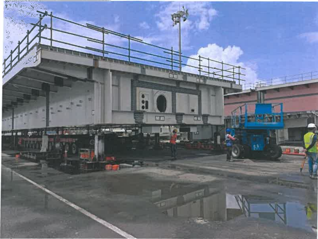
Photo No. 11: OSD works at Karanja Port in progress
