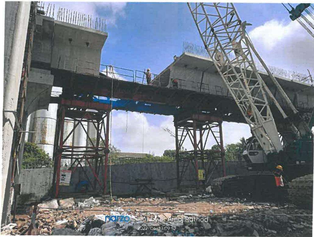
Photo No. 9: EP 15-16 Span Erection using Under Slung in progress
