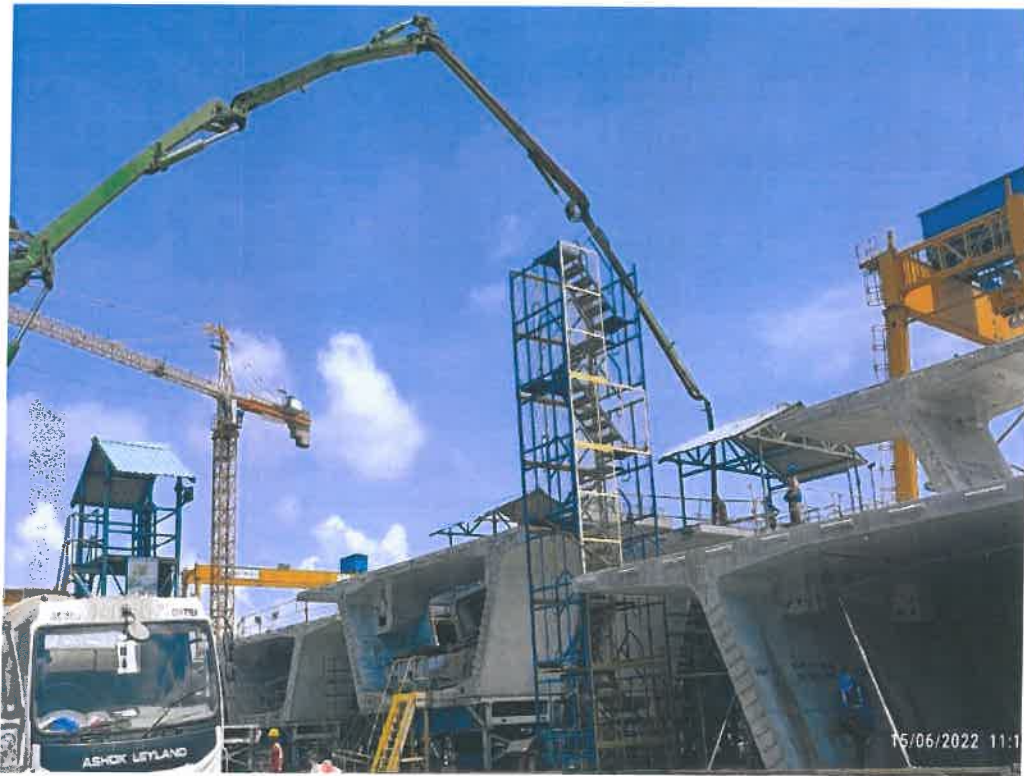
Photo No. 9: Segment concrete at Bay-1 in progress
