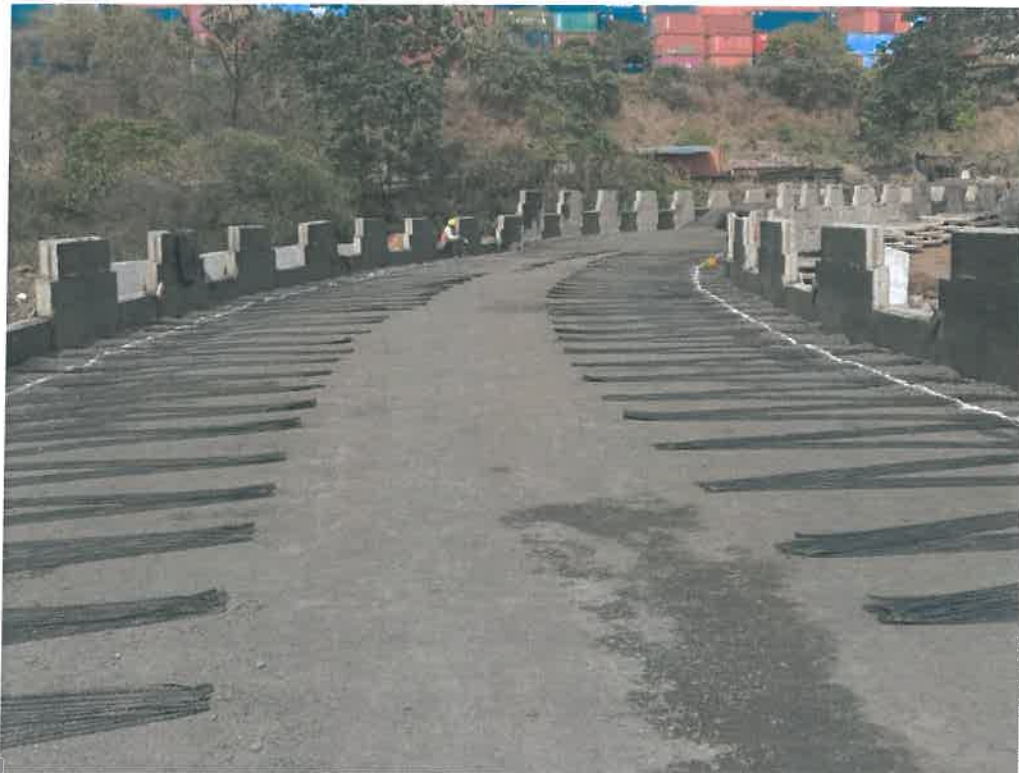
Photo No. 12: Chirle MJP Loop 2nd layer Geogrid work at CH 0+370 – CH 0+400
