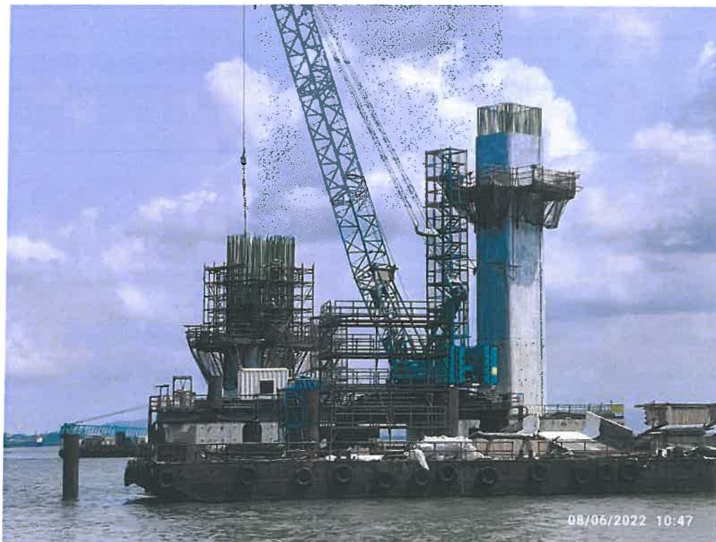
Photo No. 4: Pier reinforcement tying at MP 184 RHS in progress
