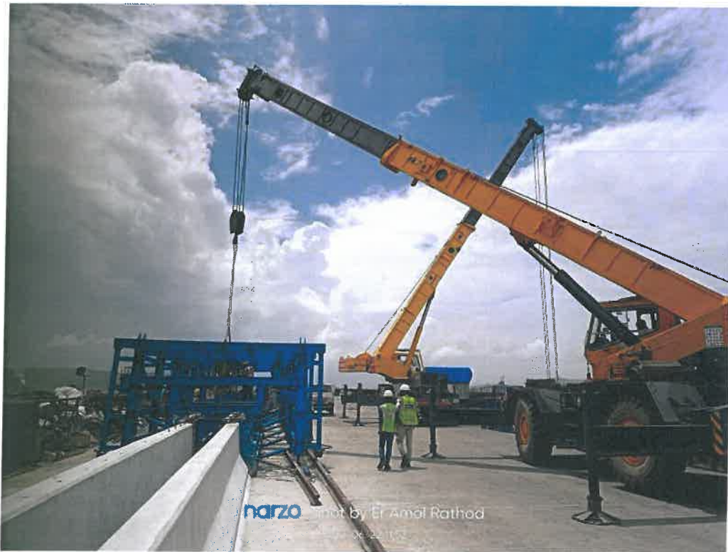
Photo No. 6: Ch. 1270 to 1290 Crash barrier Concrete Casting
