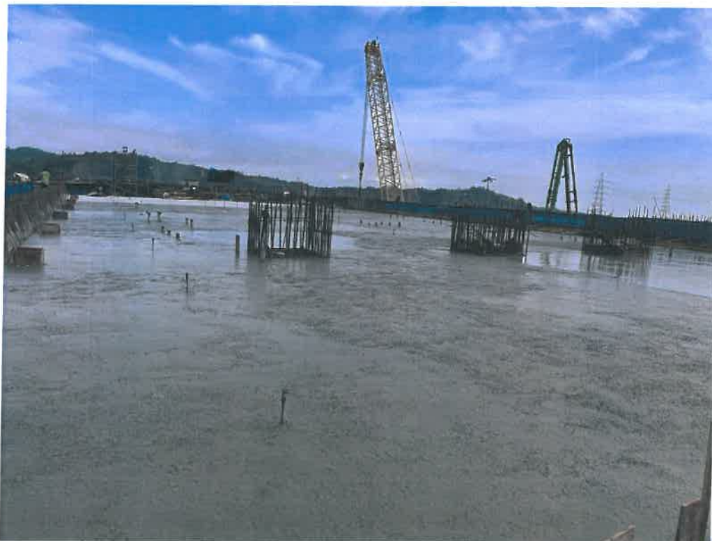
Photo No. 2: Chirle span RP33-34 Deck slab concrete casting completed
