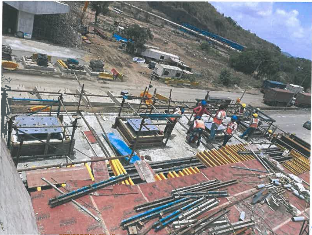
Photo No. 8: Chirle RP-35 Bearing installation survey work
