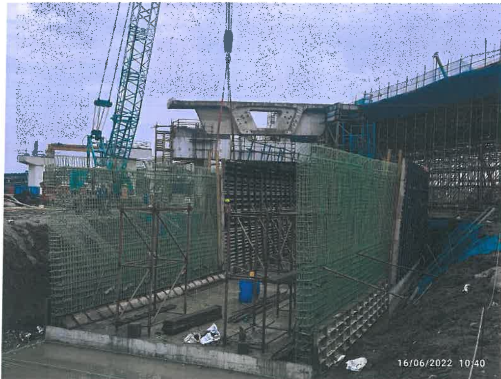
Photo No. 12: Retaining wall formwork fixing at Ramp CA in progress
