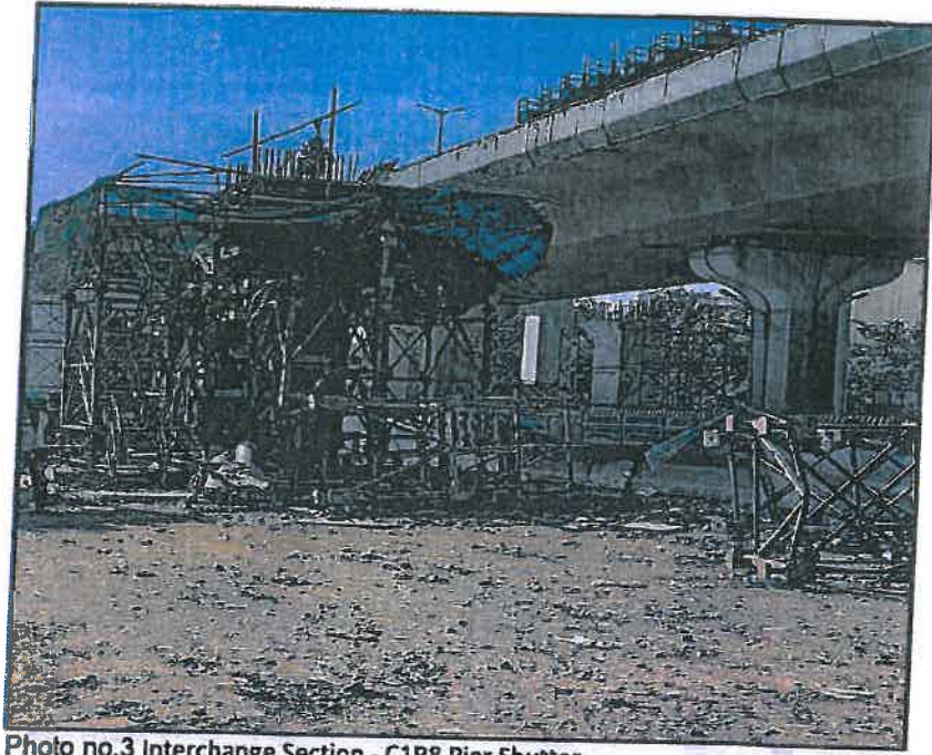
Photo no.3 Interchange Section - C1P8 Pier Shutter
