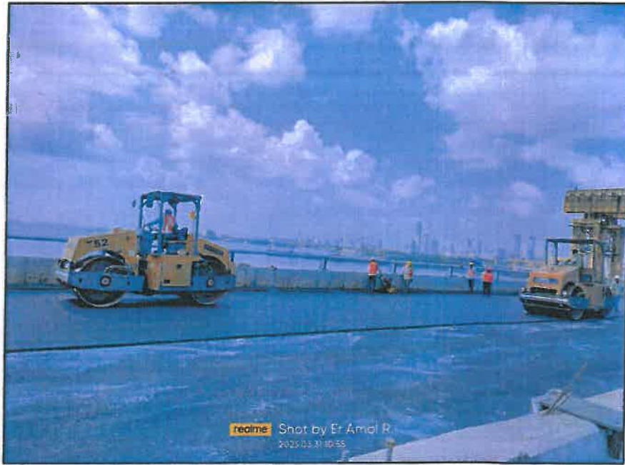
Photo no.3 Ch. 1290 SMA paving in progress
