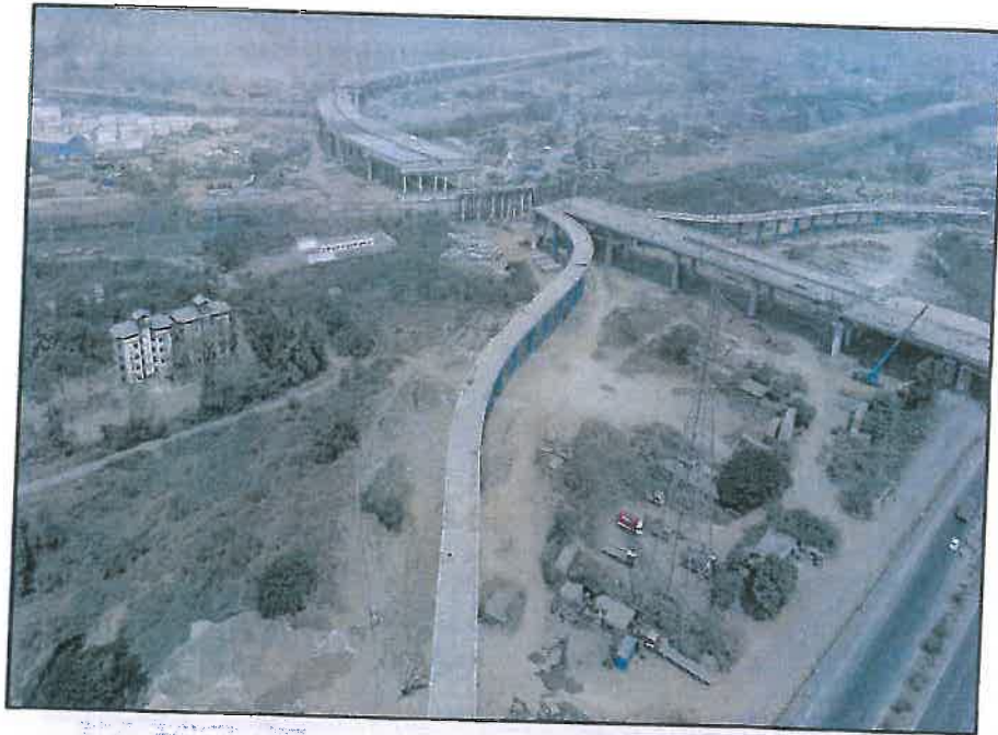
Photo no.9- JMP and MPP ramp at Chirle Interchange.
