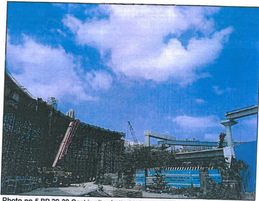
Photo no.5 BP 29-30 Cast in situ shuttering in progress
