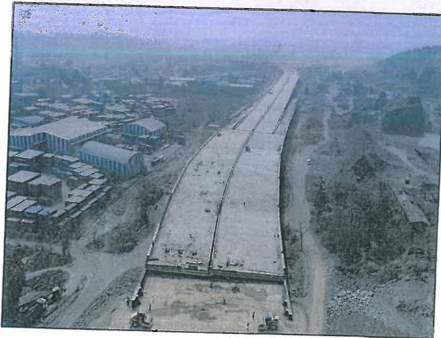
Photo no.10- Jasai Viaduct.
