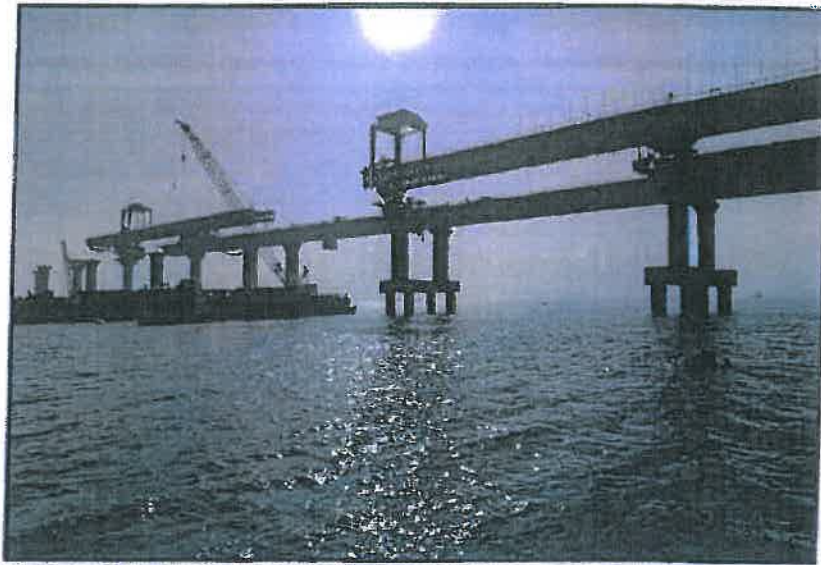
Photo no.9 Marine Section- LG-4 MP 104-105 N
