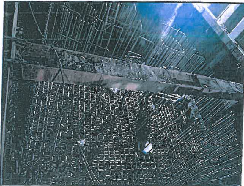
Photo no.2 Interchange Section - AP34 Pile Cap Reinforcement
