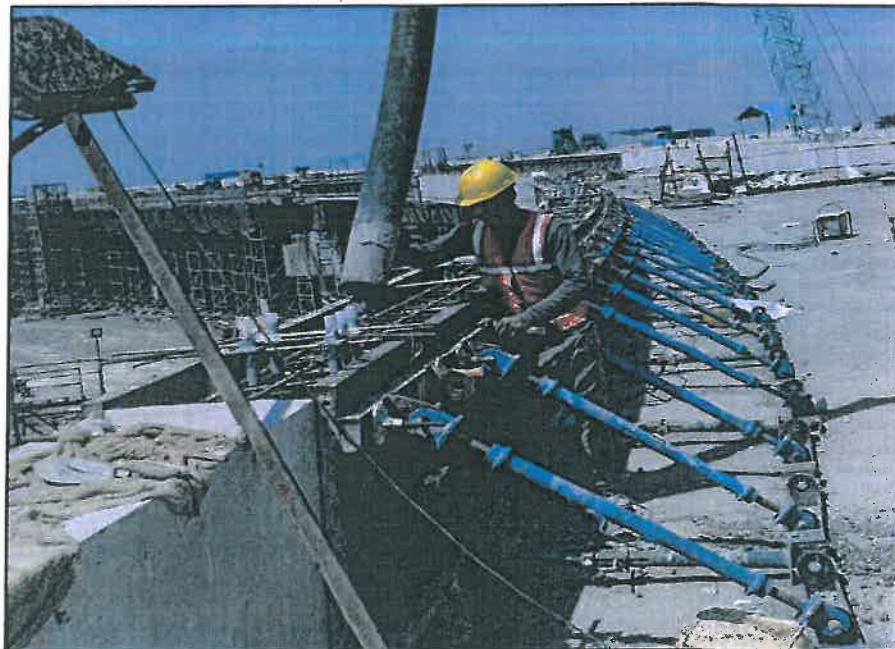
Photo no.4- Crash barrier concreting in progress at ramp AC.
