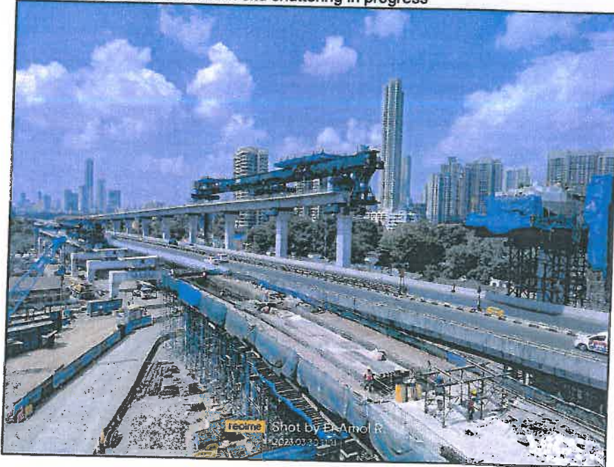
Photo no.6 Interchange view towards South Mumbai
