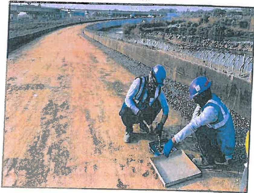
Photo no.6-Ramp AC – Soil compaction test in progress.
