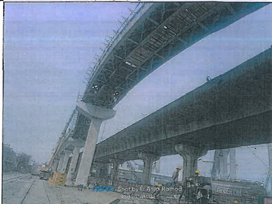
Photo no.4 Composite girder BP 24- BP 26
