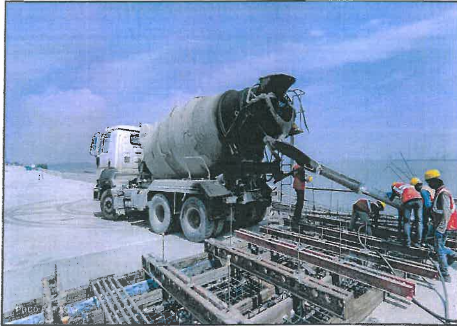
Photo no.3- Expansion Joint Cantilever slab concrete in progress.
