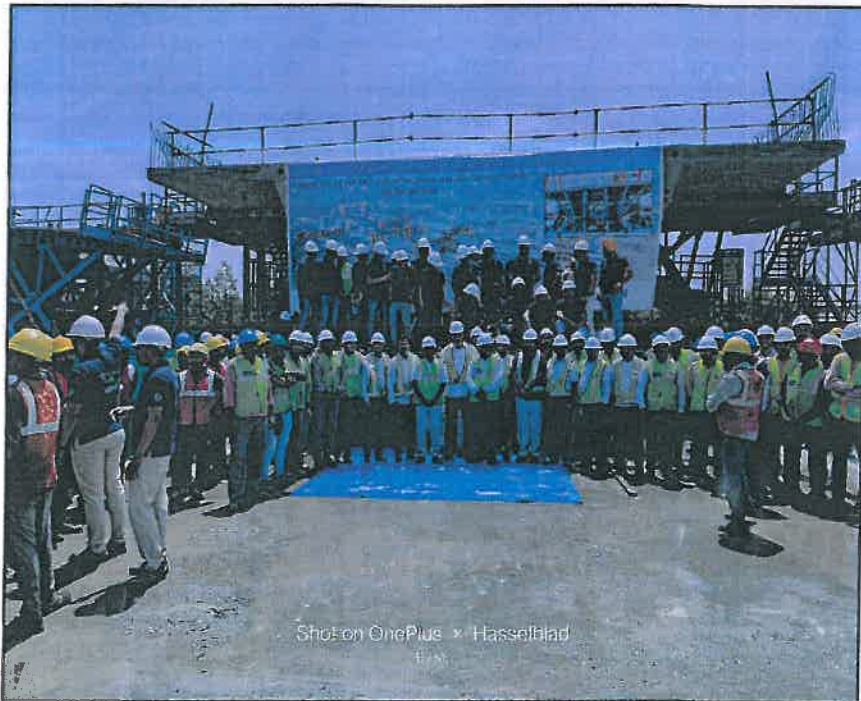
Photo no.9 Casting of Last Segment at Precast yard
