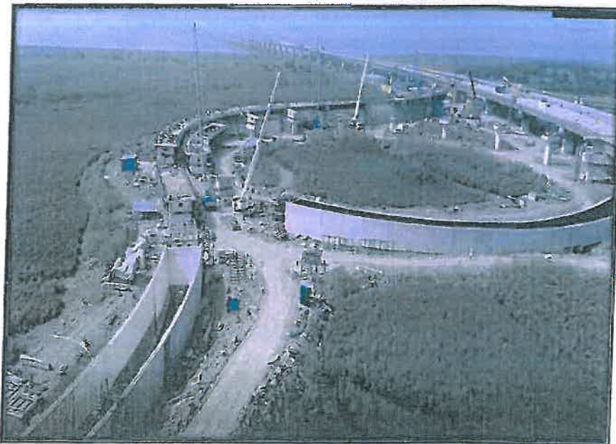
Package-2 Aerial View
