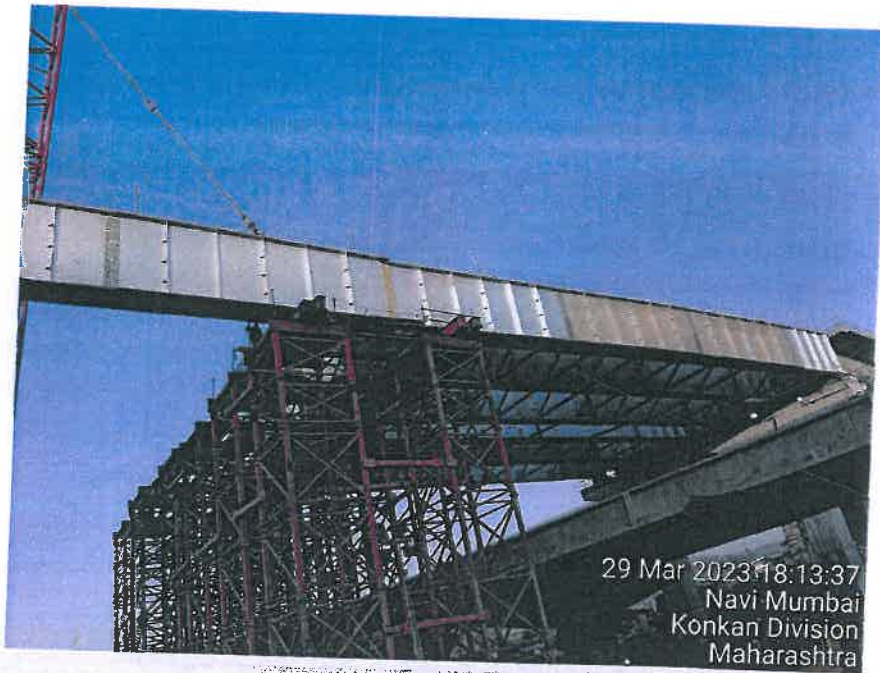
Photo no.5- Steel girder erection work at Jasai SH-54 span RP 19-20.
