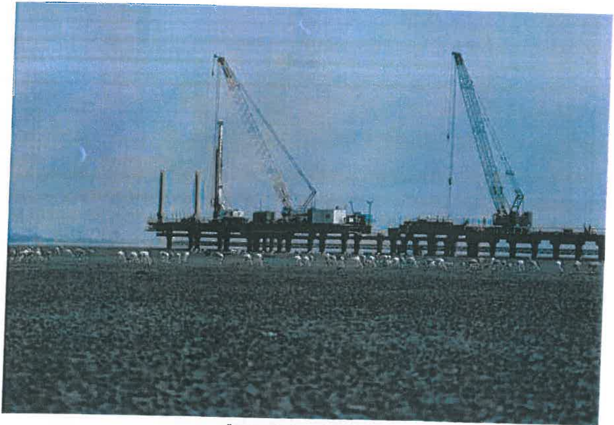
Sewri Construction site
