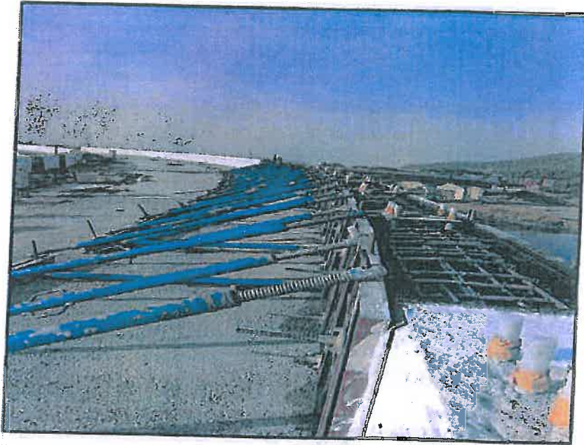
Photo no.1- Chirle Ramp PMP outer crash barrier shuttering work.
