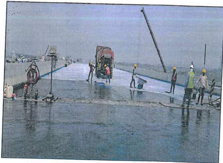
Photo no.6- Application of Tack coat in progress at LHS Carriageway.
