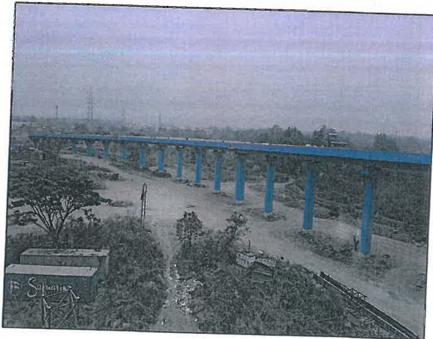
Photo no.6- Anti carbonation paint work at Chirle Ramp JMP.
