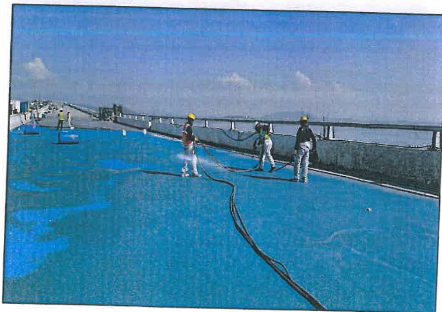
Photo no.2 Water proffing membrane at Ch.2530
