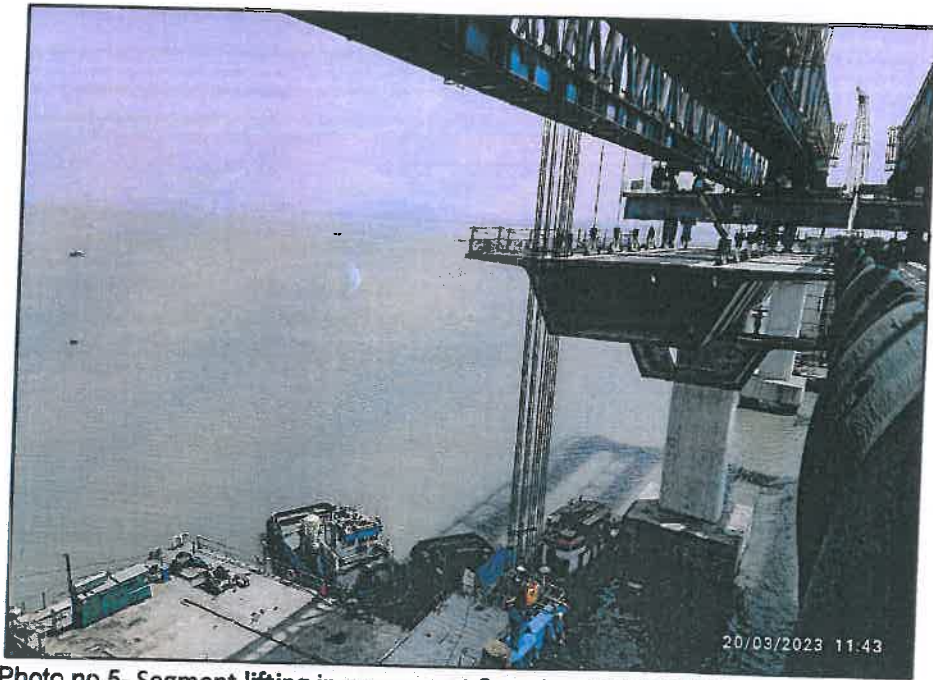
Photo no.5- Segment lifting in progress at Span MP 164-165 LHS.
