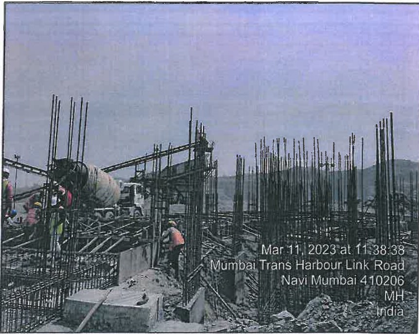
Photo no.1- Plinth beam reinforcement and Shuttering work is in progress
