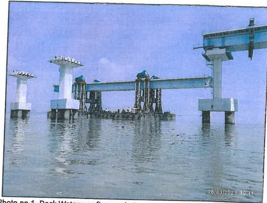
Photo no.1- Deck Waterproofing works in progress at LHS Carriageway.
