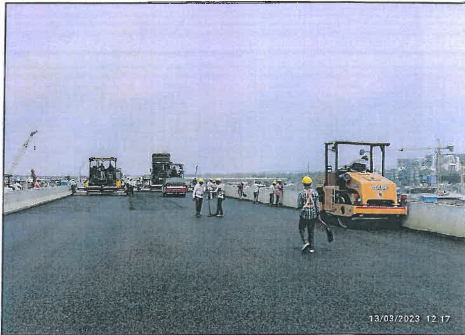
Photo no.7- SMA laying in progress at LHS Carriageway.
