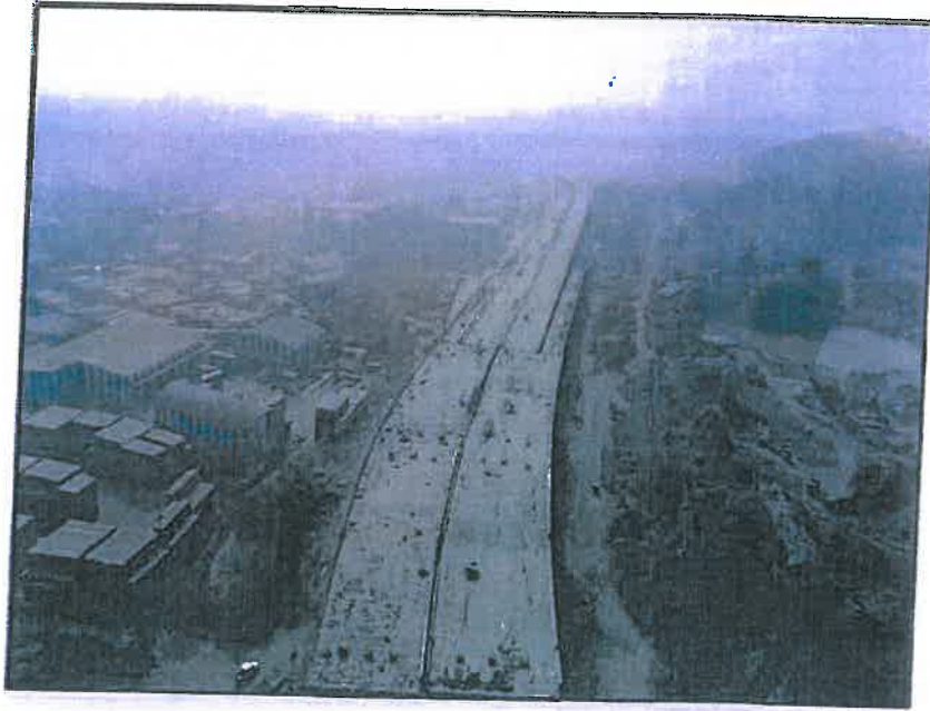
Photo no.5- Jasai Viaduct.
