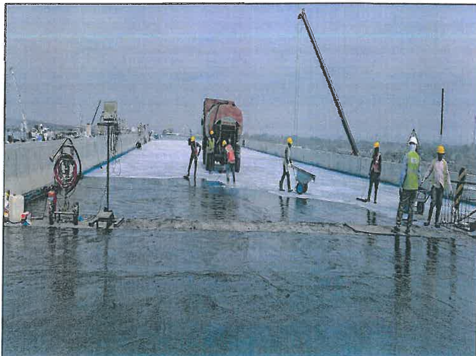
Photo no.7- SMA laying in progress at LHS Carriageway.
